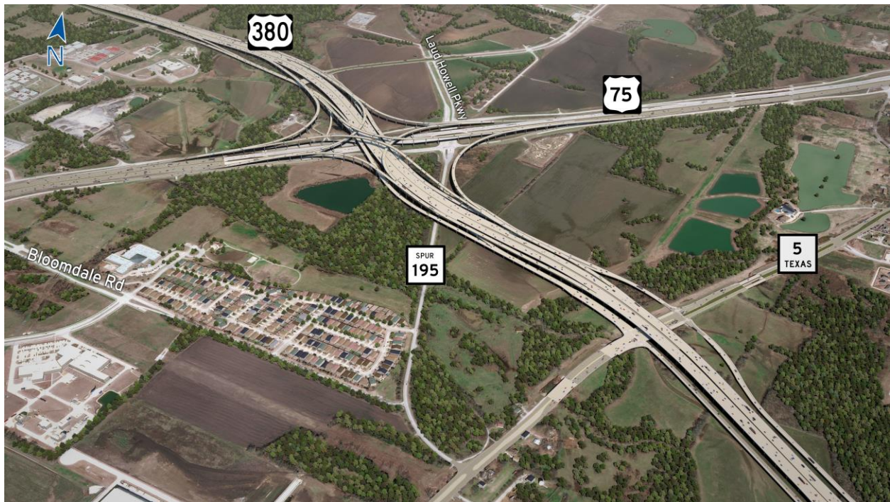
Figure 3-35: Multi-level Interchange at US 75 and Connection to SH 5, Looking Northwest – Segment E
