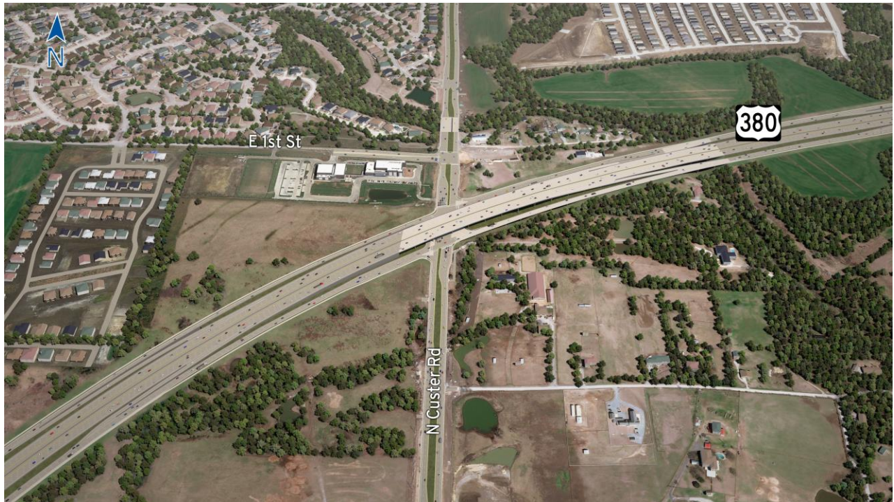
Figure 3-33: View of Elevated Section and Intersection at N. Custer Road – Segment B
