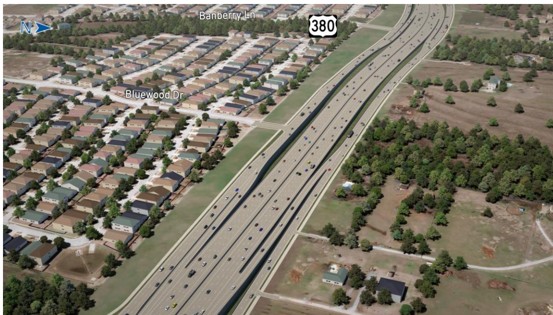
Figure 3-34: View of Elevated Section Near Heatherwood, Looking West - Segment E
