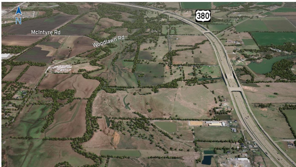
Figure 3-36: View Near CR 331/Woodlawn Road, Looking North – Segment C
