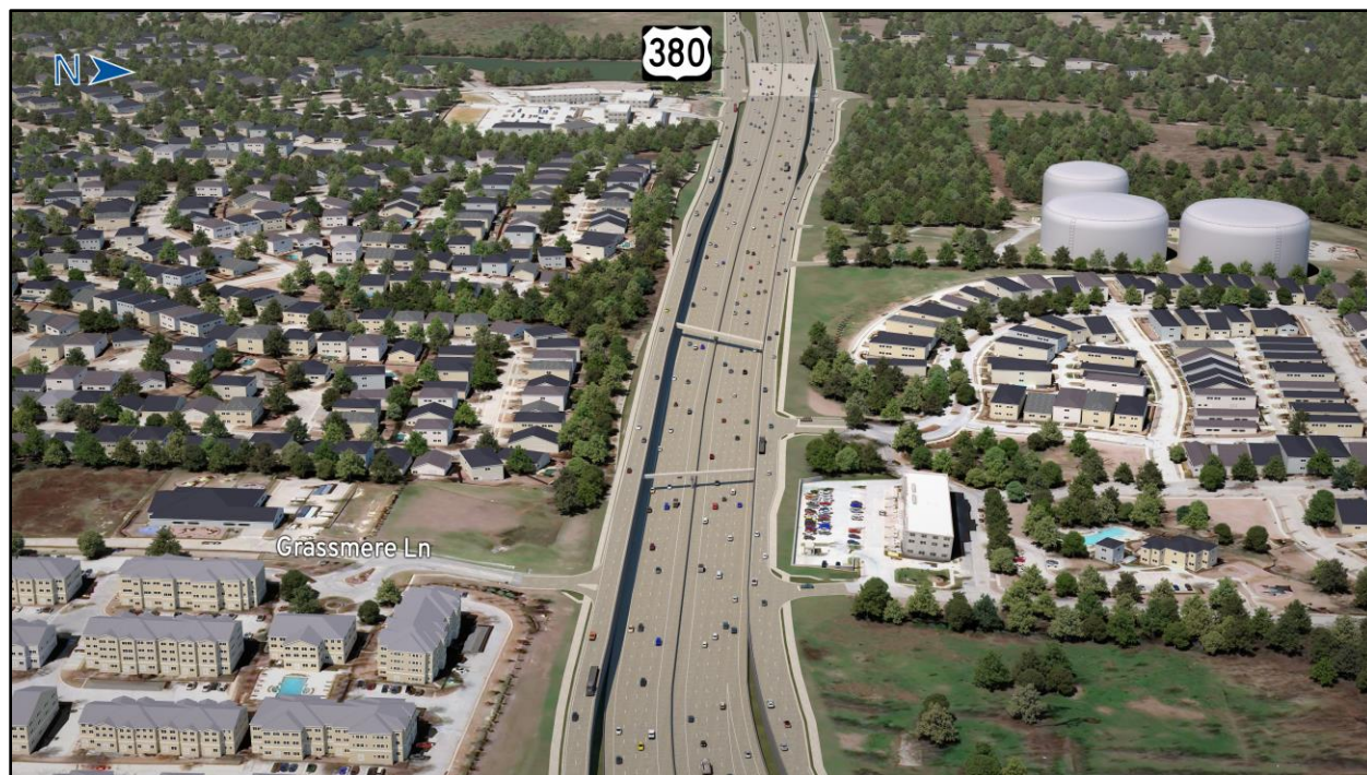
Figure 3-32: View Looking West Along the Depressed Section Between Tucker Hill (right) and Stonebridge Ranch (left) - Segment A
