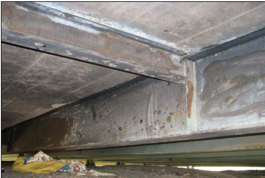
23. Looking west at a slight deflection of beam 2 (span 5) of the IH 30 eastbound bridge. The damage was caused by camp fires.
