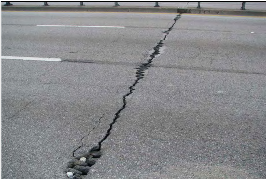
27. Looking southeast at the minor longitudinal and transversal cracking of the IH 30 westbound bridge pavement over an expansion joint.
