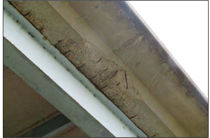
26. Looking south at the IH 30 westbound bridge spalling with exposed steel in soffit at the north deck overhang.
