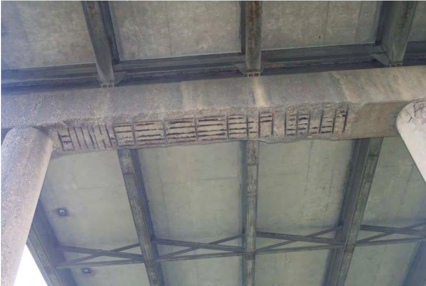
17. Looking southwest at the caps of bents 7 and 21 of the IH 35E southbound bridge which have widespread moderate spalls and exposed rebar.
