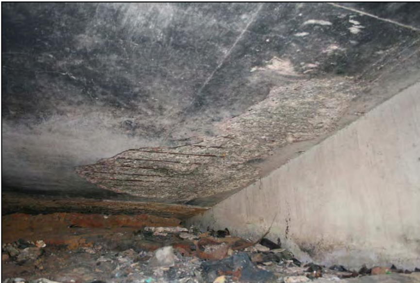
15. Looking northwest at the spalled underside deck of the IH 35E southbound bridge located at the northeast corner of span 40. The deck has moderate fire damage over a 6-ft by 10-ft area of slab and exposed rebar.
