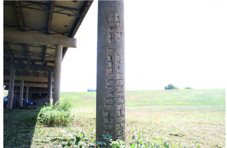
18. Looking southwest at the IH 35E southbound bridge column for bent 43. The column exhibits moderate cracks and spalls with exposed rebar.
