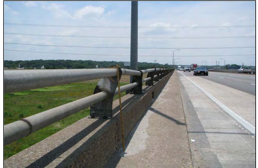
22. Looking southwest at an IH 30 eastbound bridge rail previously repaired. The rail height is uneven because of the retrofit steel pedestal utilized.
