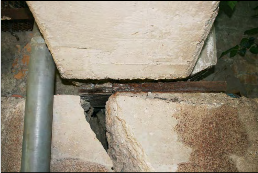
13. Northeast at the bearing area for the east exterior sidewalk beam at the north abutment of the IH 35E northbound bridge. The bearing area has been reduced by approximately 6 inches due to cracking of the abutment cap.
