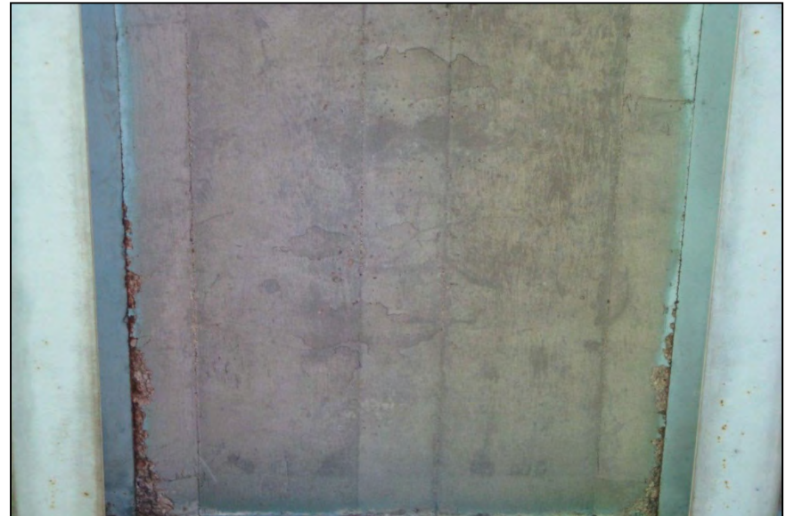
20. Looking southwest at map cracking and spalling along the beam in the deck soffit of the IH 30 eastbound bridge.
