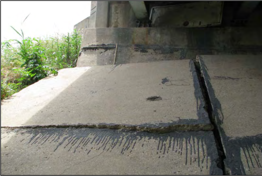
25. Looking southwest at the IH 30 eastbound bridge south end of the west riprap which has settled and cracked due to erosion/undermining of the Trinity River west embankment.
