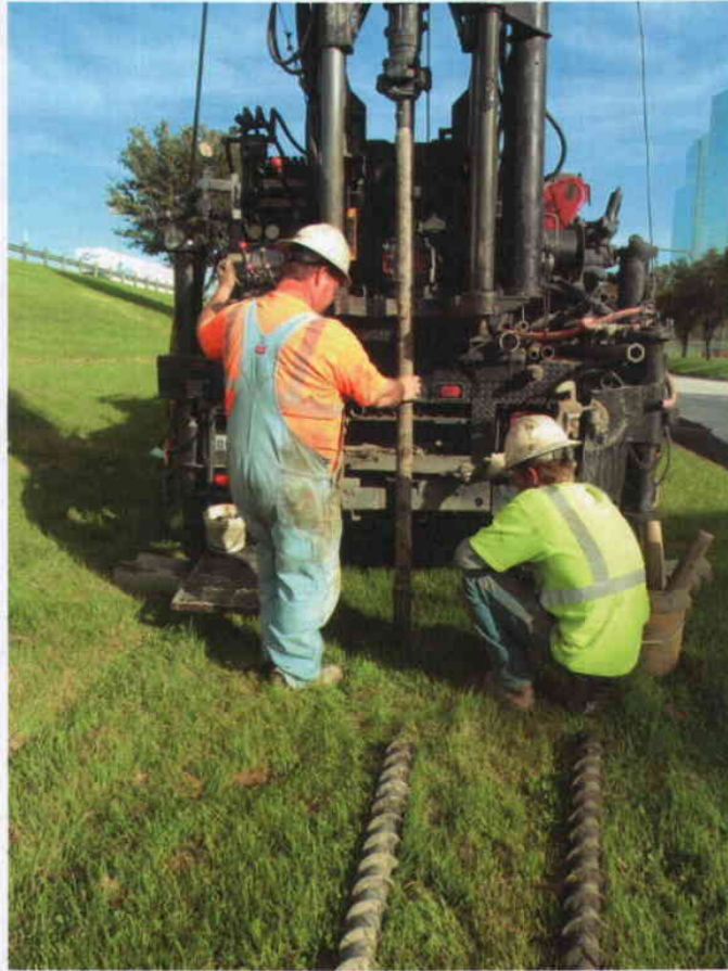
Photo 1. Collection of core sample P-14.
