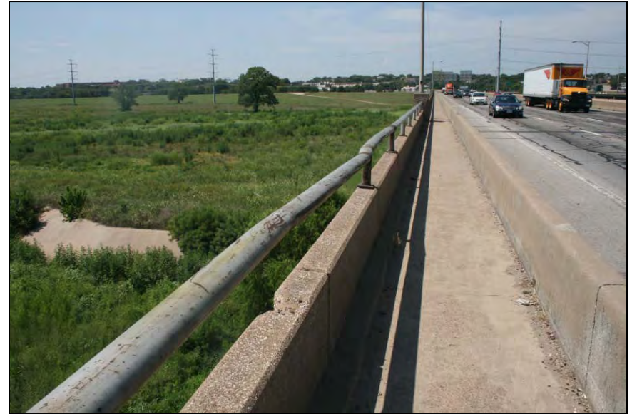
14. Looking north at the damaged railing along the IH 35E northbound bridge. The horizontal rail pipe along the east side of the pedestrian railing has moderate collision damage. Additionally, the horizontal rail is bent and one post is missing.
