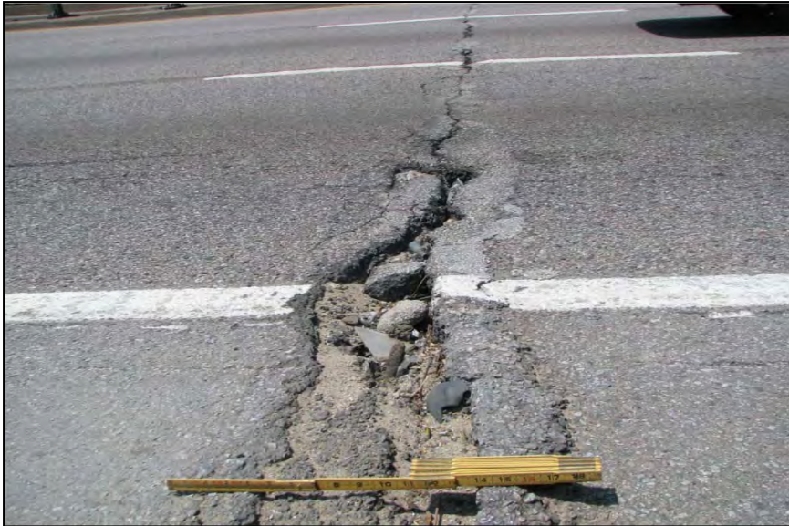
21. Looking northwest at the spalling and roughness of asphaltic pavement at the joint over bent 13 of the IH 30 eastbound bridge.
