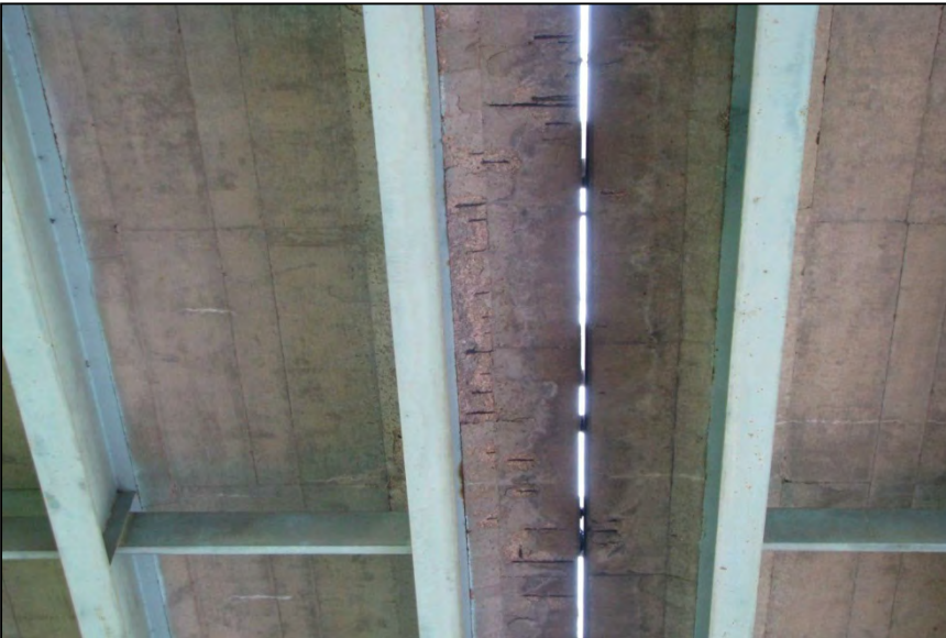
19. Looking southwest at the moderate spalling with exposed steel at the north deck overhang of the IH 30 eastbound bridge. There is also minor transversal cracking with efflorescence in the deck soffit.
