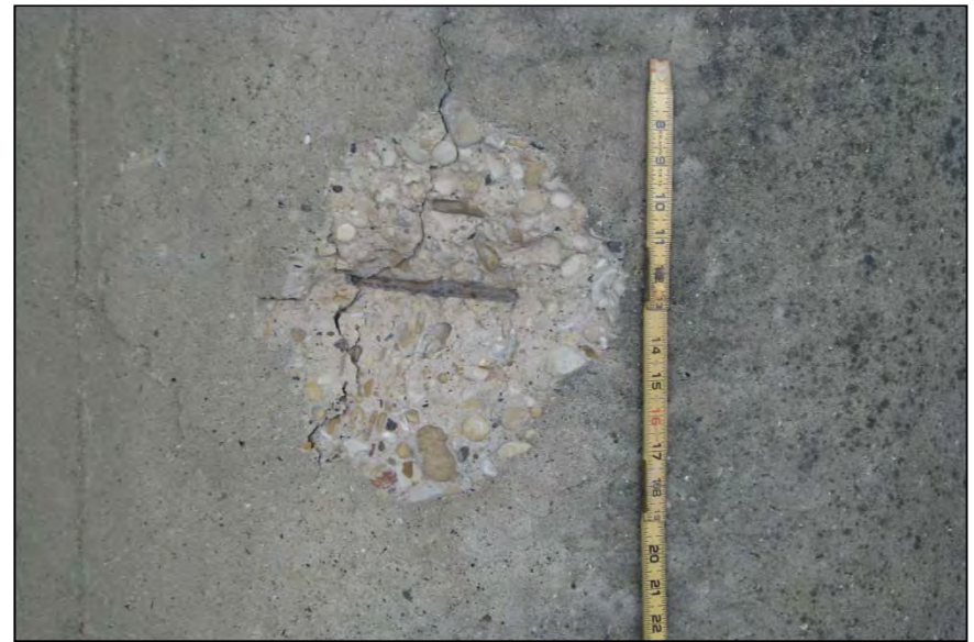
28. Looking northwest at minor spalling and exposed steel on column 3 of bent 13 of the IH 30 westbound bridge.
