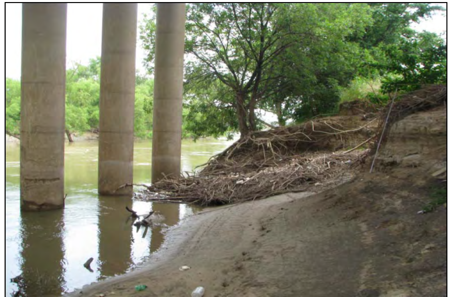
24. Looking southwest at moderate erosion of the west channel bank of the Trinity River and drift at the IH 30 eastbound bridge (bent 19).
