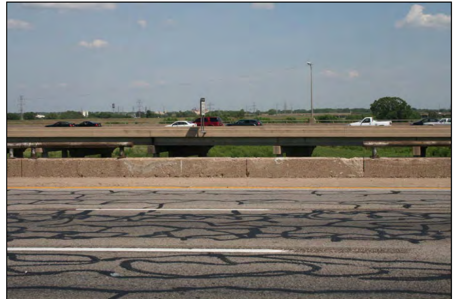
16. Looking southeast at the east side of the IH 35E southbound bridge for which four sections of horizontal rail pipe are missing.
