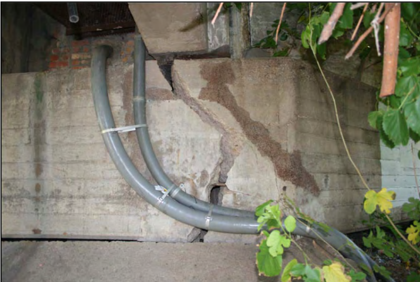
11. Looking northeast at the IH 35E northbound bridge north abutment cap that exhibits a large crack variable in width from 5 inches at the top of the cap to 4.5 inches at the bottom of the cap.
