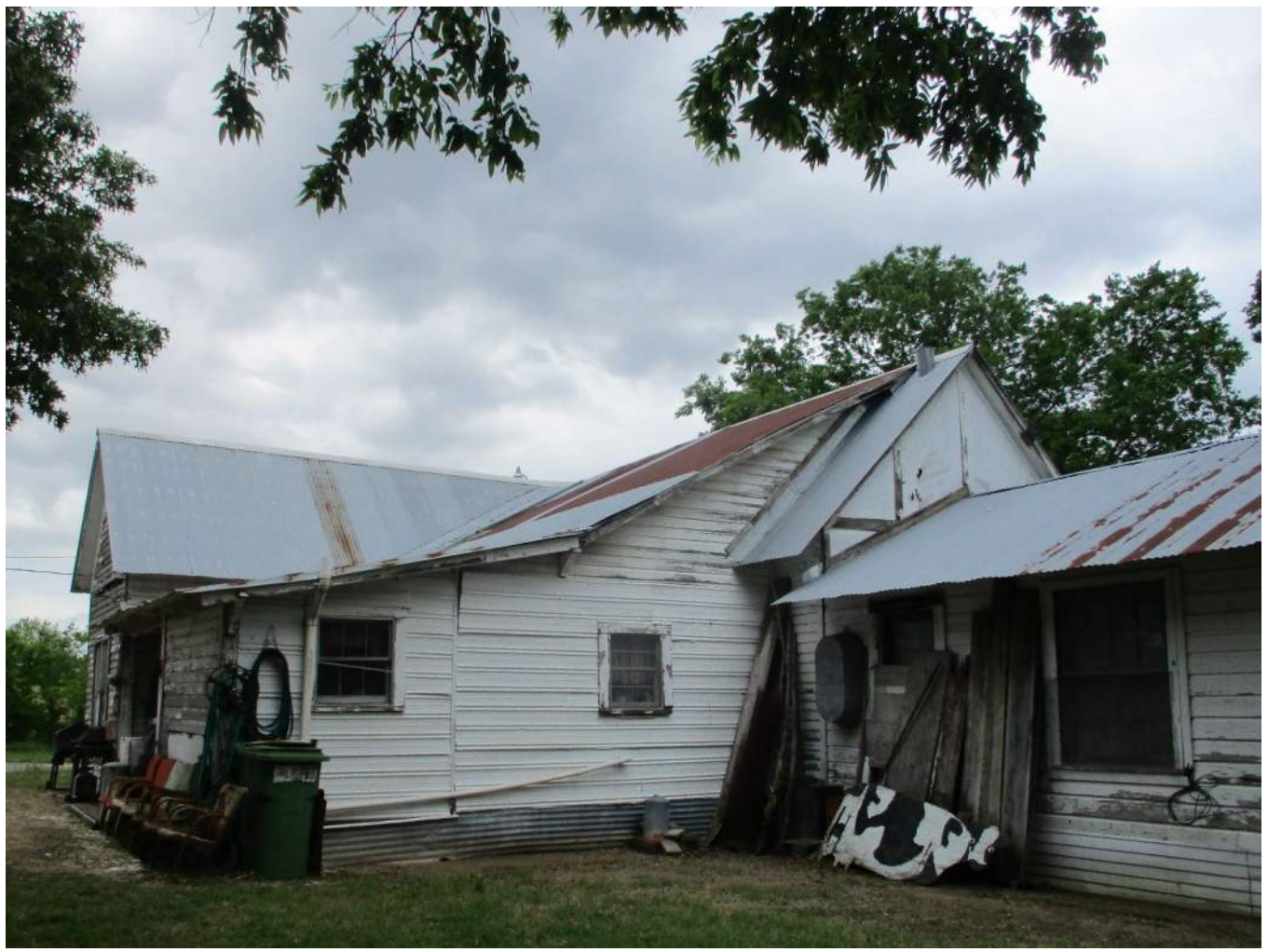
Resource 01a western elevation, facing southeast.
