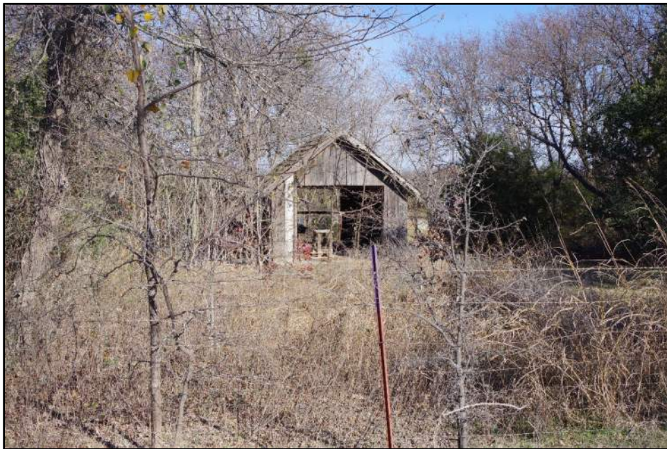
Photograph F-112: View of Resource 23g, camera facing north.
