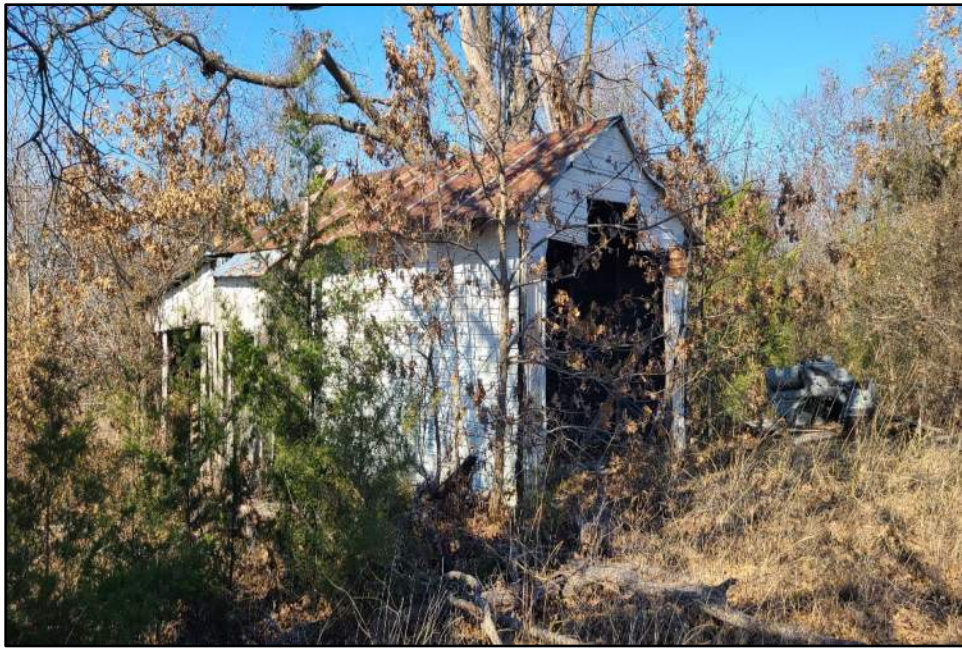
Photograph F-357: Obstructed view of Resource 78d, camera facing northeast.
