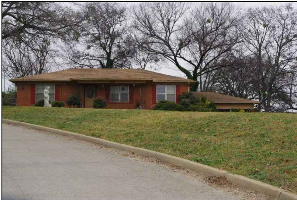
View of Resource 101a, camera facing northwest.
