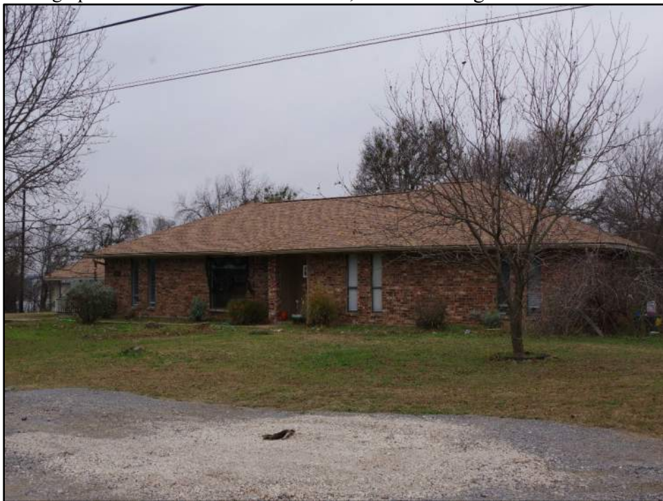
Photograph F-392: View of Resource 88, camera facing southwest.
