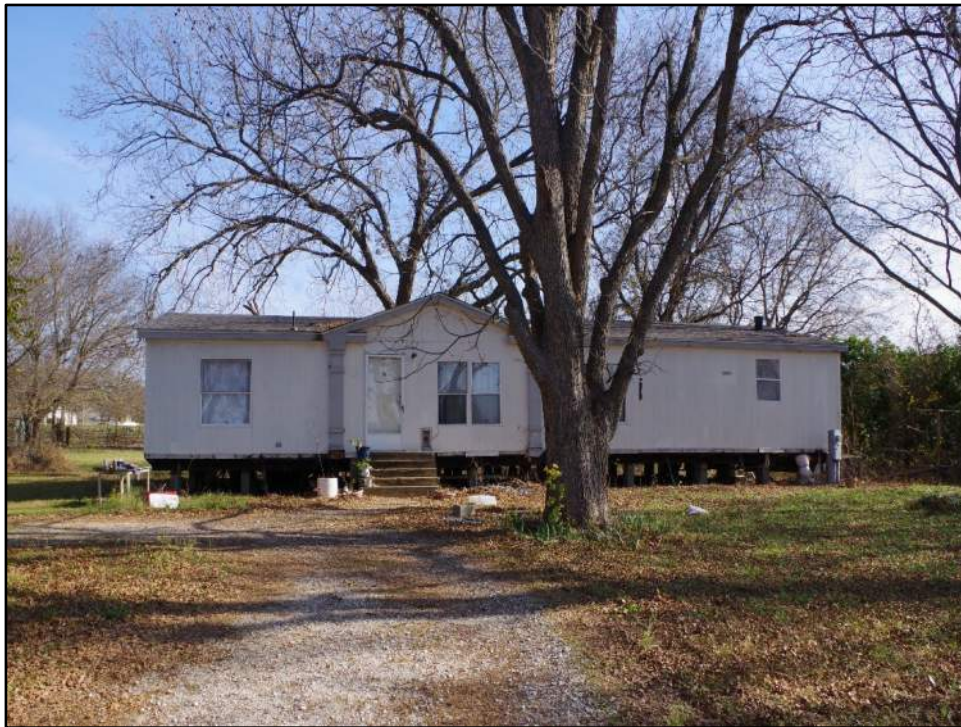
View of Resource 65, camera facing east.
