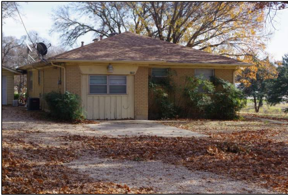
Photograph F-149: View of Resource 31a, camera facing east.
