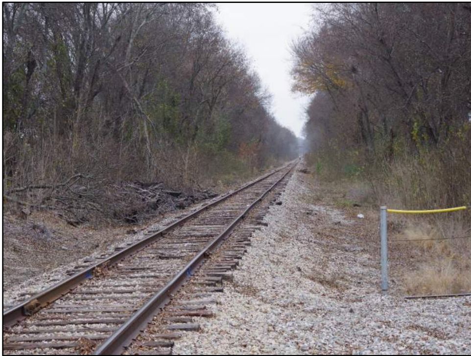
Photograph F-173: View of Resource 35a, camera facing north.
