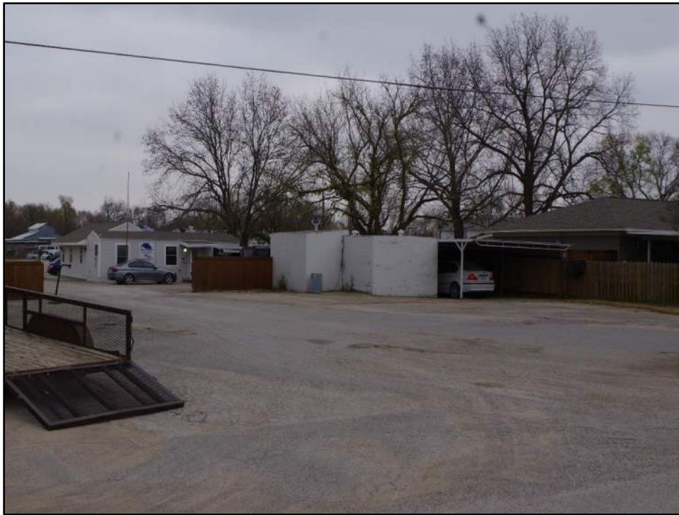
Photograph F-189: View of Resource 39a (rear) and Resource 39b (foreground), camera facing southeast.
