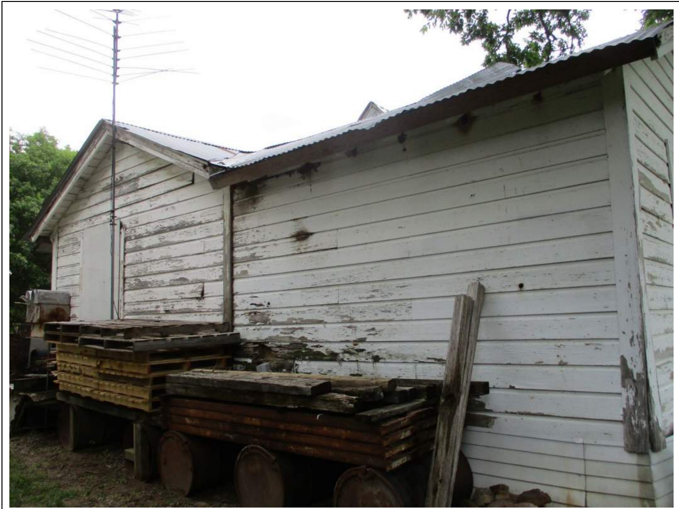
Resource 01a western addition elevation, facing southeast.
