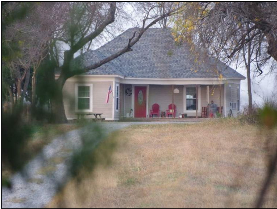
Photograph F-247: View of Resource 53a, camera facing north.
