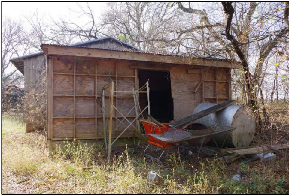
Photograph F-109: View of Resource 23e, camera facing south.
