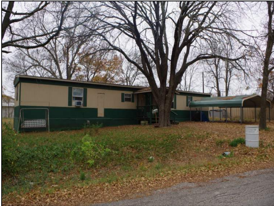
Photograph F-420: View of Resource 96, camera facing southwest.
