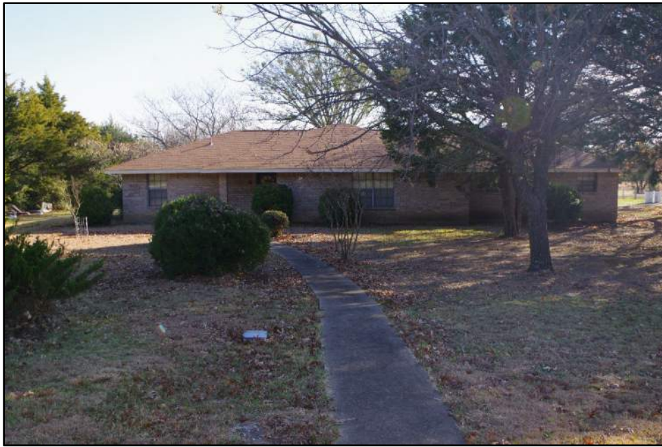
Photograph F-67: View of Resource 19a, camera facing east.
