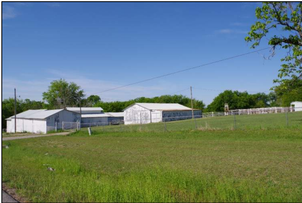
Photograph 22: View of non-historic-age outbuildings on County Road 332 (CR 332), camera facing southwest.
