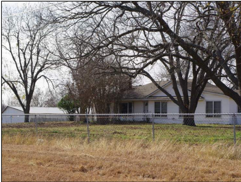
View of Resource 58a, camera facing southwest.
