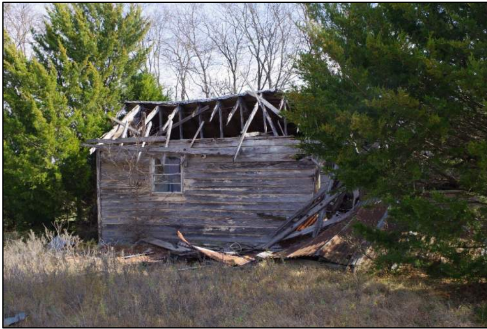
Photograph F-121: View of Resource 25b, camera facing east.
