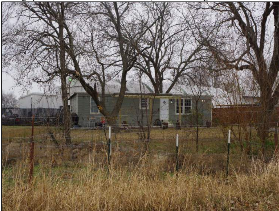
Photograph F-186: View of Resource 38b, camera facing southeast.
