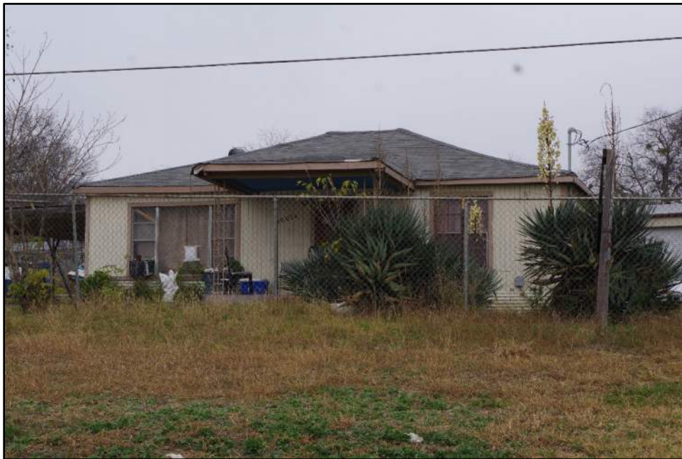
Photograph F-436: View of Resource 99a, camera facing north.
