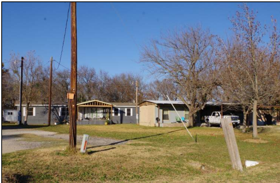
Photograph F-14: Overview of Resource 05, camera facing northeast.
