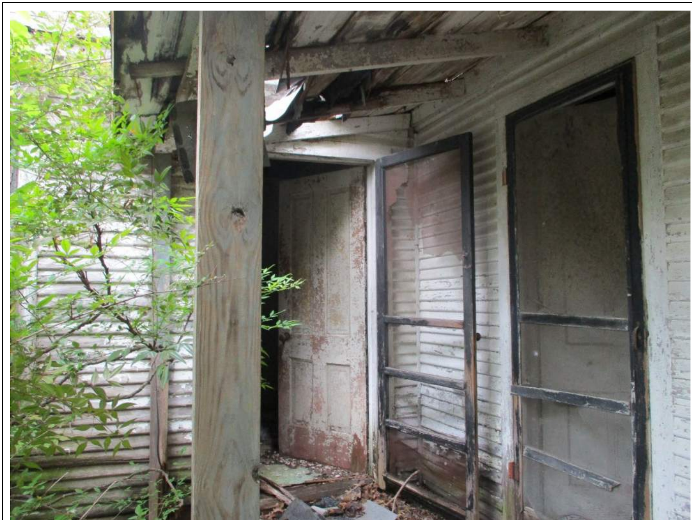
Resource 01b southern elevation and front ell, facing northwest.
