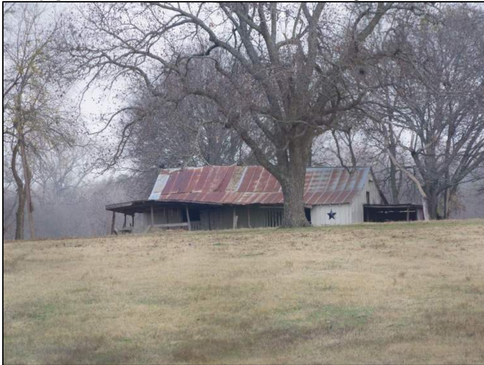
Photograph F-248: View of Resource 53b, camera facing north.
