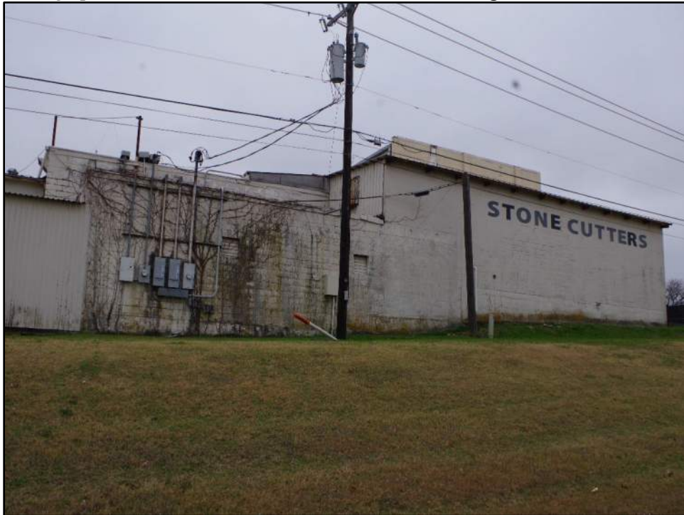
Photograph F-224: View of Resource 48, camera facing southwest.
