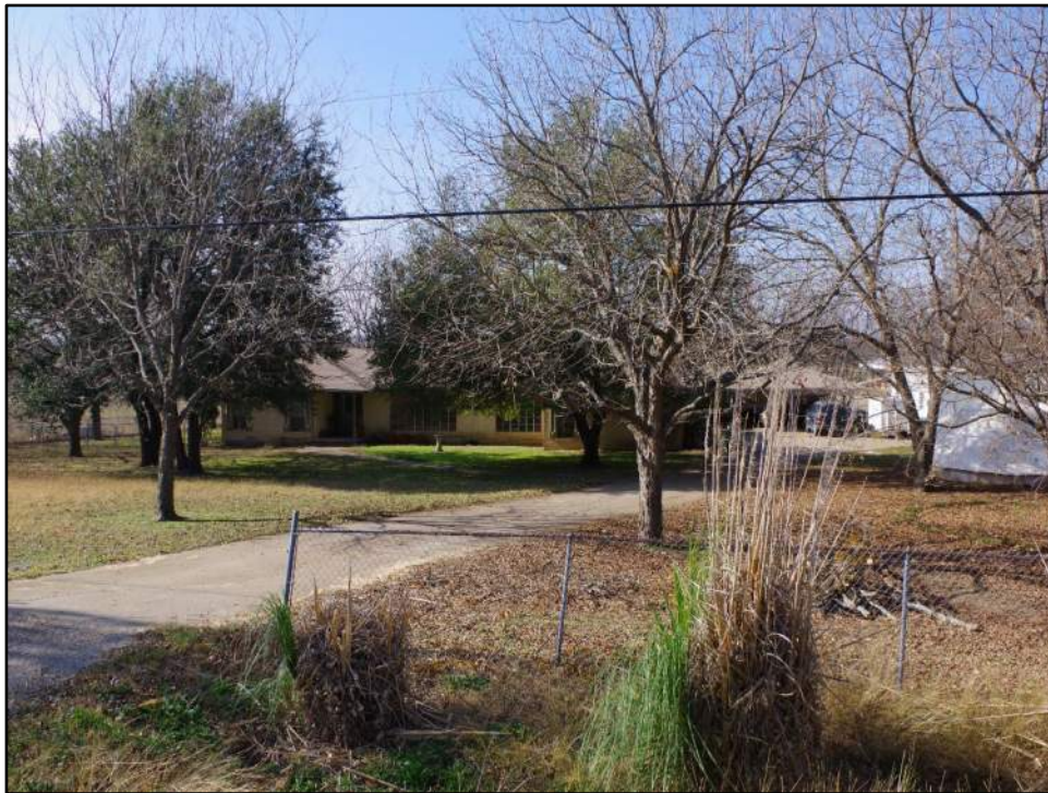
View of Resource 61a and Resource 61b (right, background), non-historic-age outbuildings, camera facing west.
