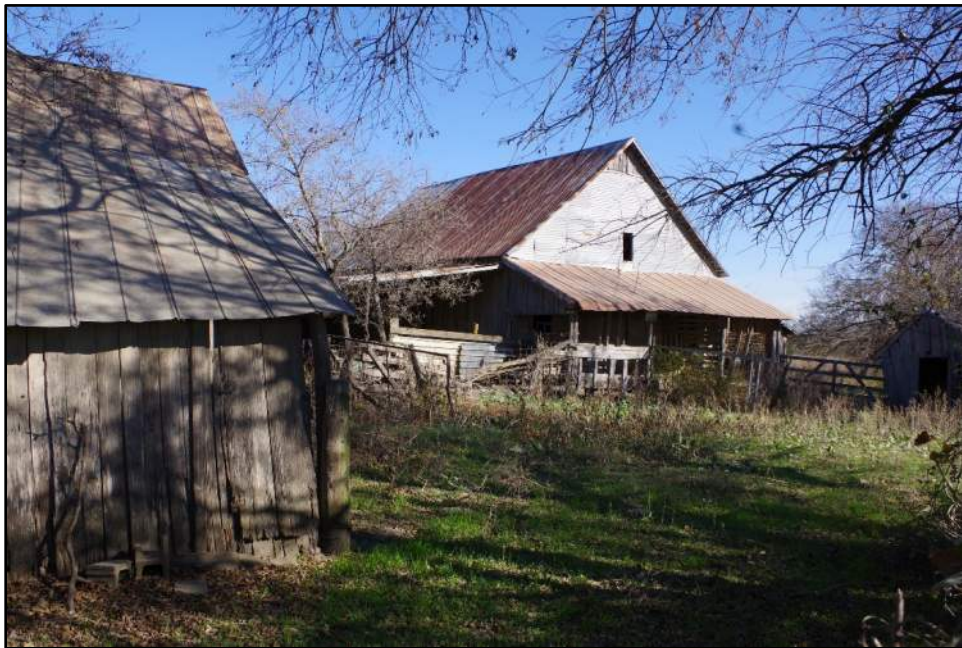
Photograph F-86: View of Resource 22b, camera facing northeast.
