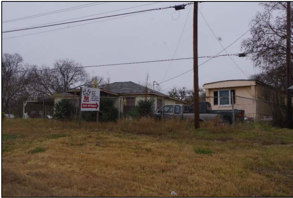
Photograph F-435: Overview of Resource 99, camera facing northwest.
