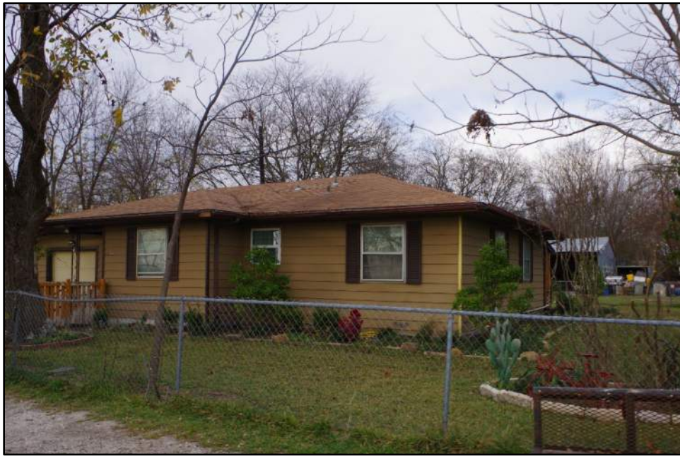
Photograph F-333: Overview of Resource 72, camera facing northwest.
