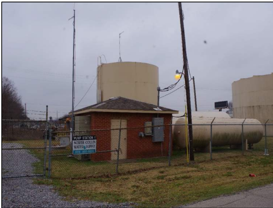
View of Resource 90a and Resource 90b (rear), camera facing southwest.
