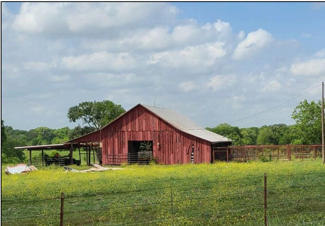
Photograph 8: View of 3187 FM 2933 barn, camera facing north (April 2023).
