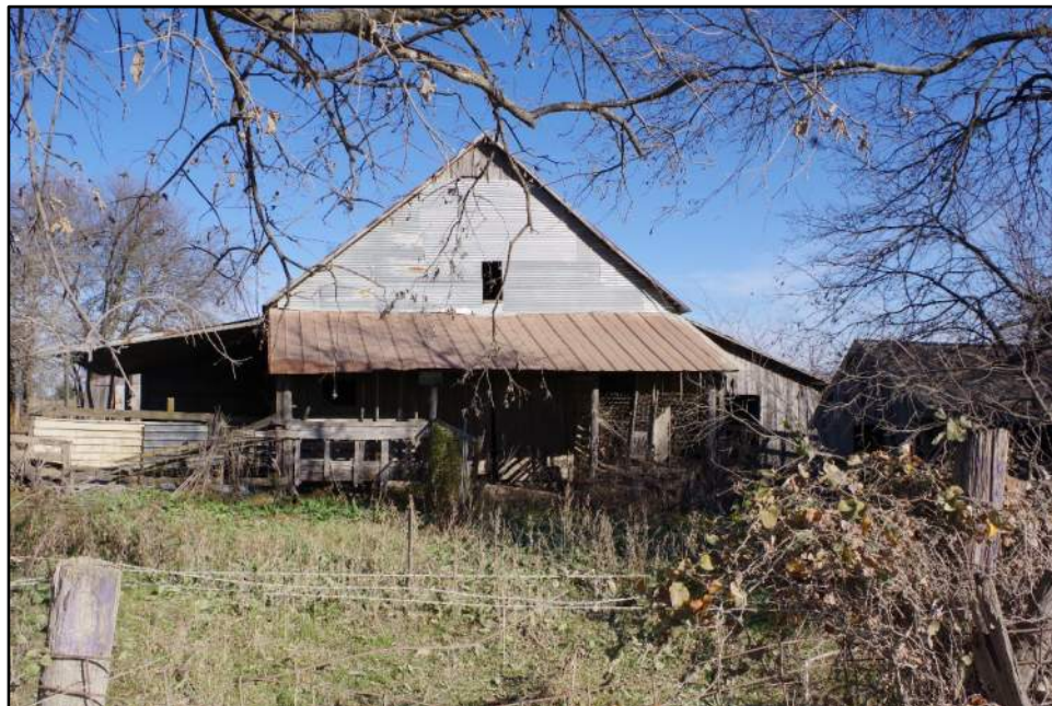
View of Resource 22b, camera facing north.
