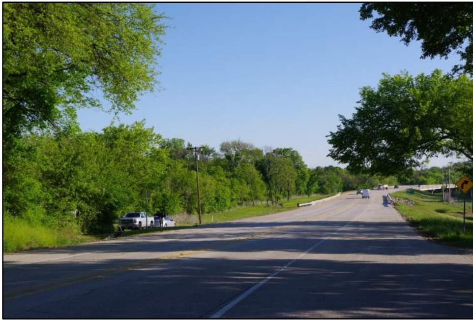
Photograph 55: View of existing ROW on North McDonald Street, camera facing northeast.
