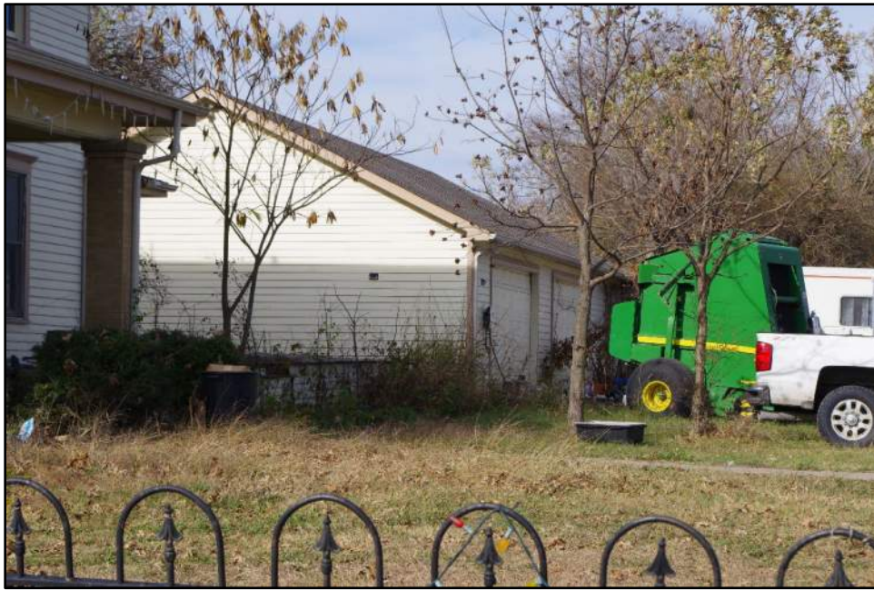
Photograph F-169: View of non-historic-age garage associated with Resource 34, camera facing north.
