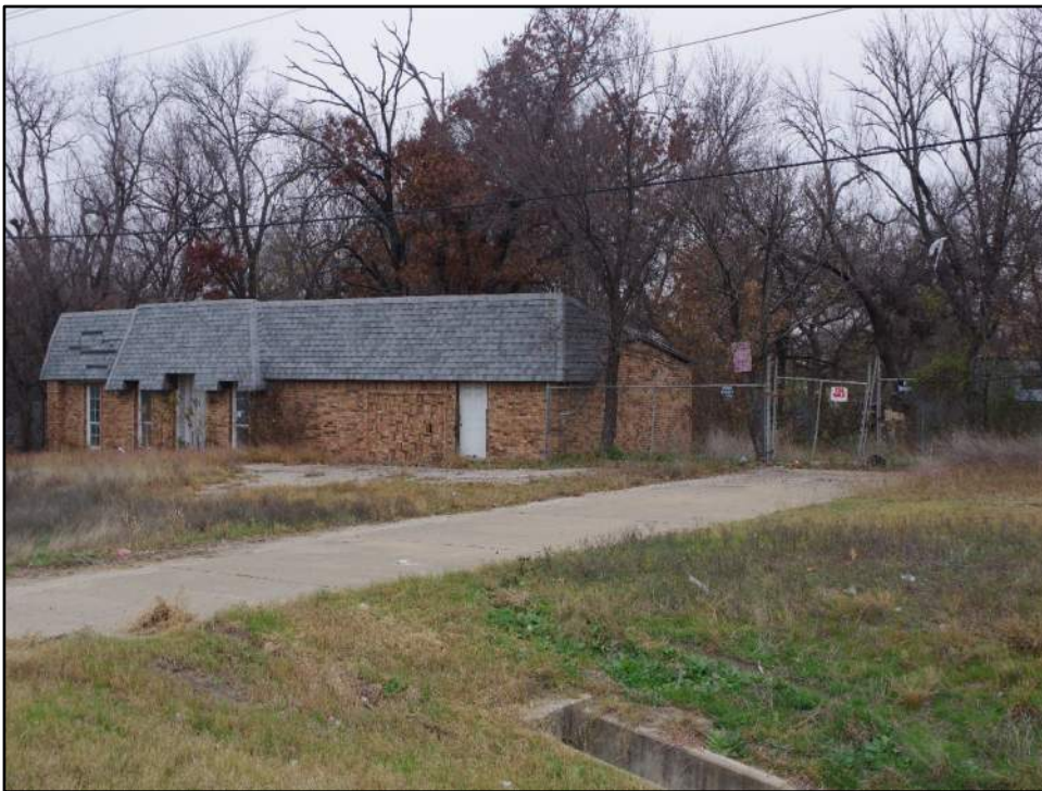
View of Resource 83, abandoned, camera facing northwest.
