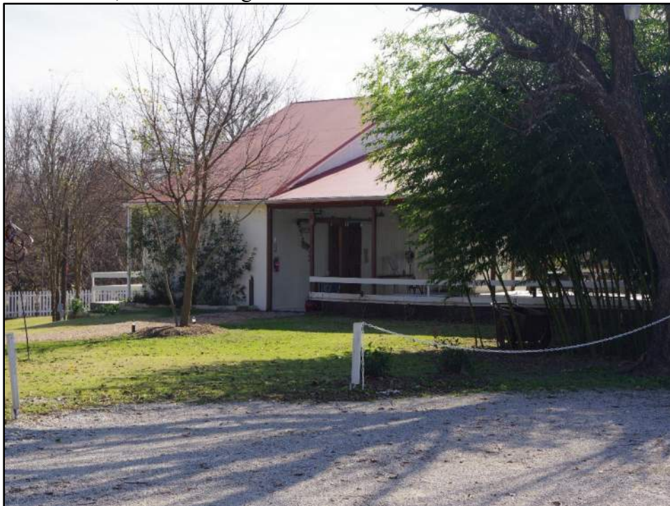
Photograph F-322: View of non-historic-age building associated with Resource 68, camera facing south.
