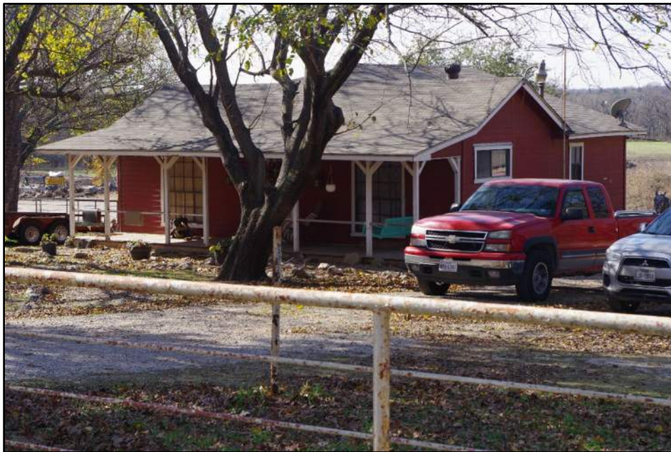
Photograph F-142: View of Resource 30b, camera facing southwest.
