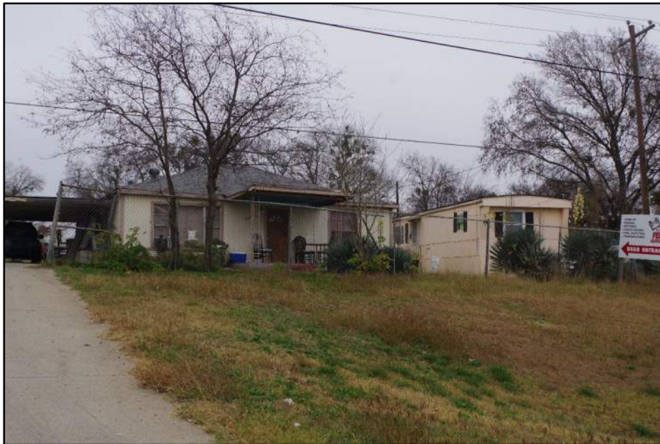
View of Resource 99a and Resource 99b, camera facing northeast.
