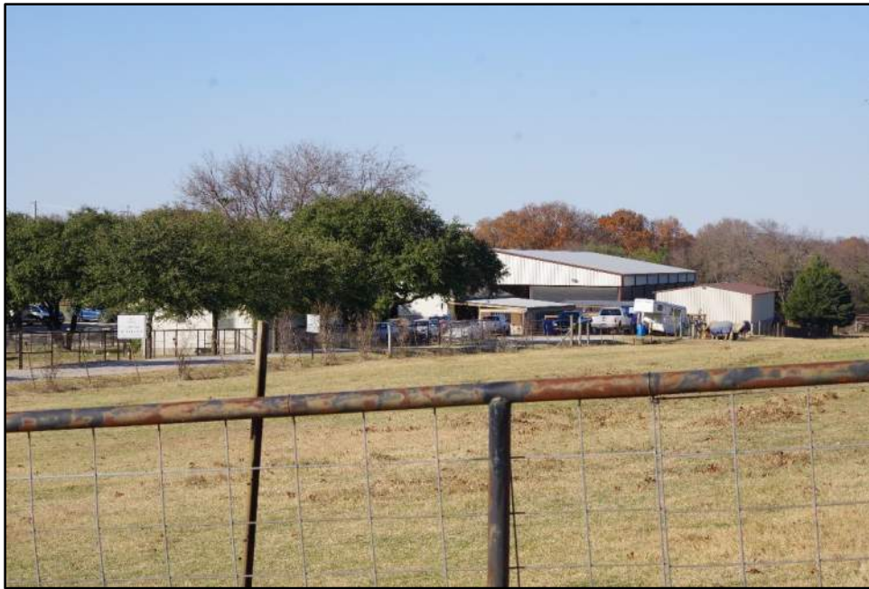
Photograph F-25: View of Resource 07c and Resource 07d (right), camera facing northwest.
