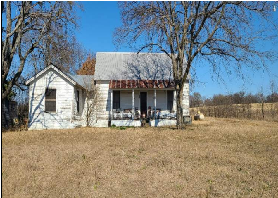
Photograph F-348: View of Resource 78a, camera facing north.
