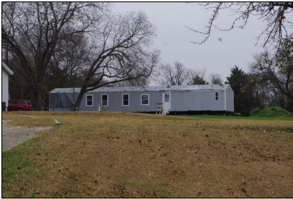
View of Resource 97c, camera facing northwest.
