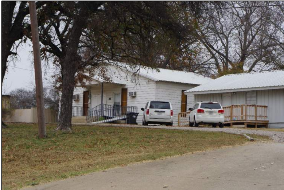
Obstructed view of Resource 97a, camera facing northwest.
