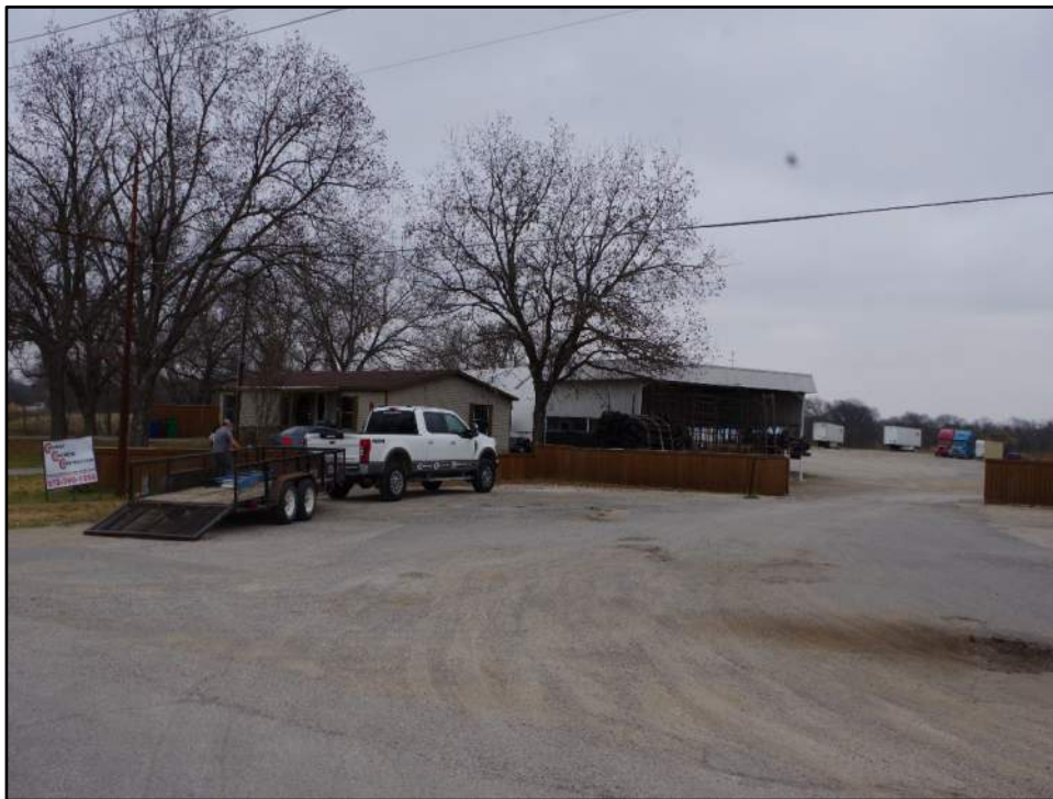
View of Resource 39c (right), camera facing northeast.
