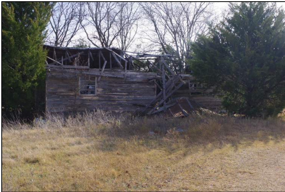
Photograph F-122: View of Resource 25b, camera facing southeast.
