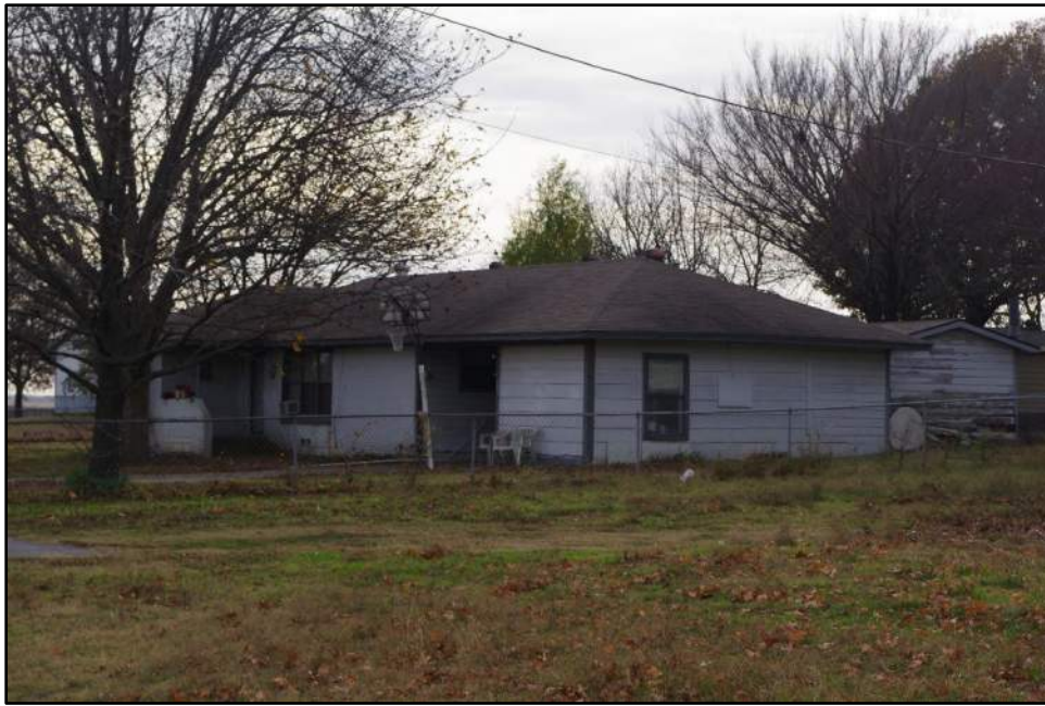
Photograph F-339: View of Resource 74, camera facing southwest.
