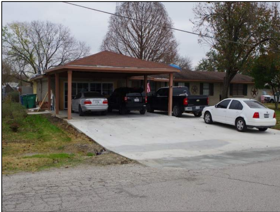
View of Resource 42, camera facing east.
