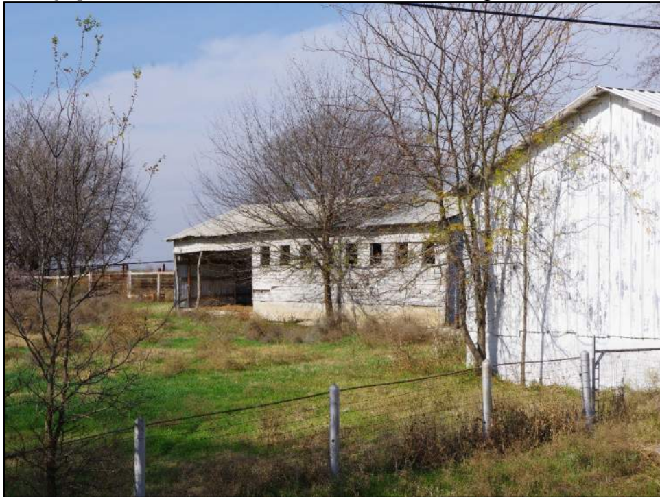
Photograph F-290: View of Resource 58e, camera facing northwest.
