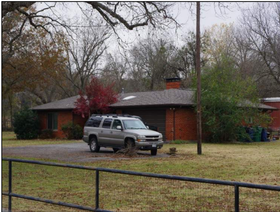
View of Resource 44a, camera facing southwest.
