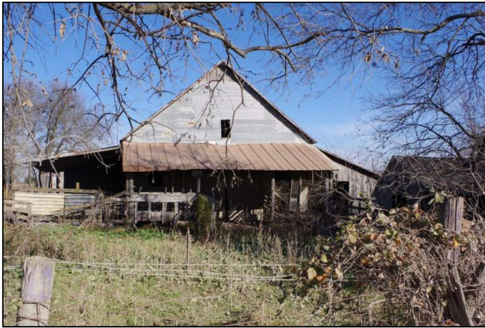
Photograph F-85: View of Resource 22b, camera facing north.
