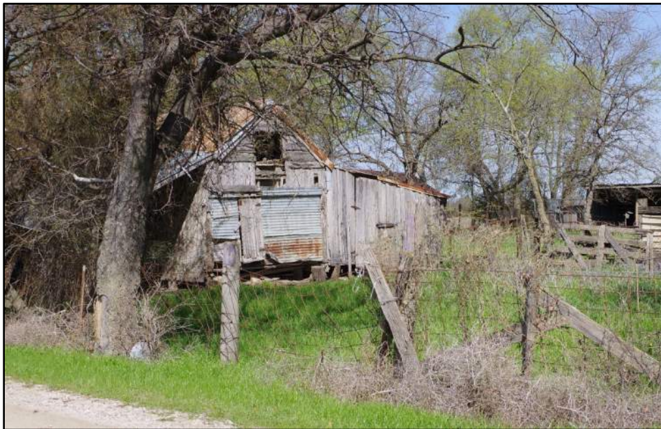
Photograph F-94: View of Resource 22h, camera facing northwest.
