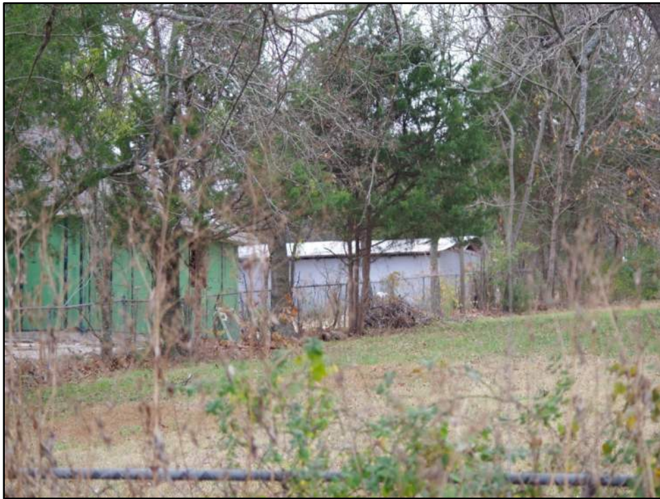
Photograph F-219: View of Resource 47, camera facing southwest.
