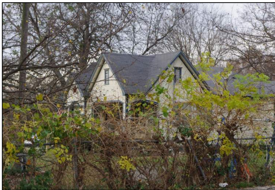
View of Resource 71a, camera facing northwest.
