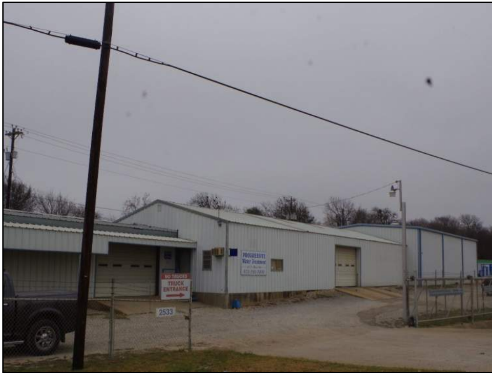
Photograph F-385: View of non-historic-age buildings associated with Resource 86, camera facing northeast.
