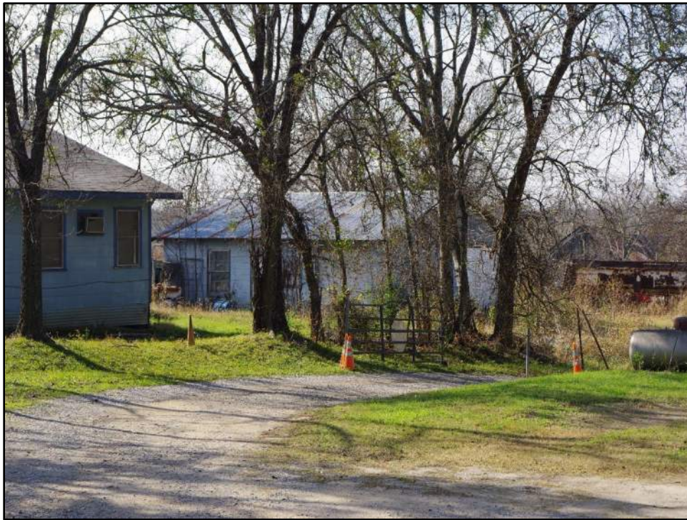
Photograph F-305: View of Resource 63b, camera facing southwest.
