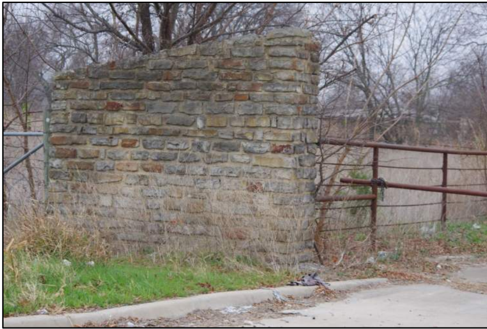
Photograph F-51: View of entrance to Resource 15, camera facing northwest.
