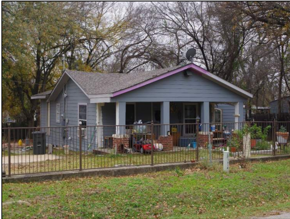
View of Resource 93a, camera facing southwest.
