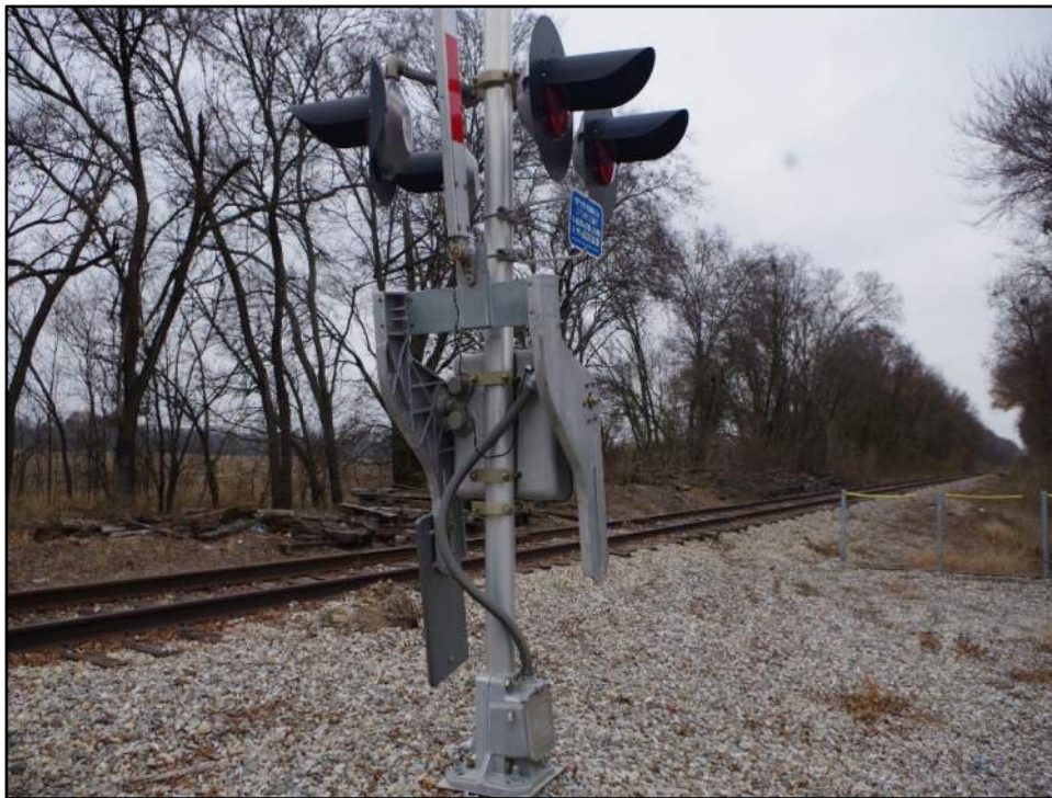
View of Resource 35a, camera facing north.
