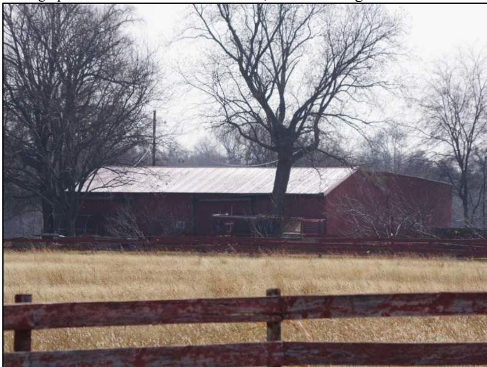
Photograph F-270: View of Resource 56b, camera facing southeast.
