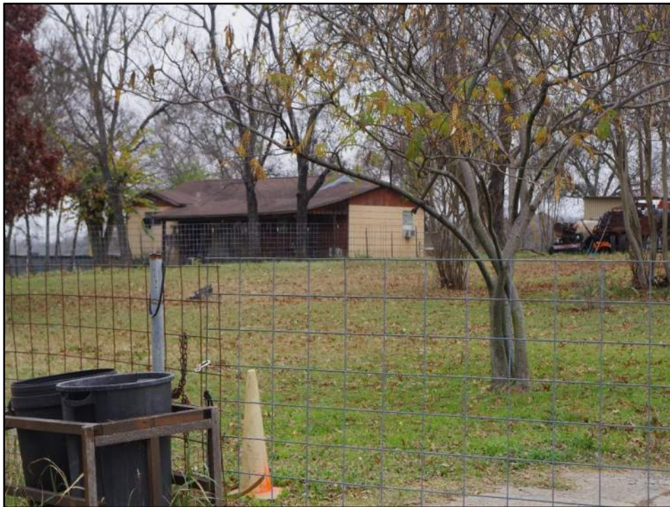
View of Resource 84a, camera facing north.
