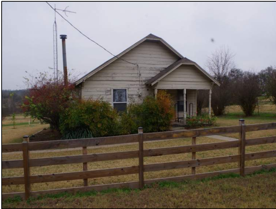
Photograph F-427: View of Resource 98a, camera facing north.
