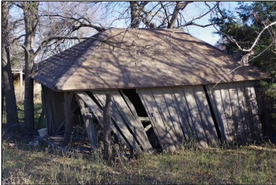
View of Resource 22i, camera facing northeast.
