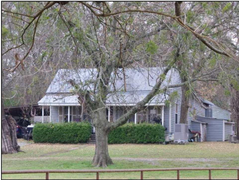
Photograph F-209: View of Resource 45, camera facing west-southwest.
