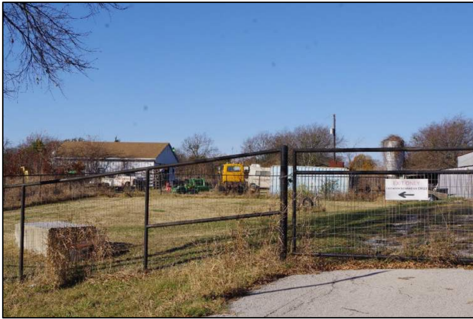
Photograph F-77: View of Resource 20b (right) and non-historic-age shed (left), camera facing west.
