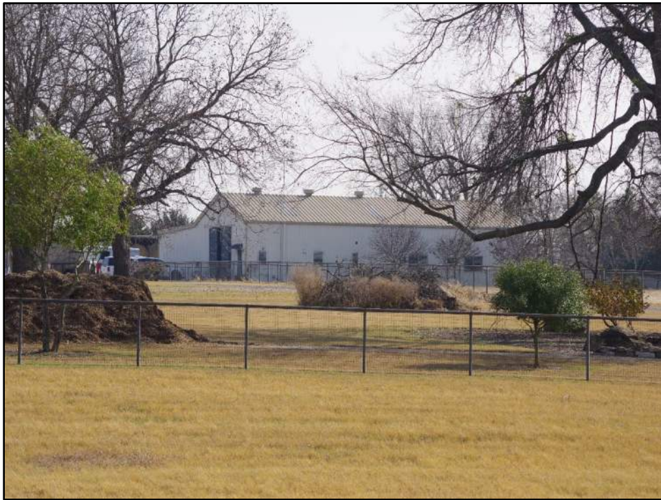
Photograph F-261: View of Resource 55a, camera facing east-southeast.
