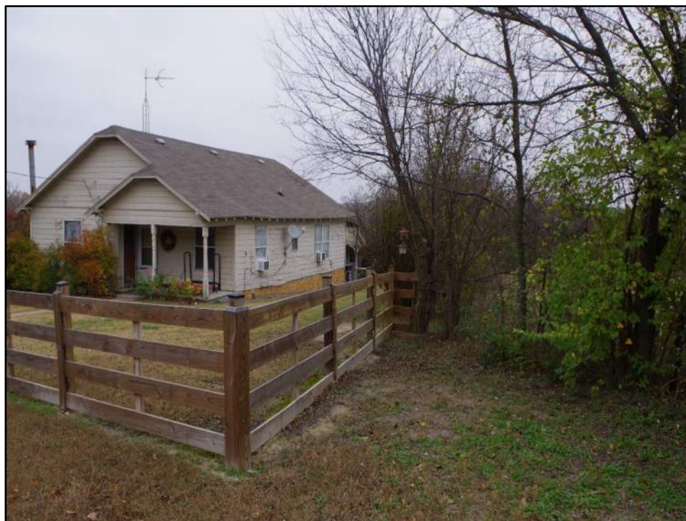
View of Resource 98a, camera facing northeast.
