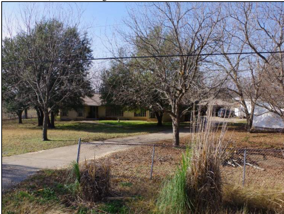
Photograph F-298: View of Resource 61a, obstructed view of Resource 61b (right, background), and non-historic-age outbuildings, camera facing west.
