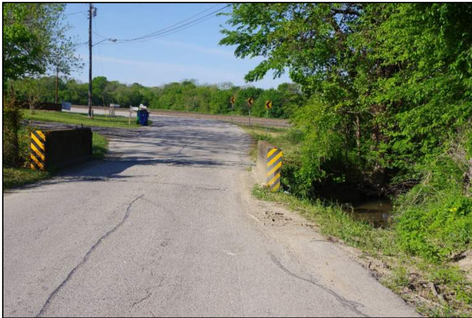
Photograph 32: View of bridge/culvert on Woodlawn Road, camera facing south-southwest.
