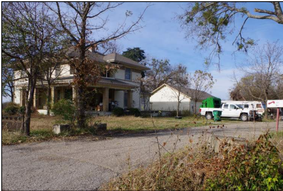
Photograph F-162: Overview of Resource 34, camera facing northwest.
