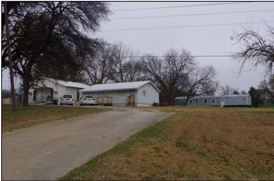
Photograph F-421: Overview of Resource 97, camera facing northwest.
