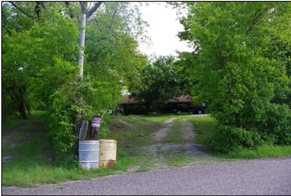
Photograph 4: View of historic-age dwelling on CR 1124, camera facing southeast.
