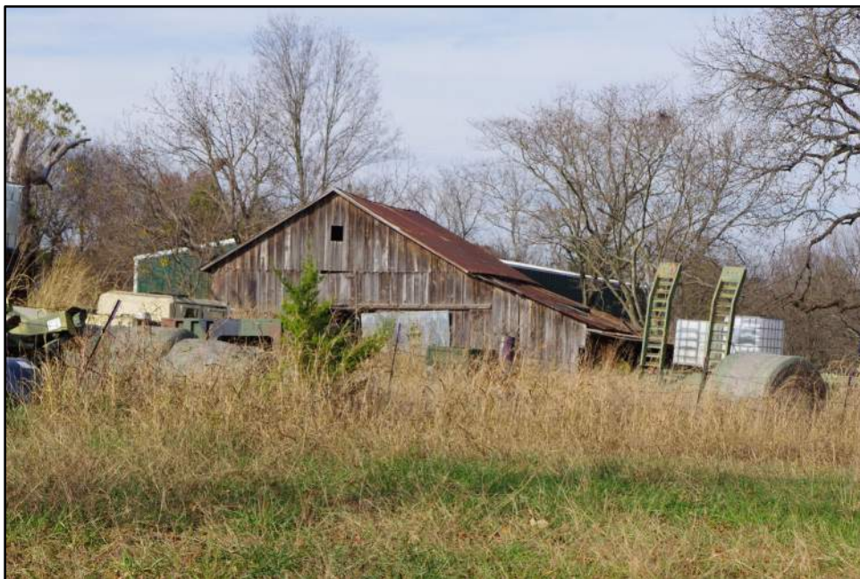
Photograph 4: View of barn on property at 551 McIntyre Road, camera facing north.
