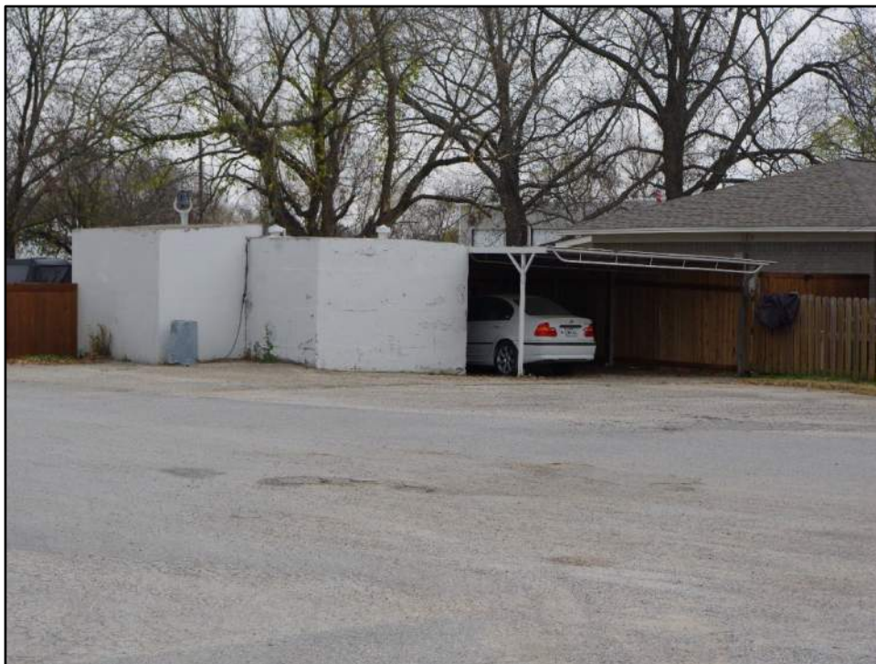
View of Resource 39b carport, camera facing southeast.
