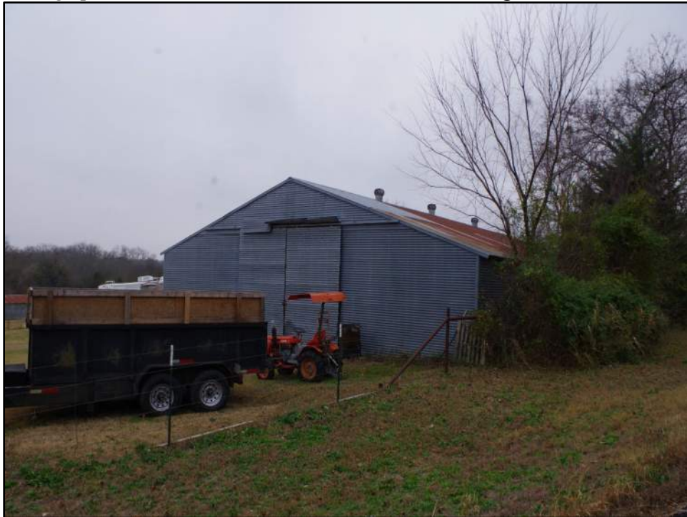
Photograph F-432: View of Resource 98c, camera facing east.
