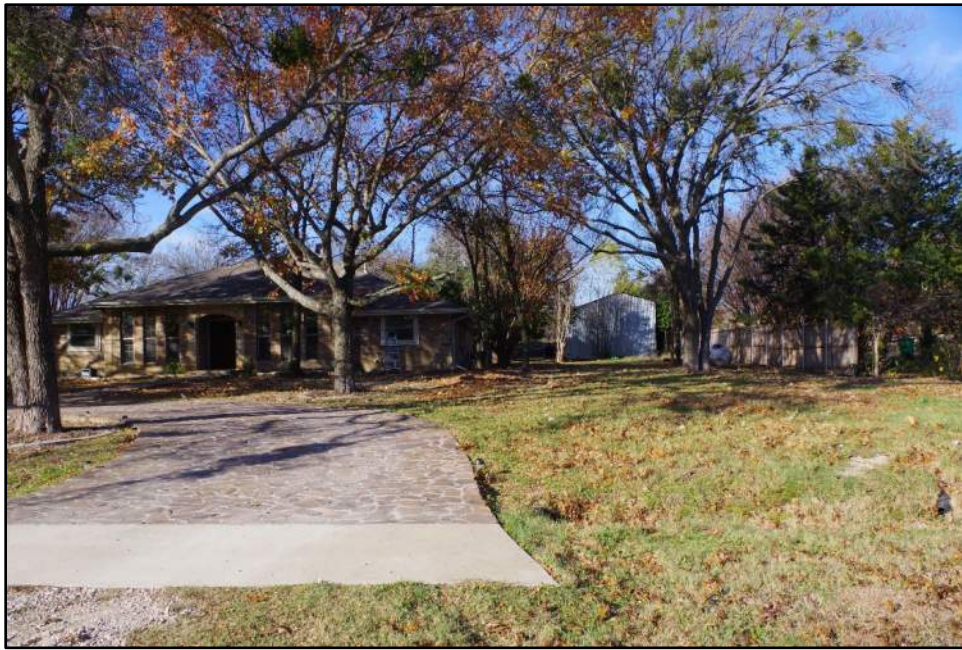
Photograph F-63: Overview of Resource 18, camera facing west.
