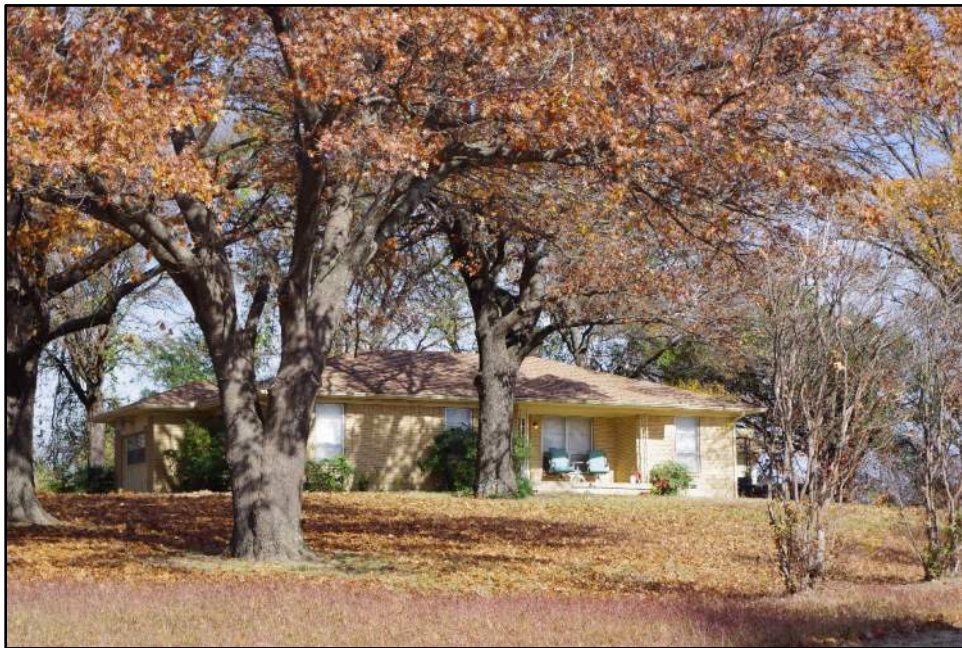
Photograph F-148: View of Resource 31a, camera facing north.
