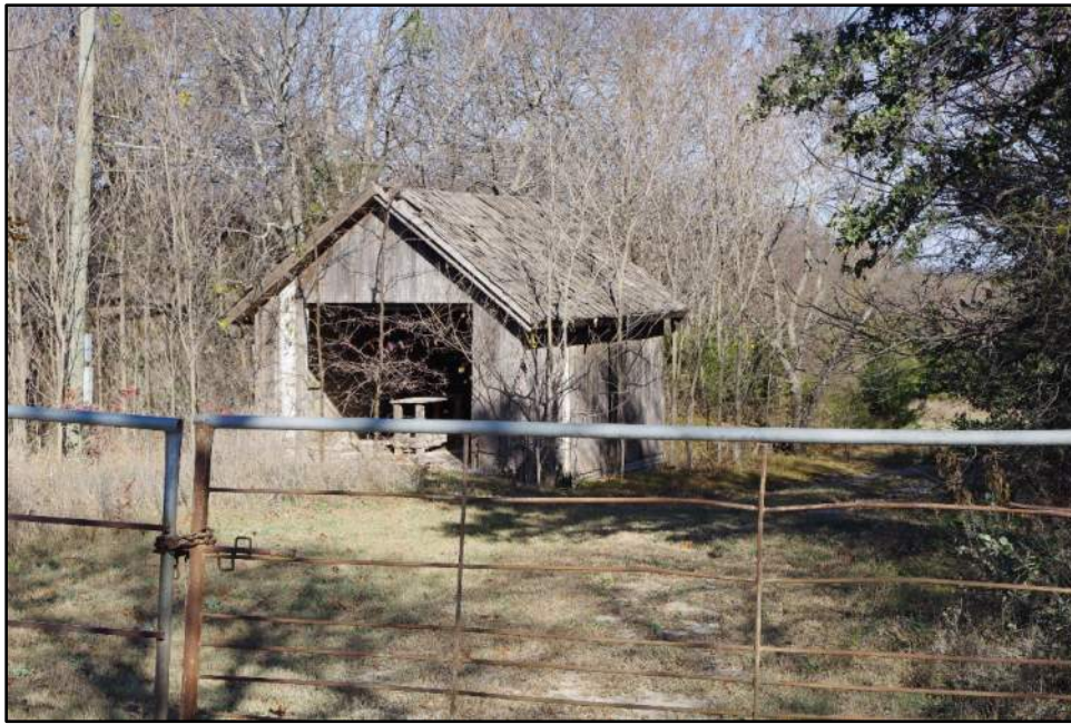
Photograph F-111: View of Resource 23g, camera facing northwest.
