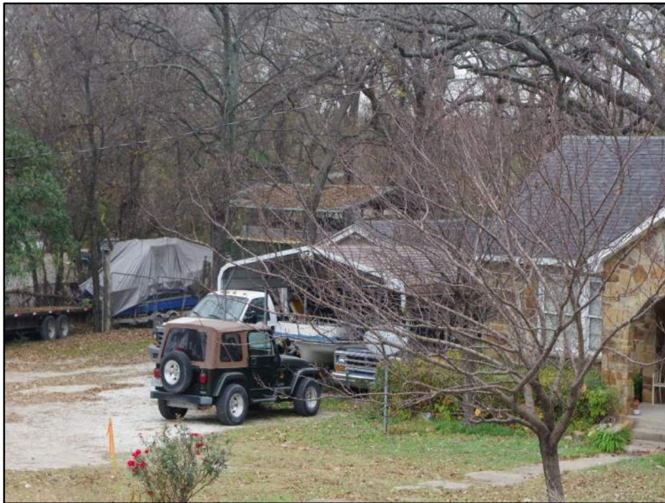
View of Resource 81b (rear) and non-historic-age carport, camera facing northwest.
