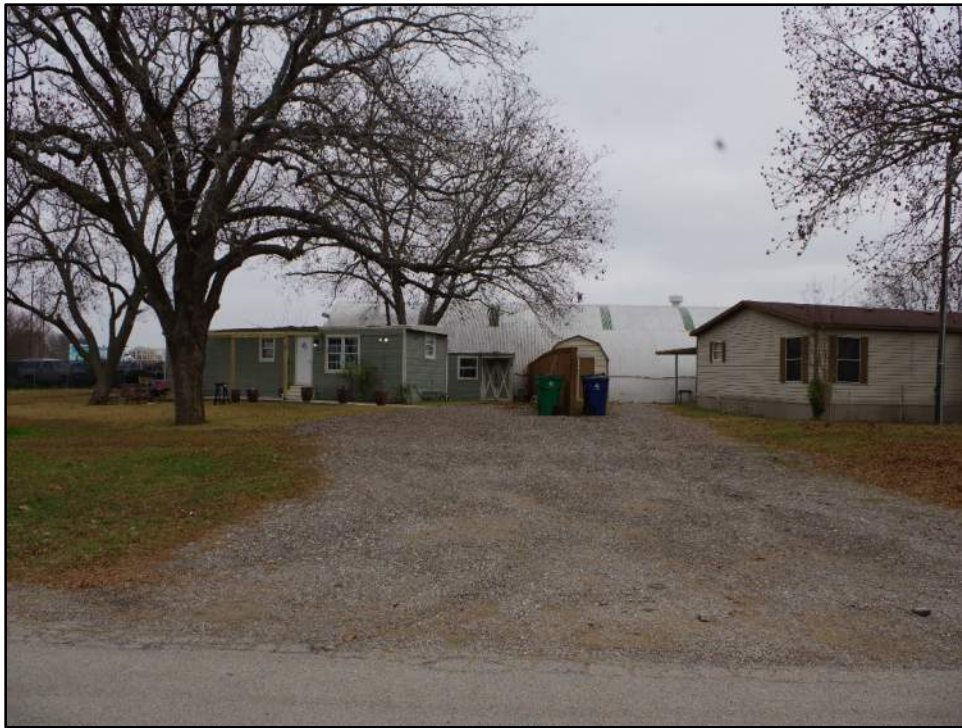
Photograph F-187: View of Resource 38b, camera facing east.
