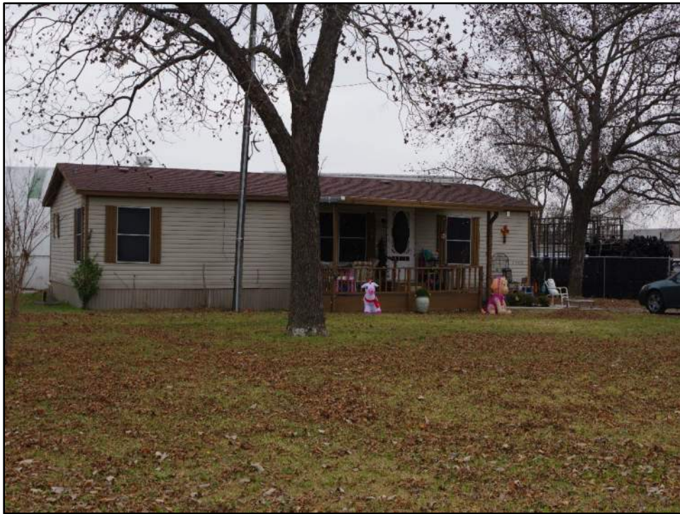
Photograph F-185: View of Resource 38a, camera facing east.
