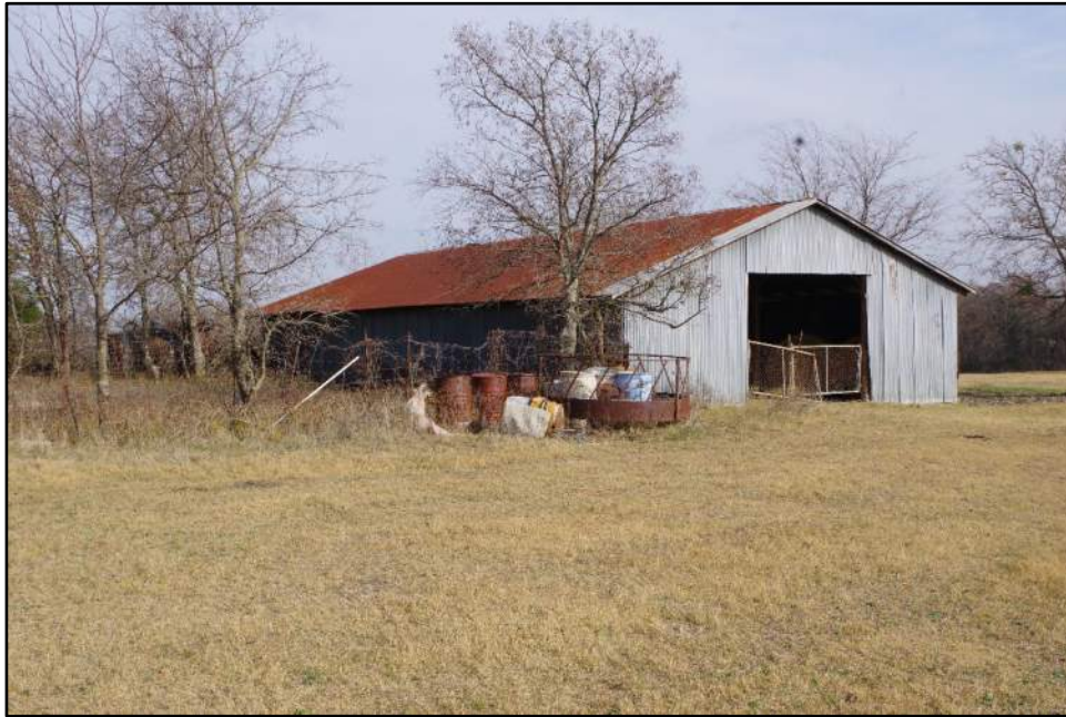
View of Resource 25a, camera facing northeast.
