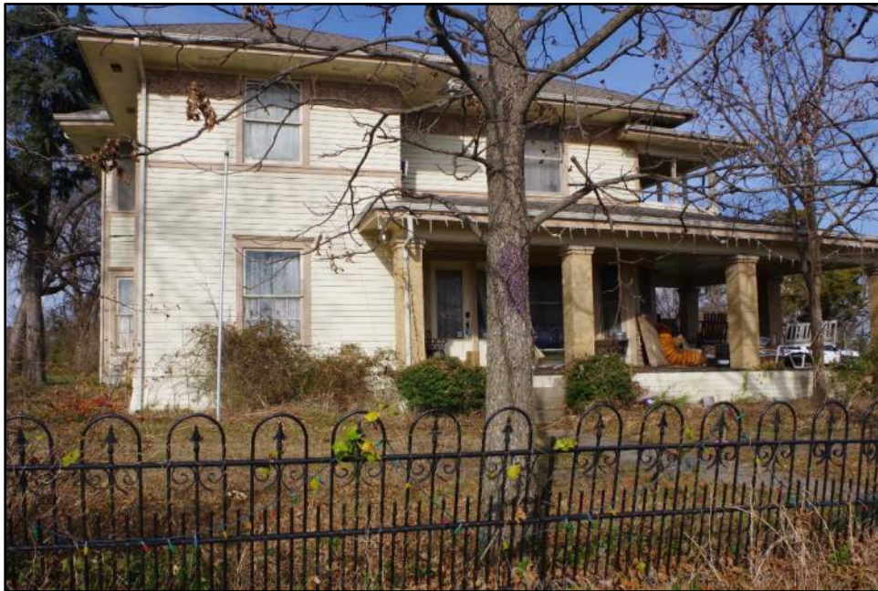
Photograph F-164: View of Resource 34a, camera facing north.
