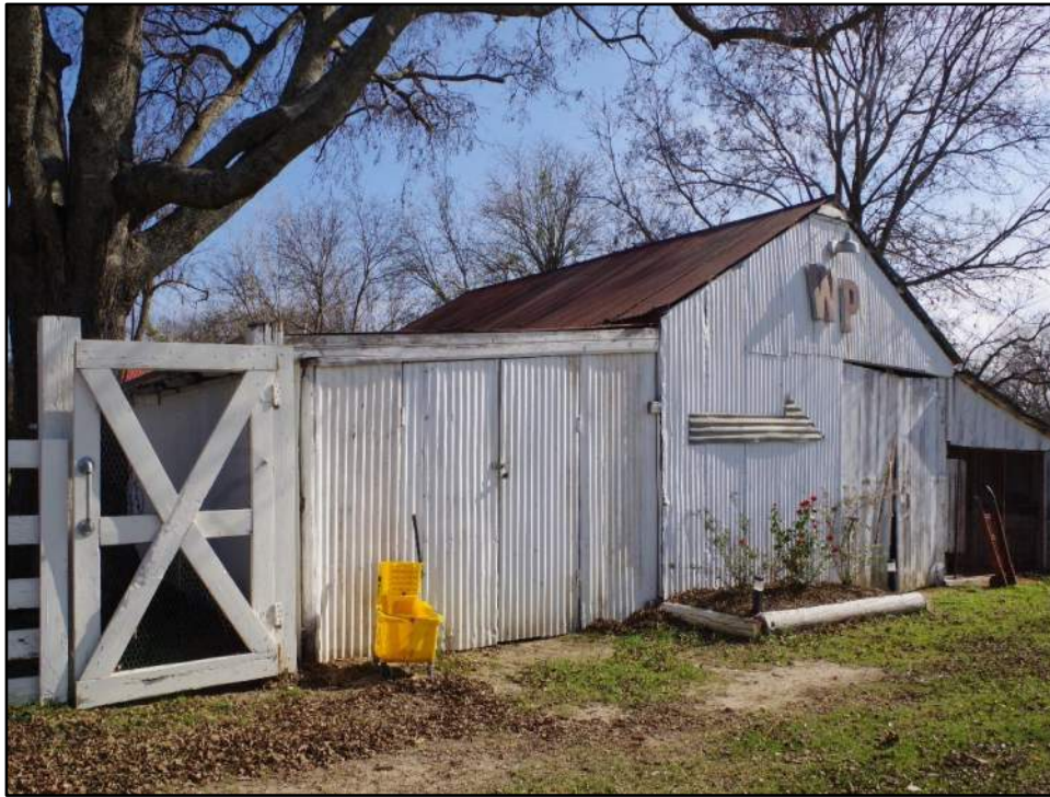
View of Resource 68a, camera facing southwest.
