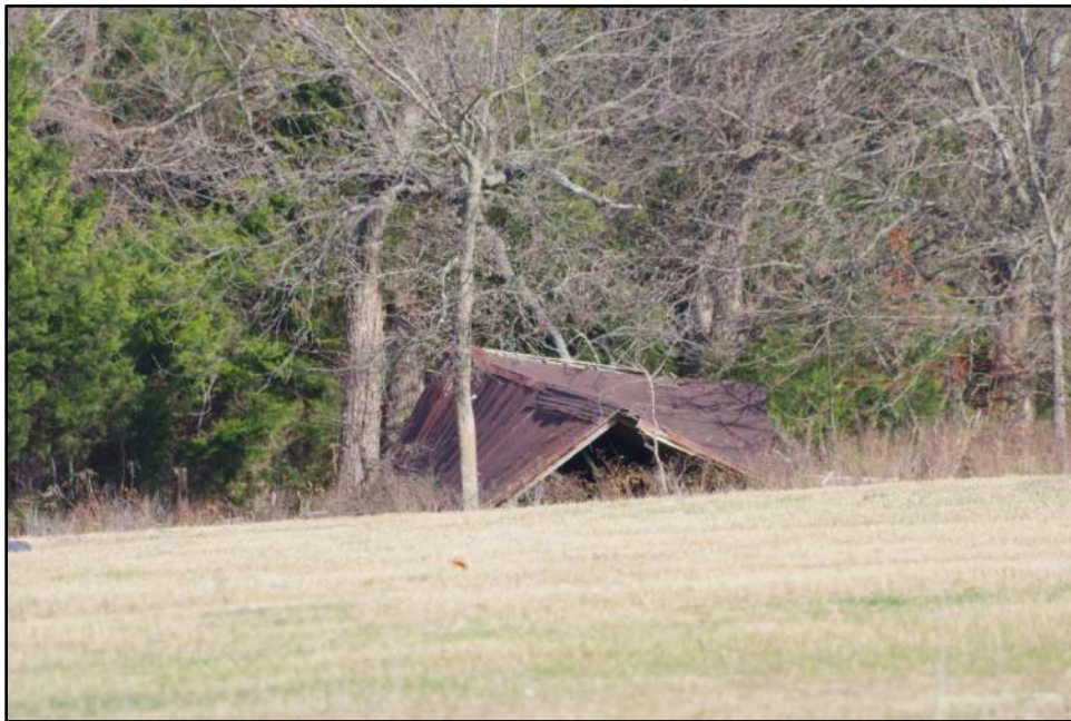
Photograph F-124: View of collapsed building associated with Resource 25, camera facing east.
