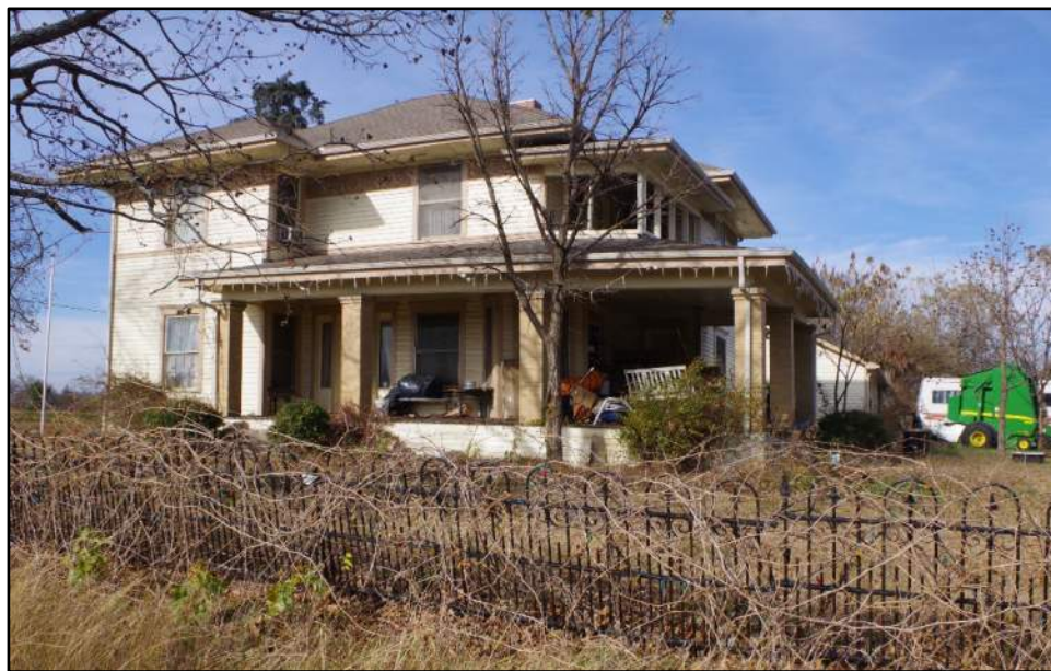
View of Resource 34a, camera facing north.
