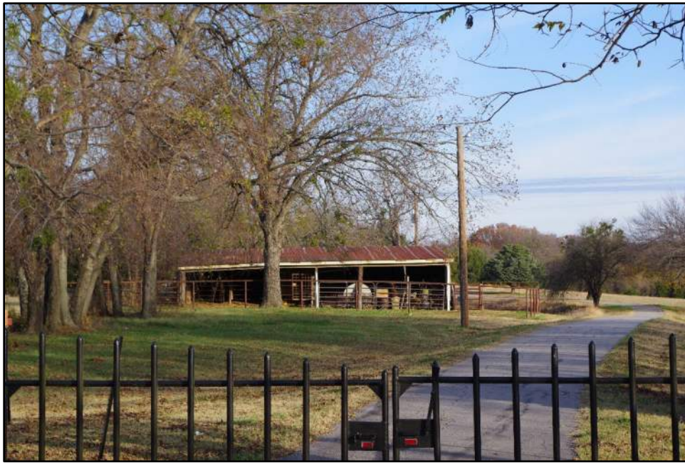
Photograph F-53: View of Resource 16a, camera facing north.
