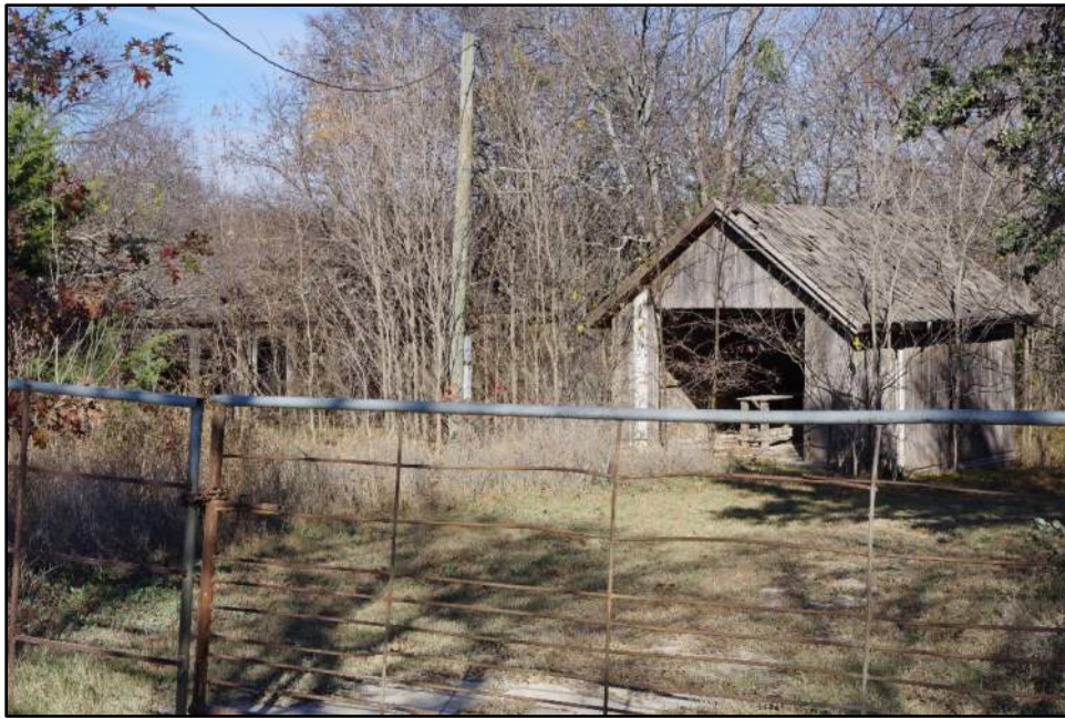
Photograph F-99: Overview of Resource 23, camera facing northwest.
