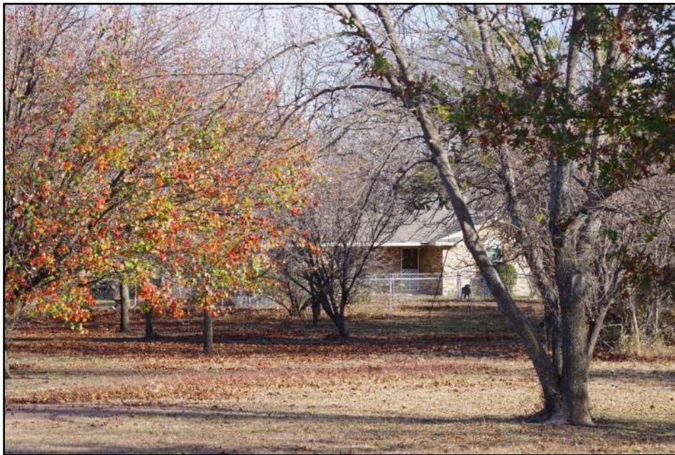
Photograph F-58: View of Resource 17a, camera facing north.
