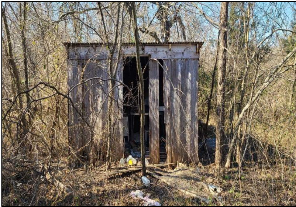
Photograph F-359: Obstructed view of Resource 78e, camera facing west.
