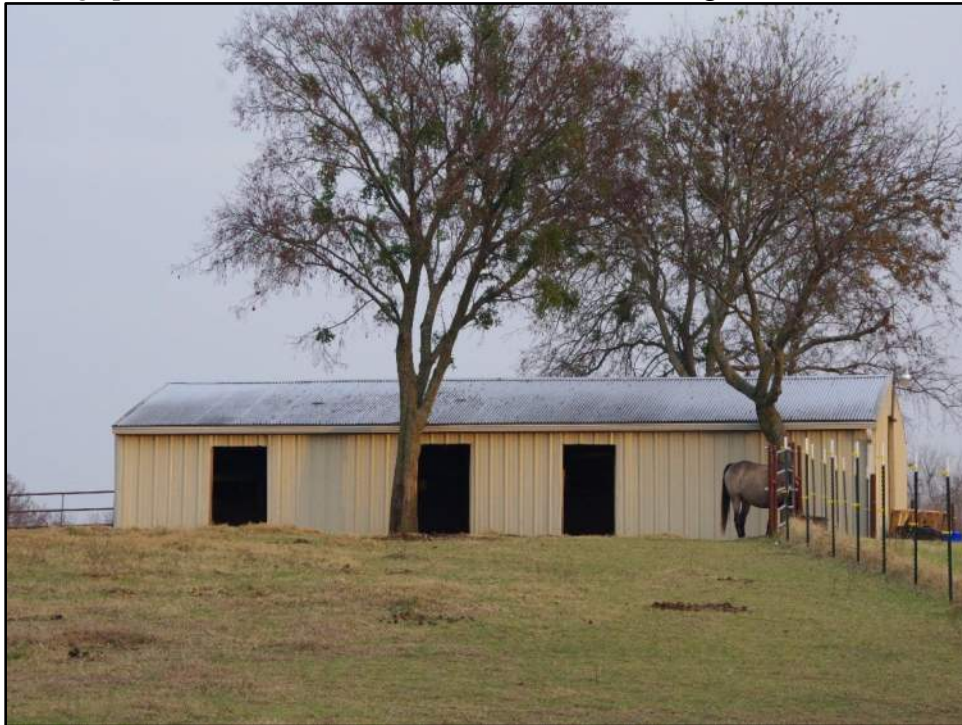
Photograph F-236: View of Resource 50b, camera facing northeast.
