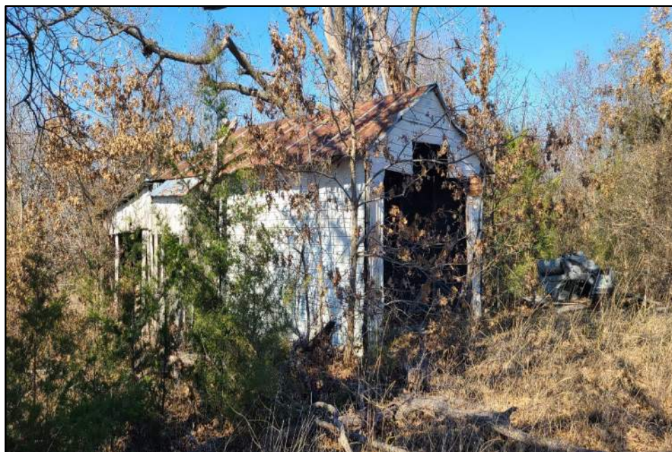
Obstructed view of Resource 78d, camera facing northeast.
