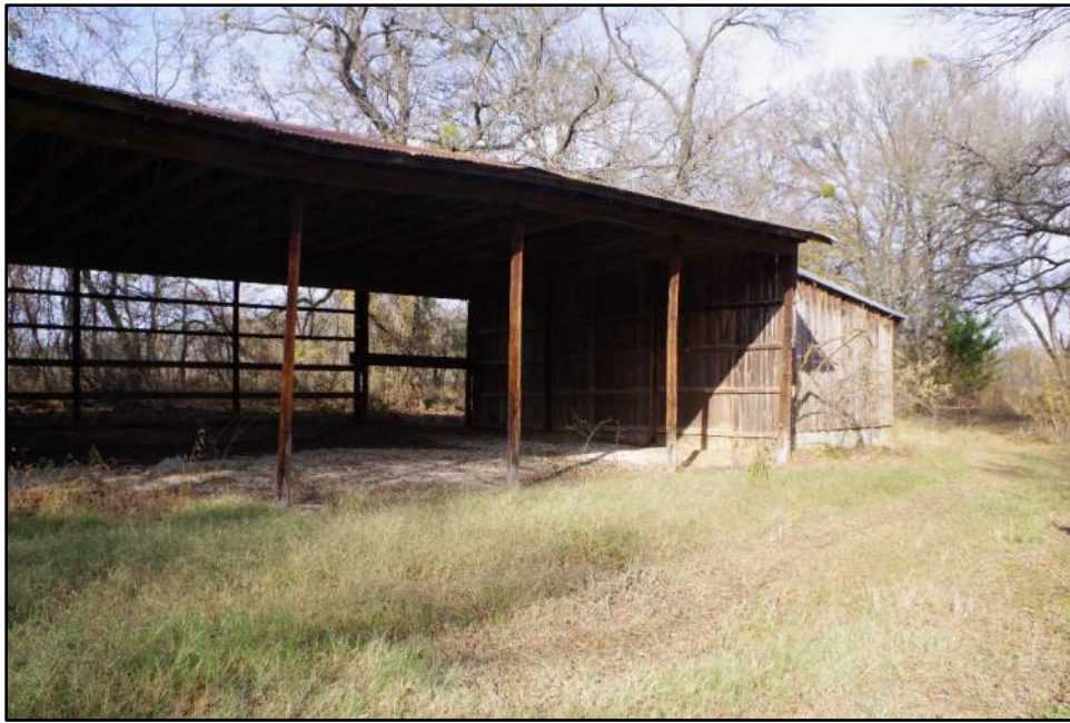
Photograph F-107: View of Resource 23c, camera facing north-northwest.
