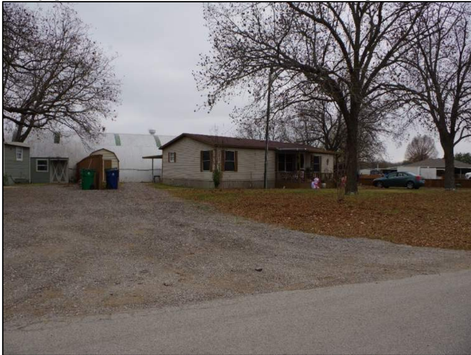
Photograph F-184: View of Resource 38a, camera facing east.
