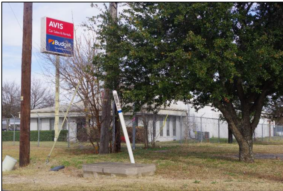
Obstructed view of Resource 33, camera facing northeast.
