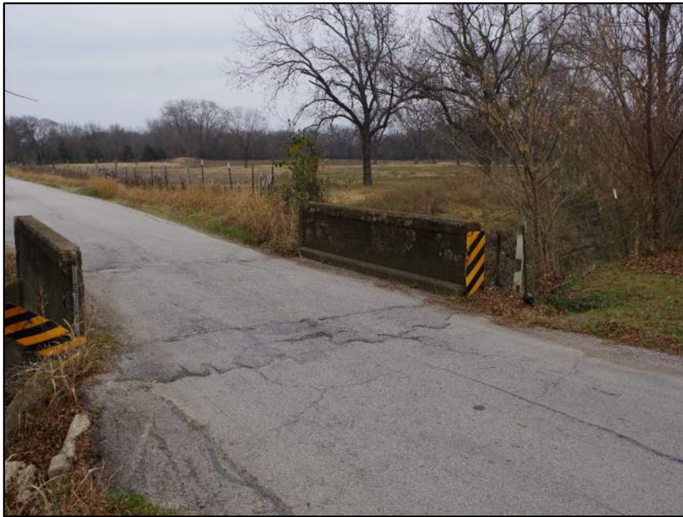
Photograph F-179: View of Resource 37, camera facing southwest.
