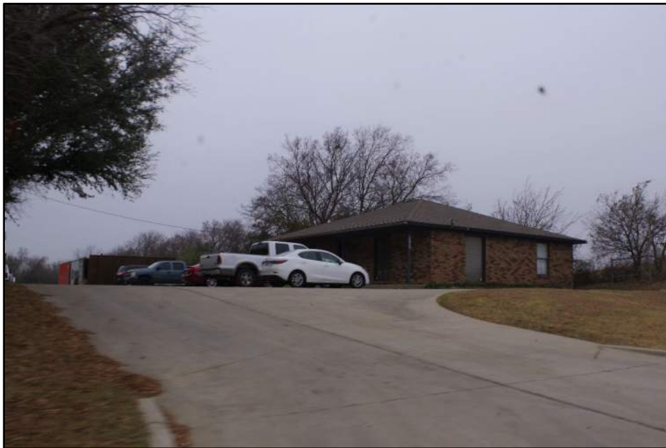
Photograph F-38: View of Resource 11, camera facing southwest.
