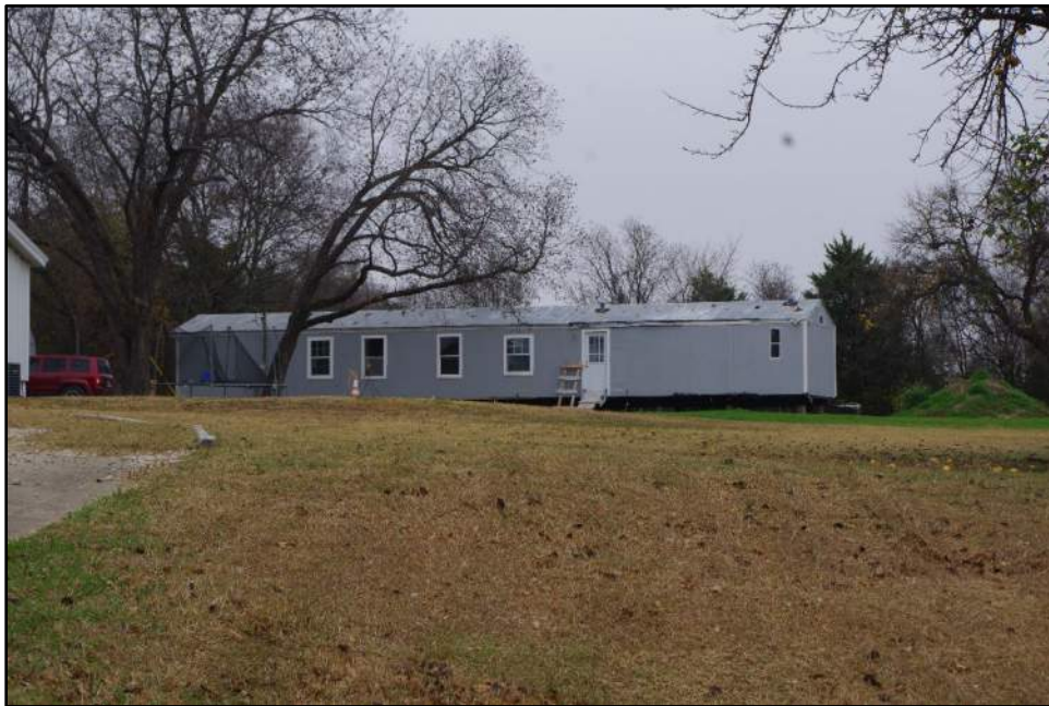
Photograph F-426: View of Resource 97c, camera facing northwest.
