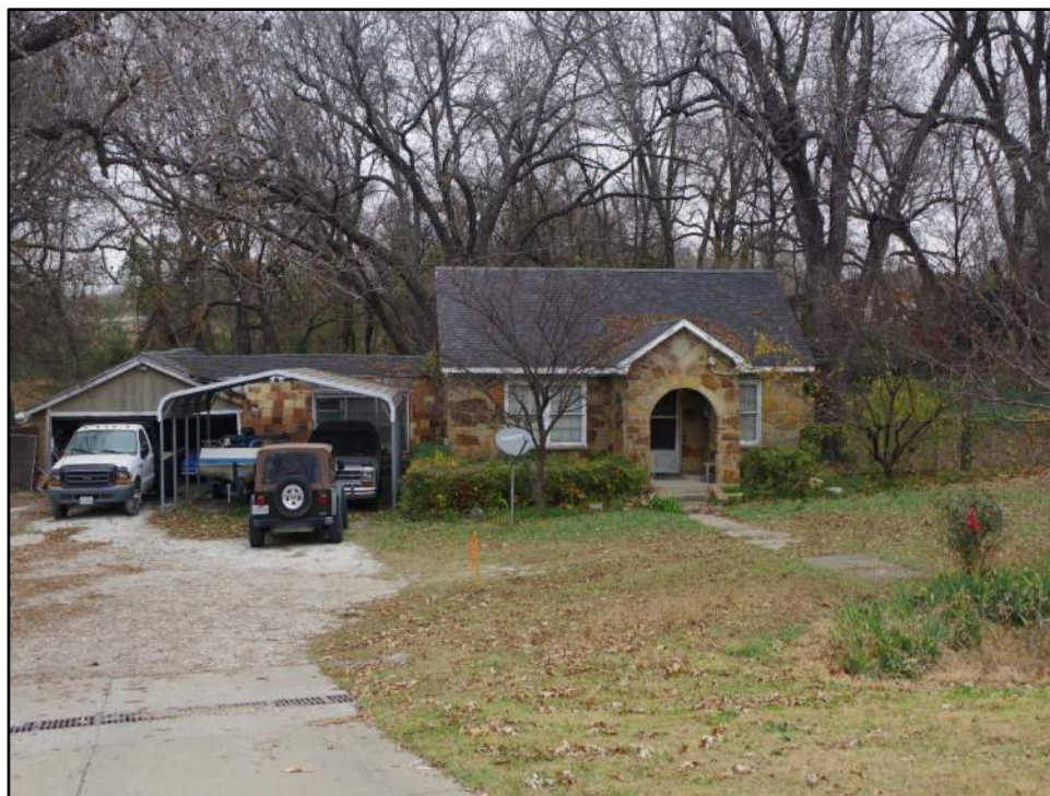
View of Resource 81a and non-historic-age carport, camera facing north.
