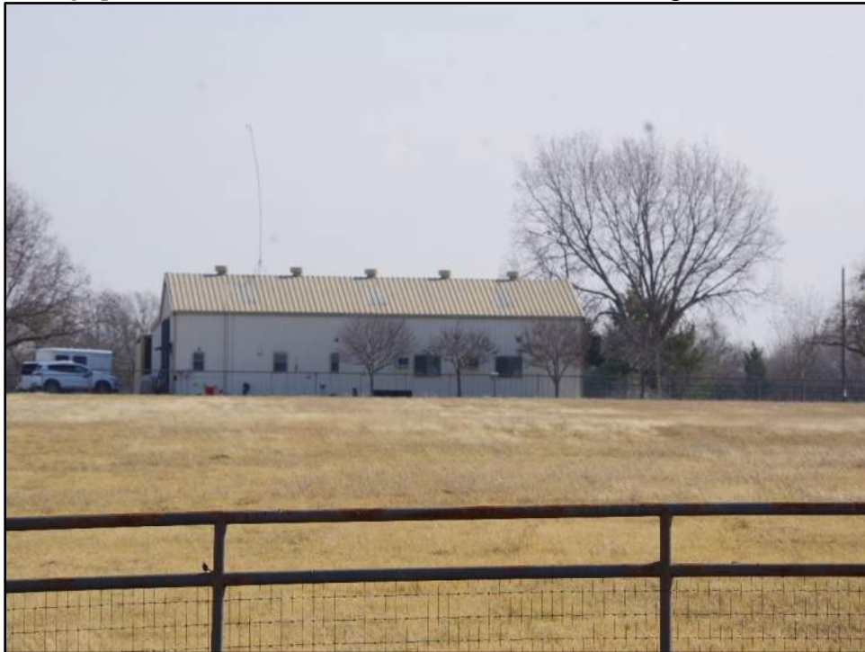
Photograph F-260: View of Resource 55a, camera facing east.
