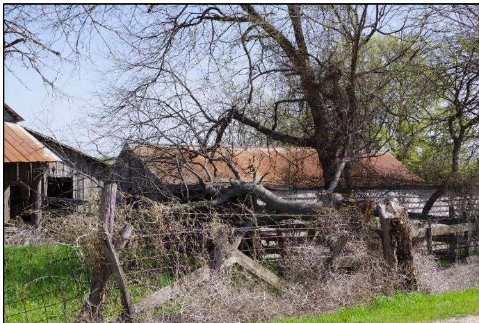
View of Resource 22g, camera facing northeast.
