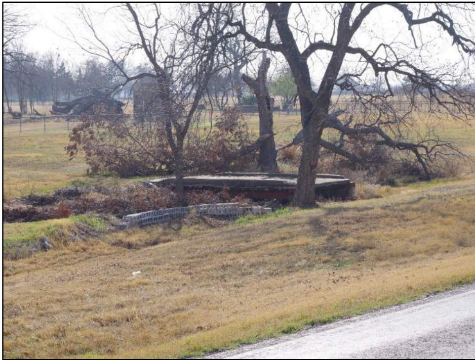
Photograph F-263: View of Resource 55b, camera facing southeast.
