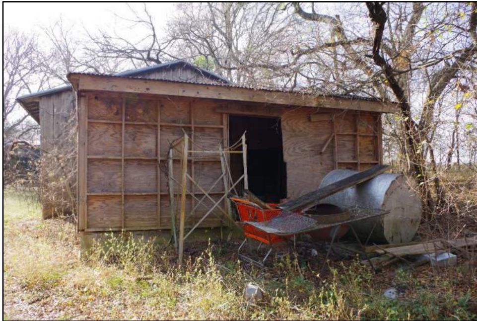
View of Resource 23e, camera facing south.
