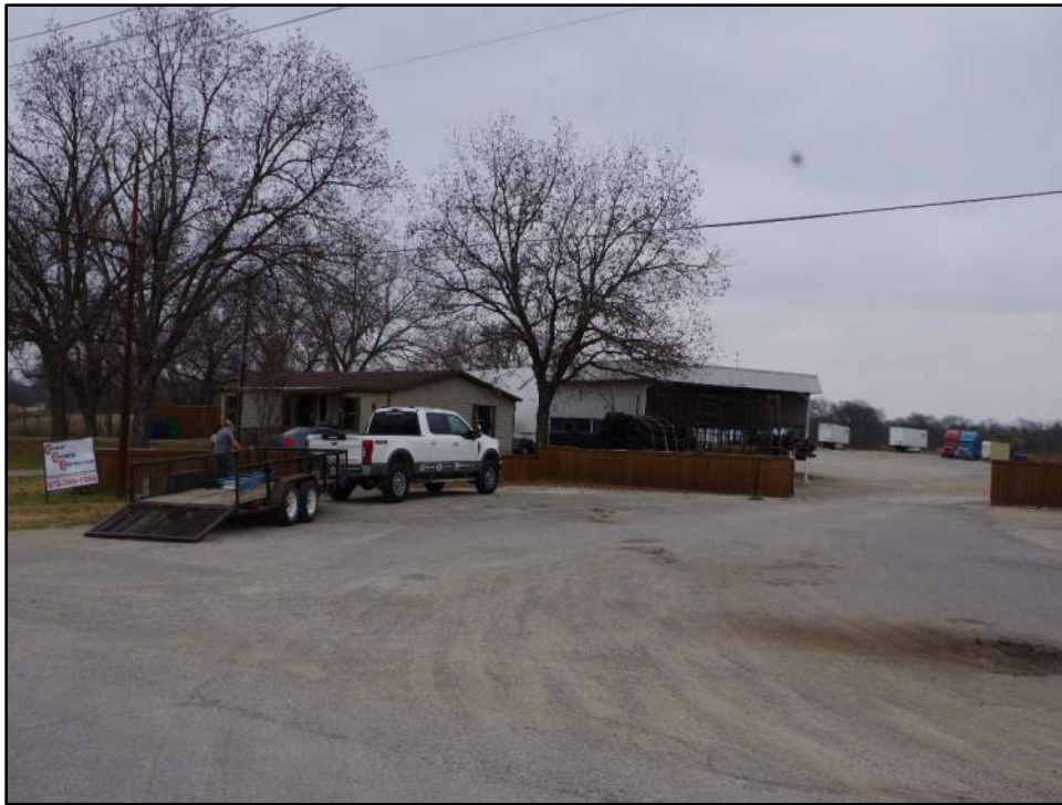
Photograph F-191: View of Resource 39c (right), camera facing northeast.
