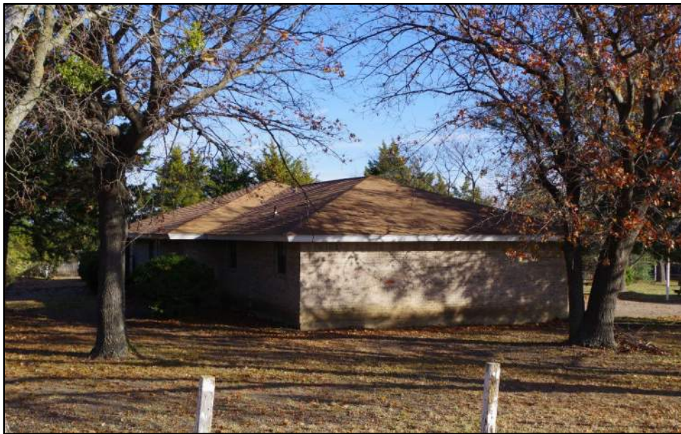
Photograph F-68: View of Resource 19a, camera facing east.
