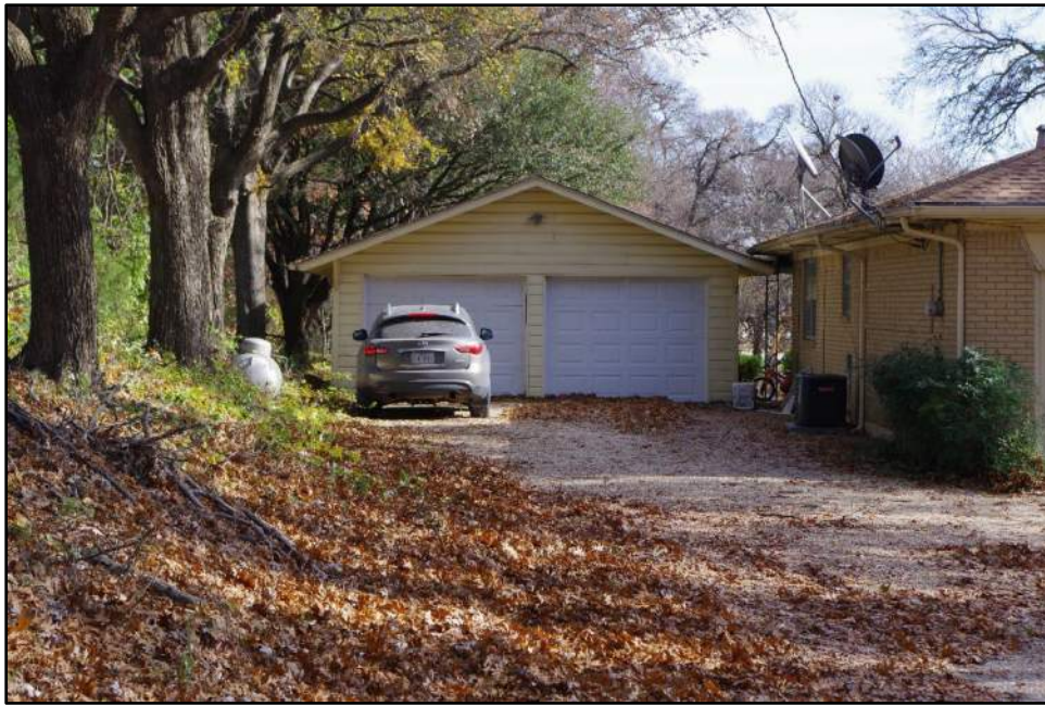
Photograph F-151: View of Resource 31b, camera facing east.
