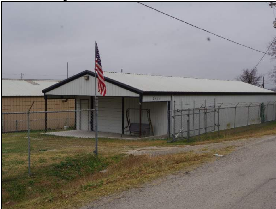
Photograph F-386: View of non-historic-age buildings associated with Resource 86, camera facing southwest.
