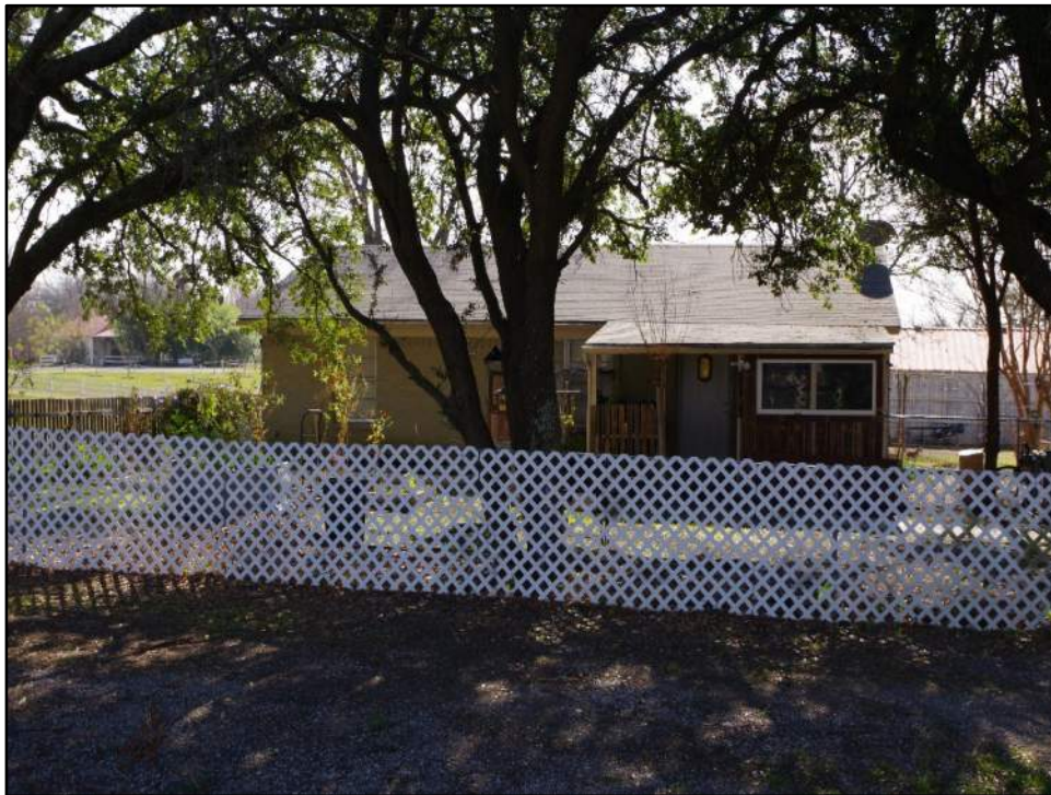
View of Resource 67a, camera facing south
