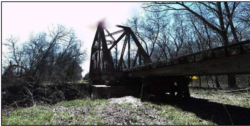
Photograph 16: Railroad Truss Bridge over East Fork Trinity River.
