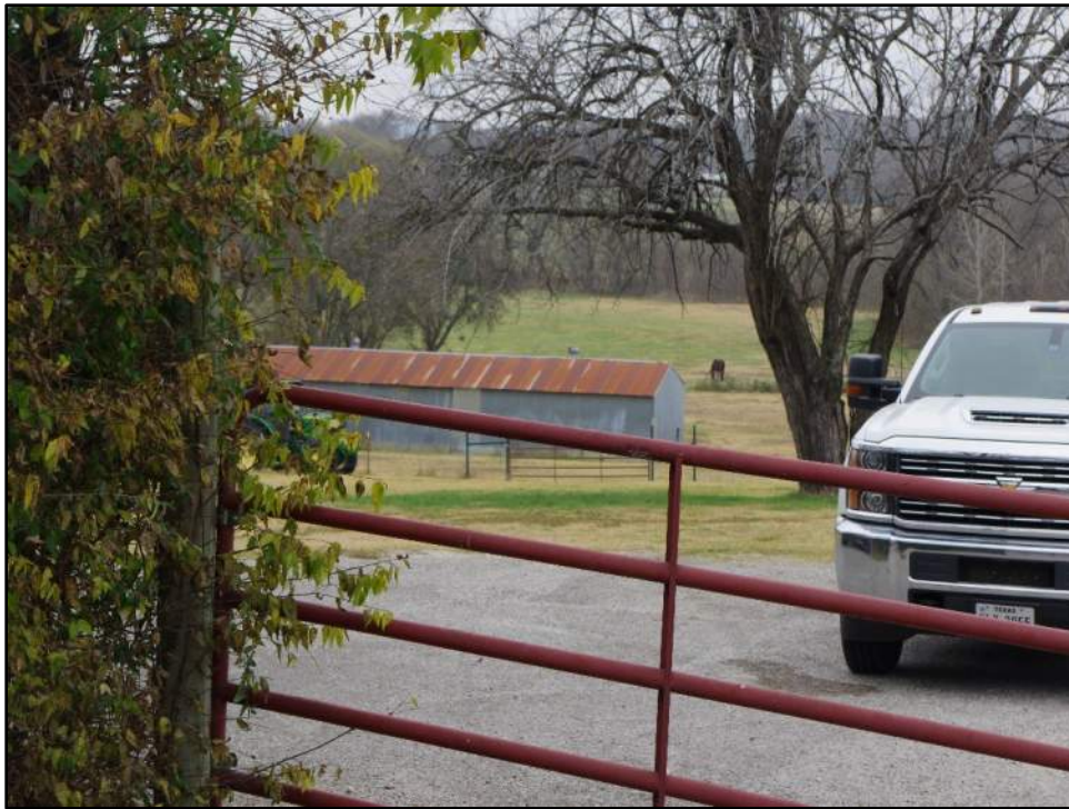
Photograph F-431: View of Resource 98b, camera facing northeast.
