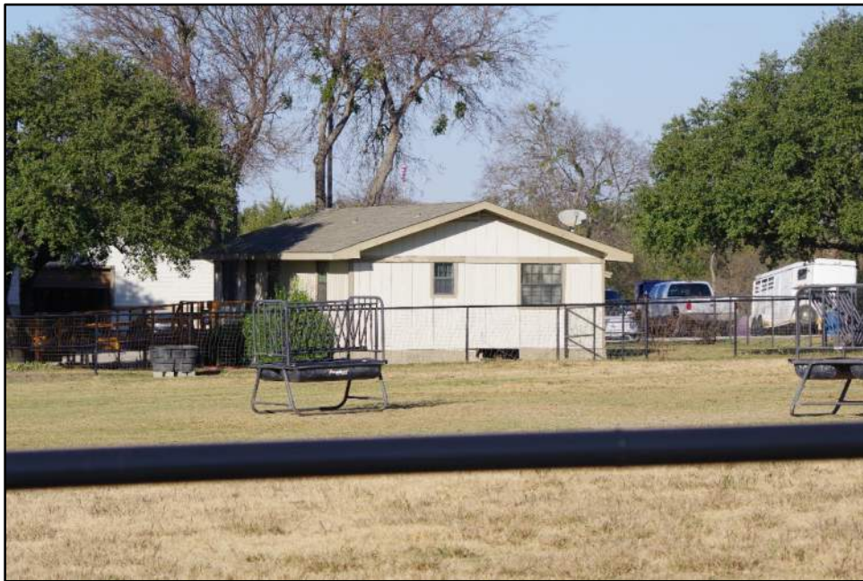
Photograph F-22: View of Resource 07a, camera facing north.
