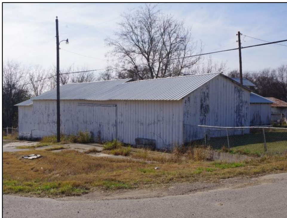
View of Resource 58d, camera facing southwest.
