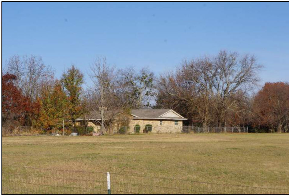
View of Resource 17a, camera facing northwest.
