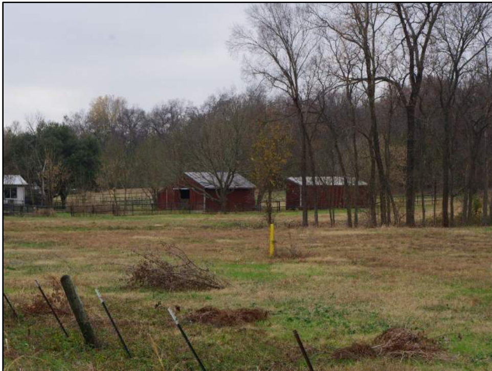
Photograph F-203: View of non-historic-age outbuildings associated with Resource 43, camera facing southwest.
