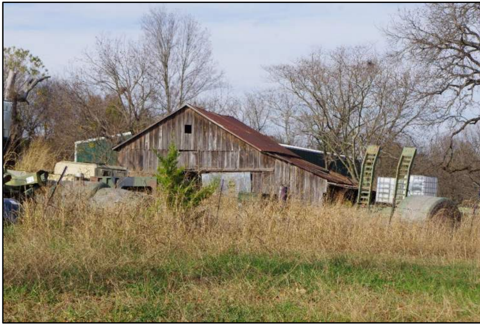
Photograph F-167: View of Resource 34b, camera facing north.
