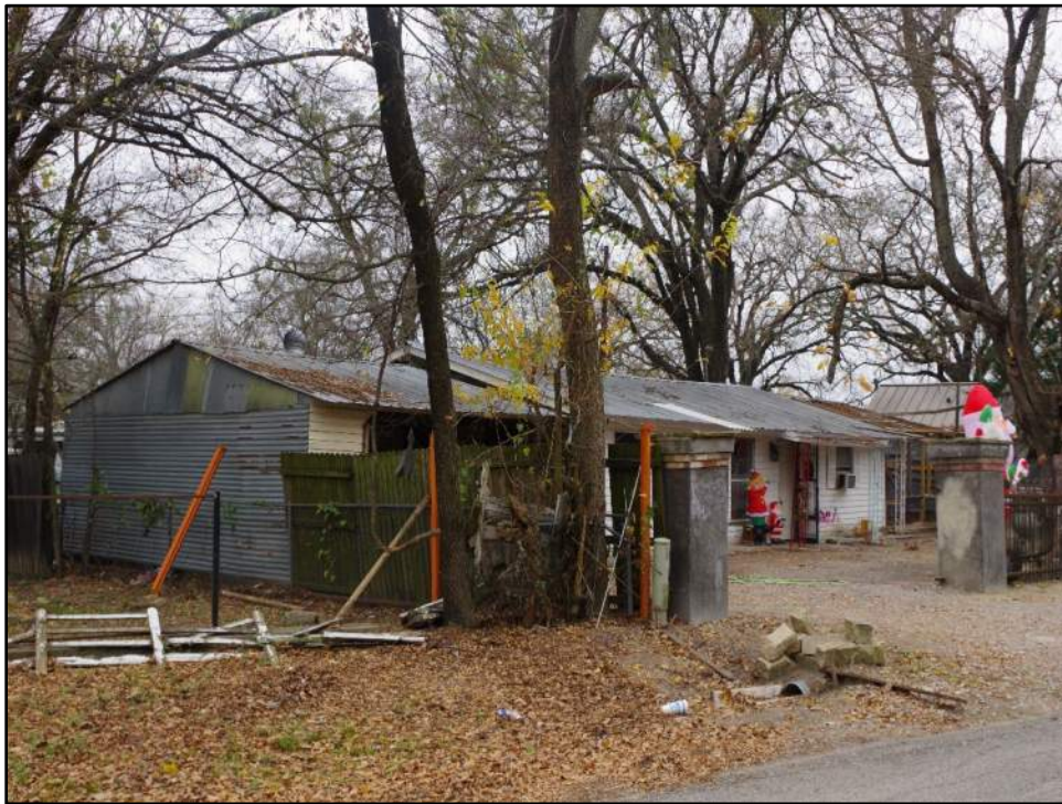
Photograph F-406: View of Resource 92, camera facing southwest.
