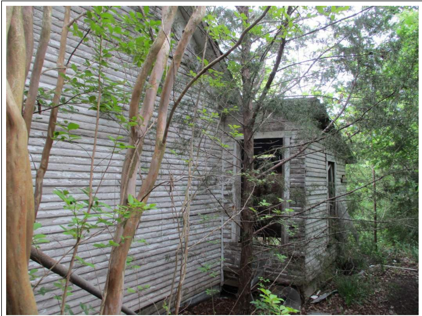
Resource 01b eastern elevation, facing northwest.
