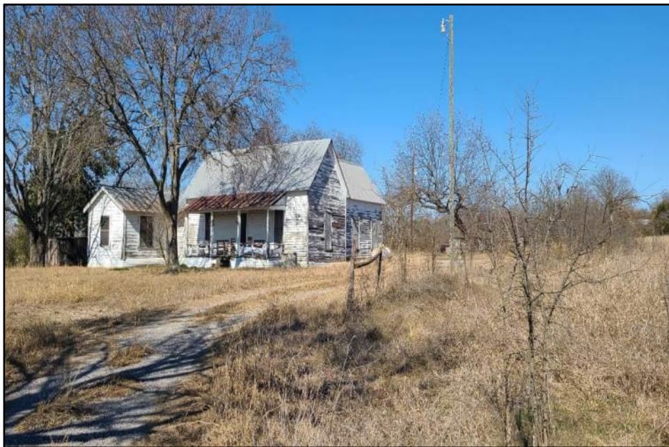
View of Resource 78a, camera facing northwest.
