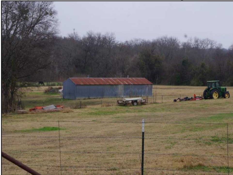
Photograph F-430: View of Resource 98b, camera facing northeast.
