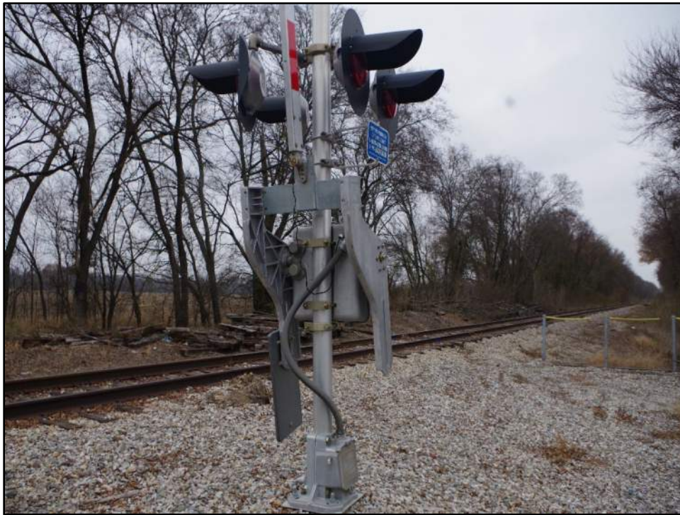
Photograph F-171: View of Resource 35a, camera facing north.
