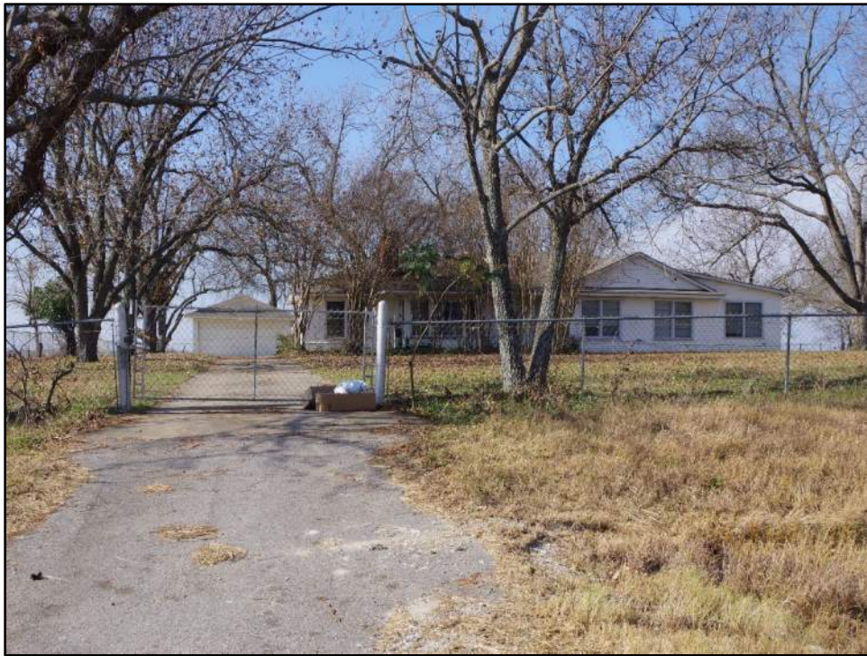
Photograph F-283: View of Resource 58a (right) and 58b (left), camera facing west.
