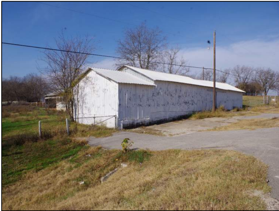
Photograph F-289: View of Resource 58d, camera facing northwest.
