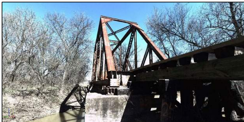
View of Resource 35b, camera facing north.
