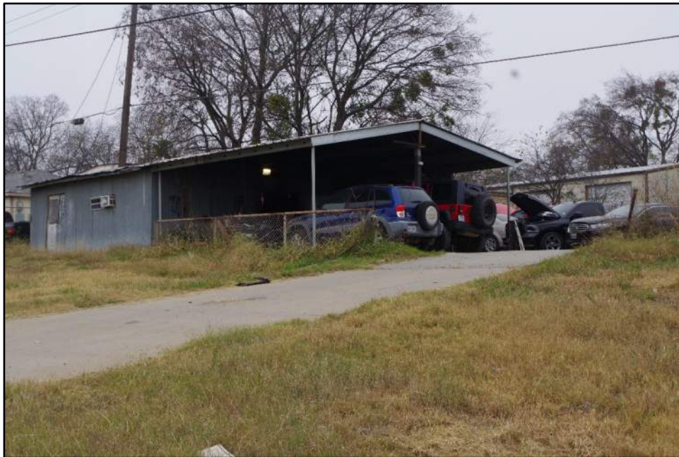
View of Resource 100a, camera facing northwest.
