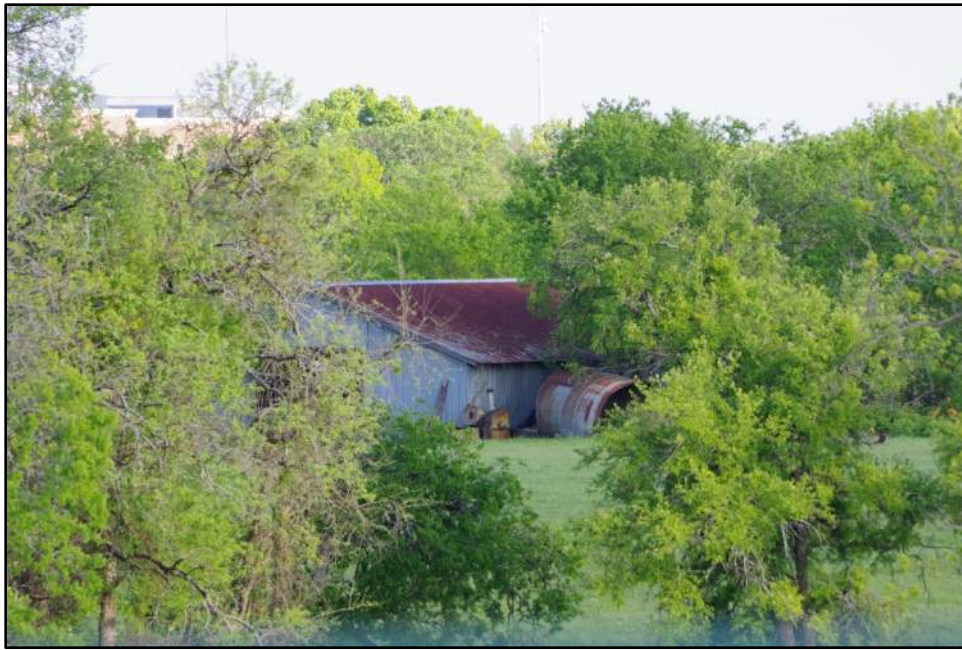
Photograph 51: Obstructed view of historic-age barn, camera facing east.
