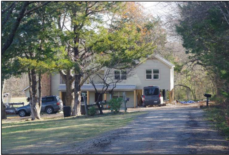
View of Resource 27, camera facing east.
