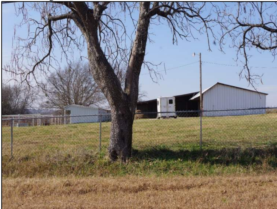
Photograph F-286: View of Resource 58c (right) and non-historic-age pole barn (left), camera facing west.
