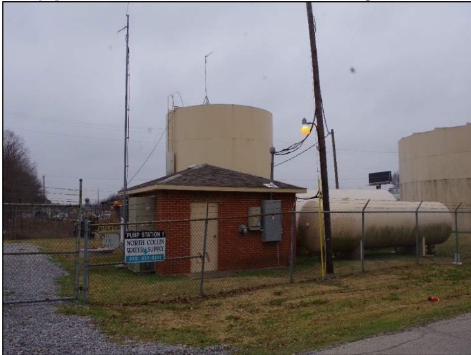
Photograph F-398: View of Resource 90a and Resource 90b (rear), camera facing southwest.
