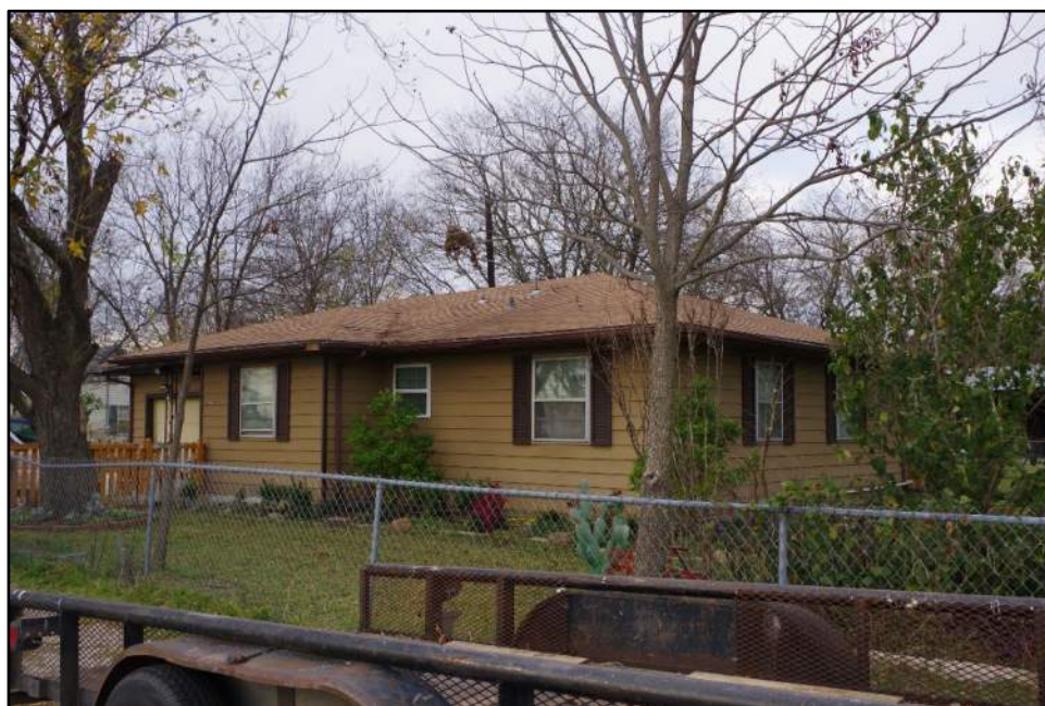
View of Resource 72a, camera facing northwest.
