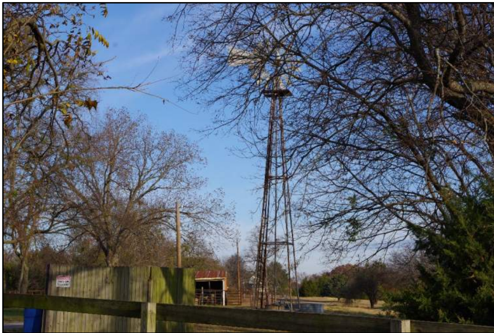
Photograph F-54: View of Resource 16b (windmill), camera facing north.
