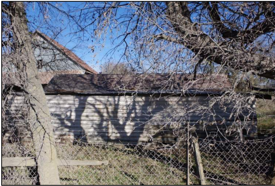
Photograph F-93: View of Resource 22g, camera facing north.
