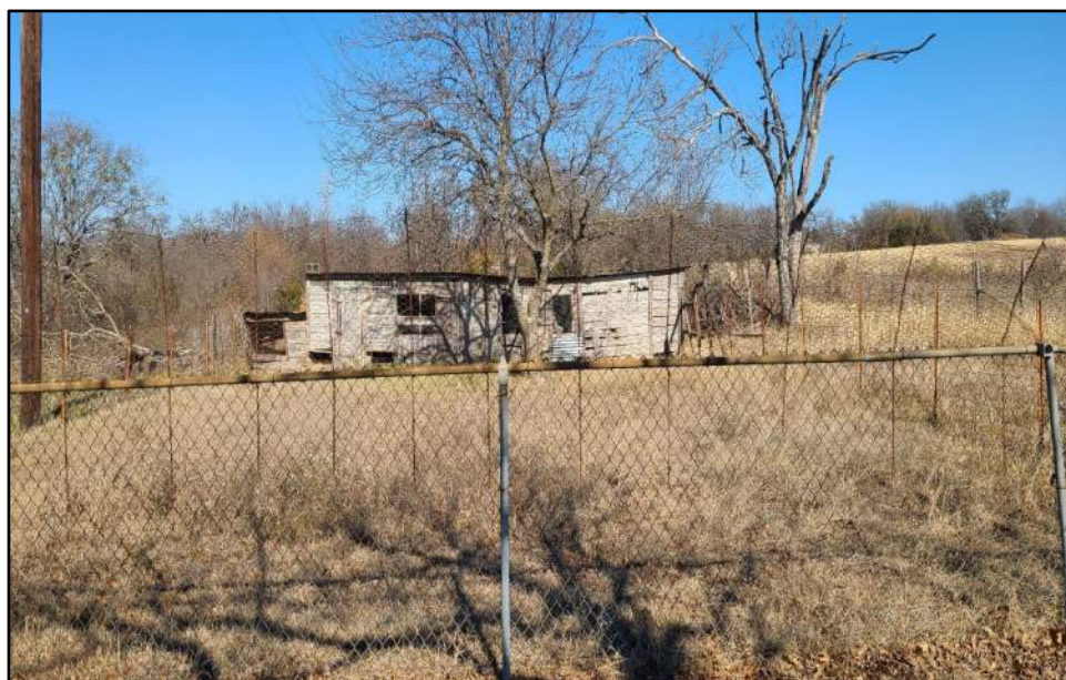
View of Resource 78c, camera facing north.
