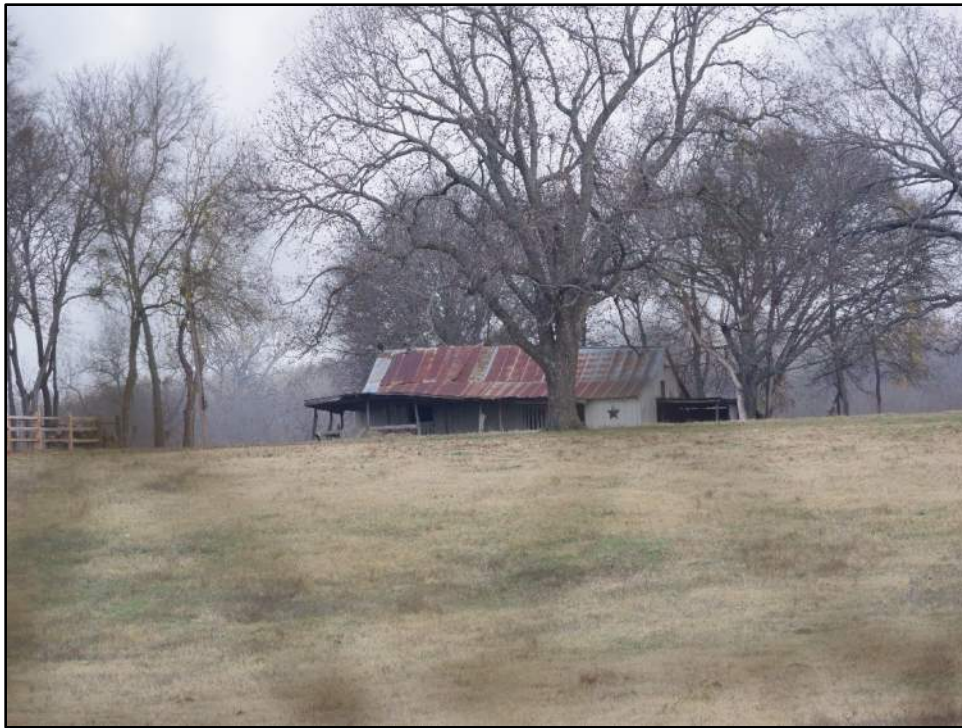
Photograph F-249: View of Resource 53b, camera facing north
