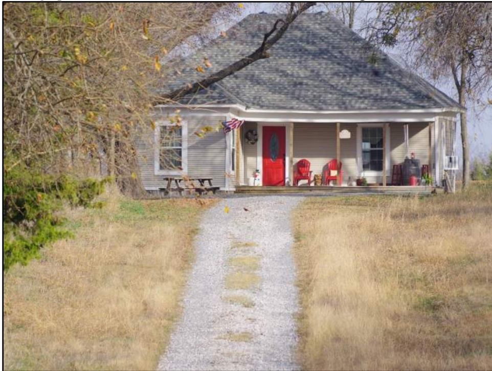
Photograph F-246: View of Resource 53a, camera facing north.
