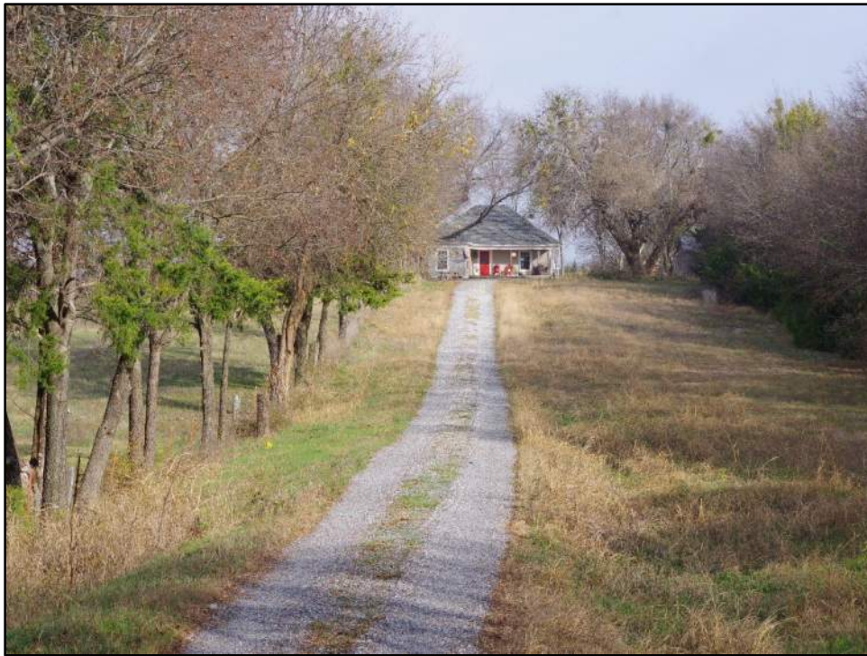
Photograph F-245: View of Resource 53a, camera facing north.
