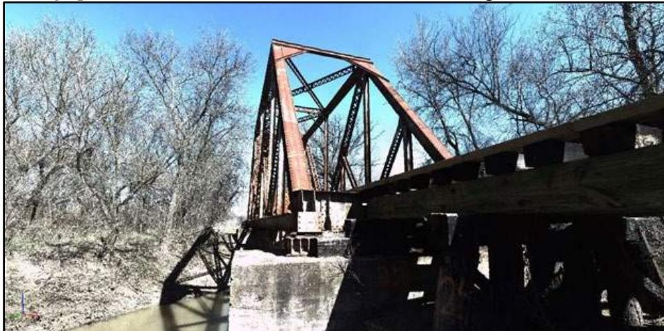
Photograph F-174: View of Resource 35b, camera facing north.
