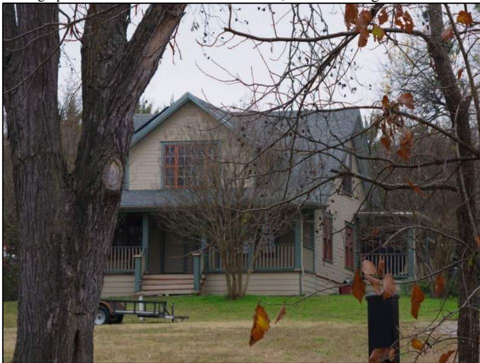
Photograph F-214: View of Resource 46, camera facing southwest.
