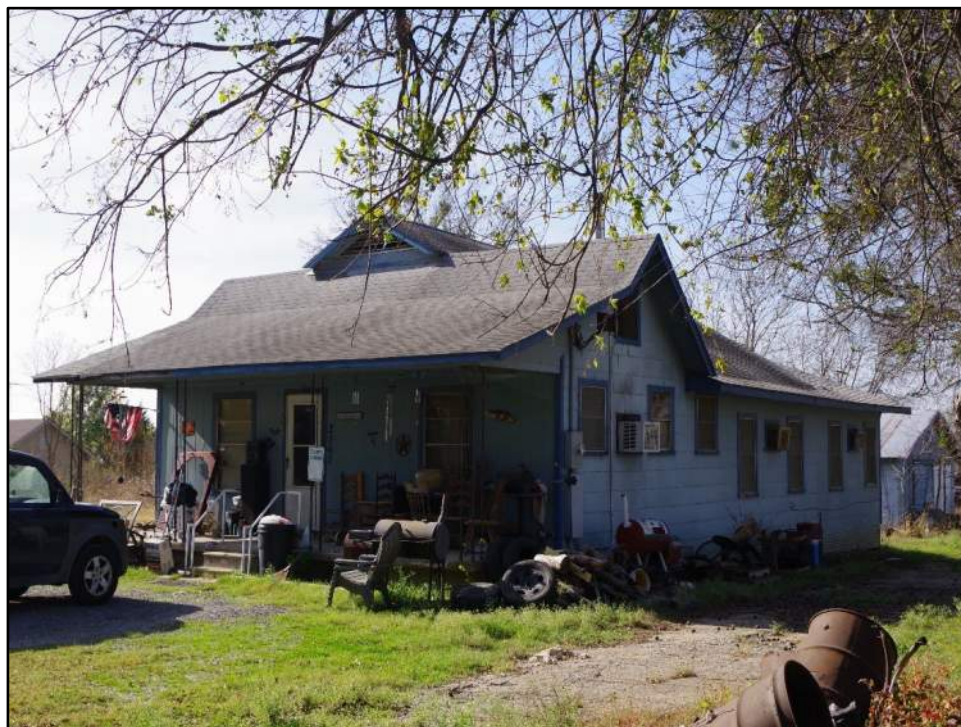
View of Resource 63a, camera facing southwest.
