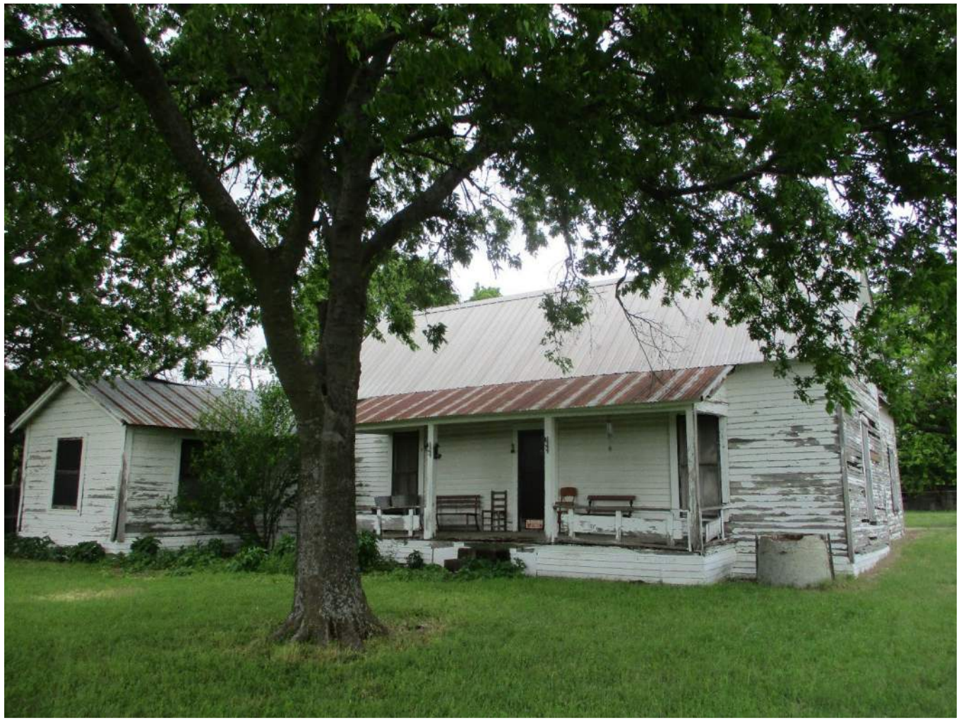
Resource 01a southern elevation, facing northwest.
