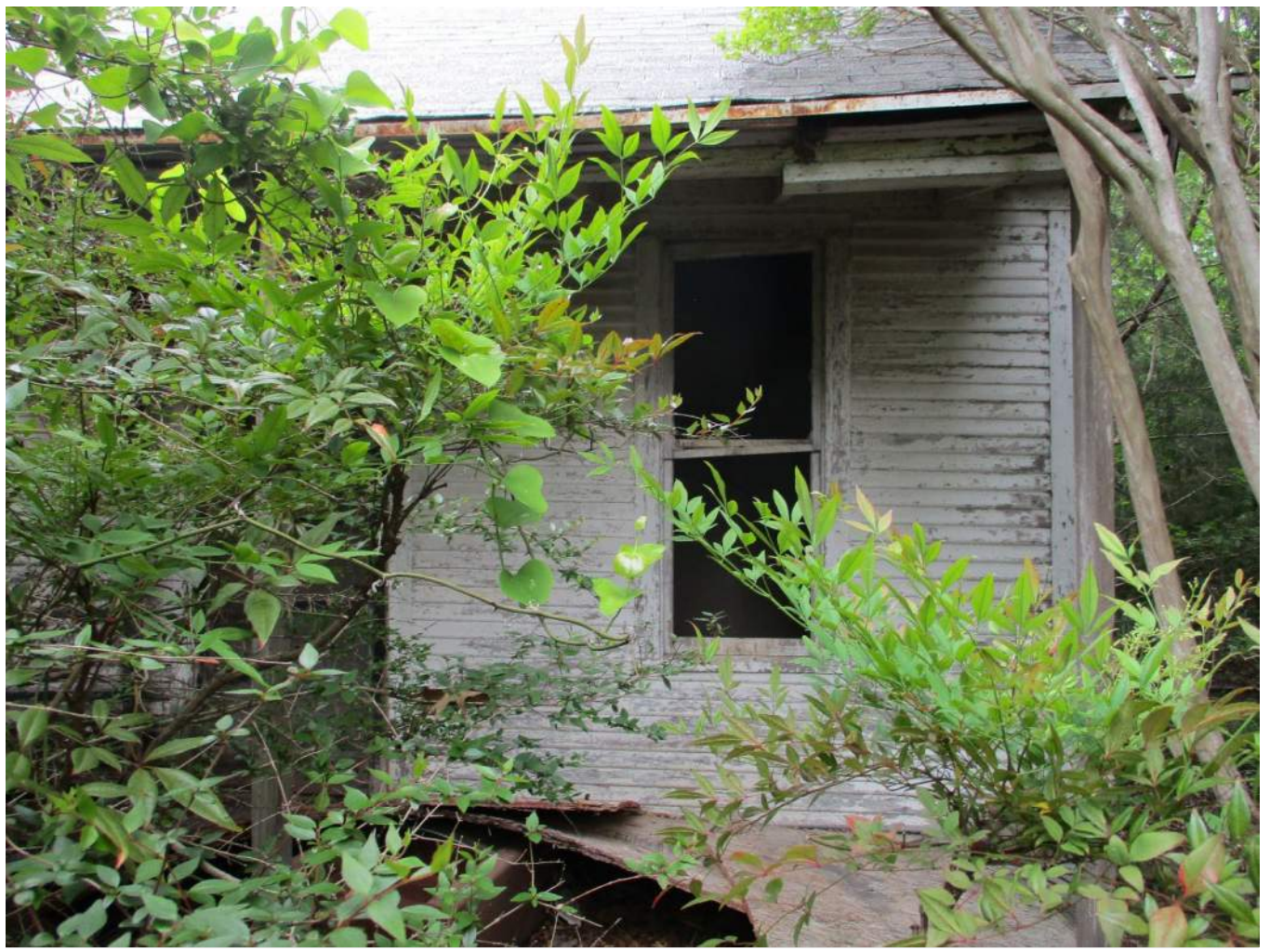
Resource 01b southern elevation, facing north.
