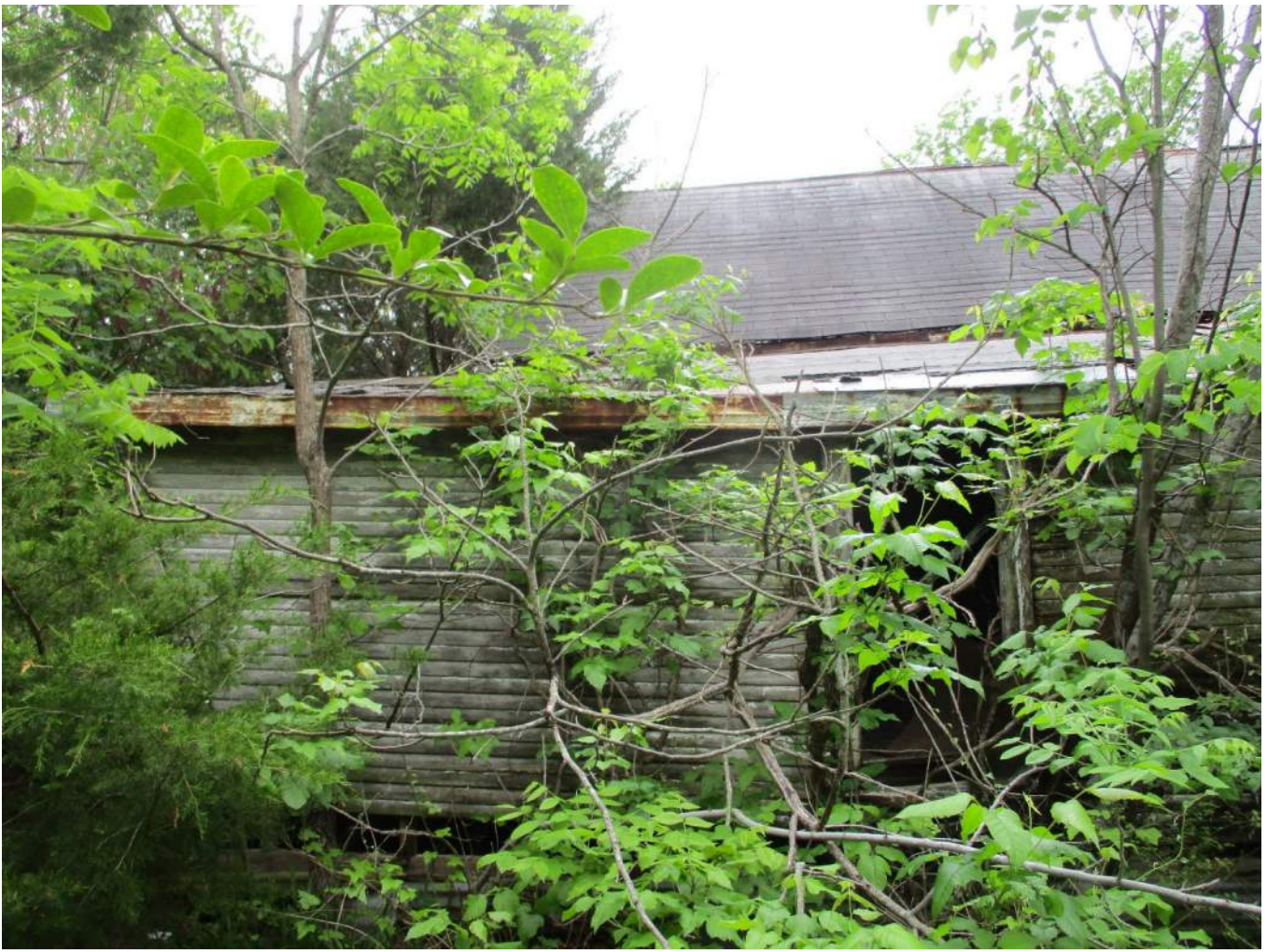
Resource 01b northern elevation, facing south.
