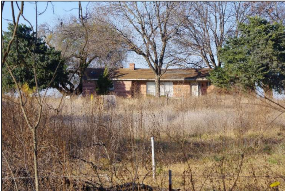
Photograph F-42: View of Resource 13a, camera facing north.
