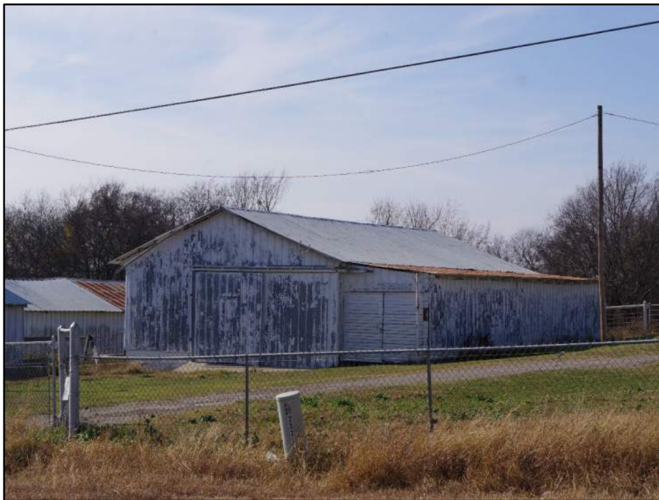
View of Resource 58f, camera facing southwest.
