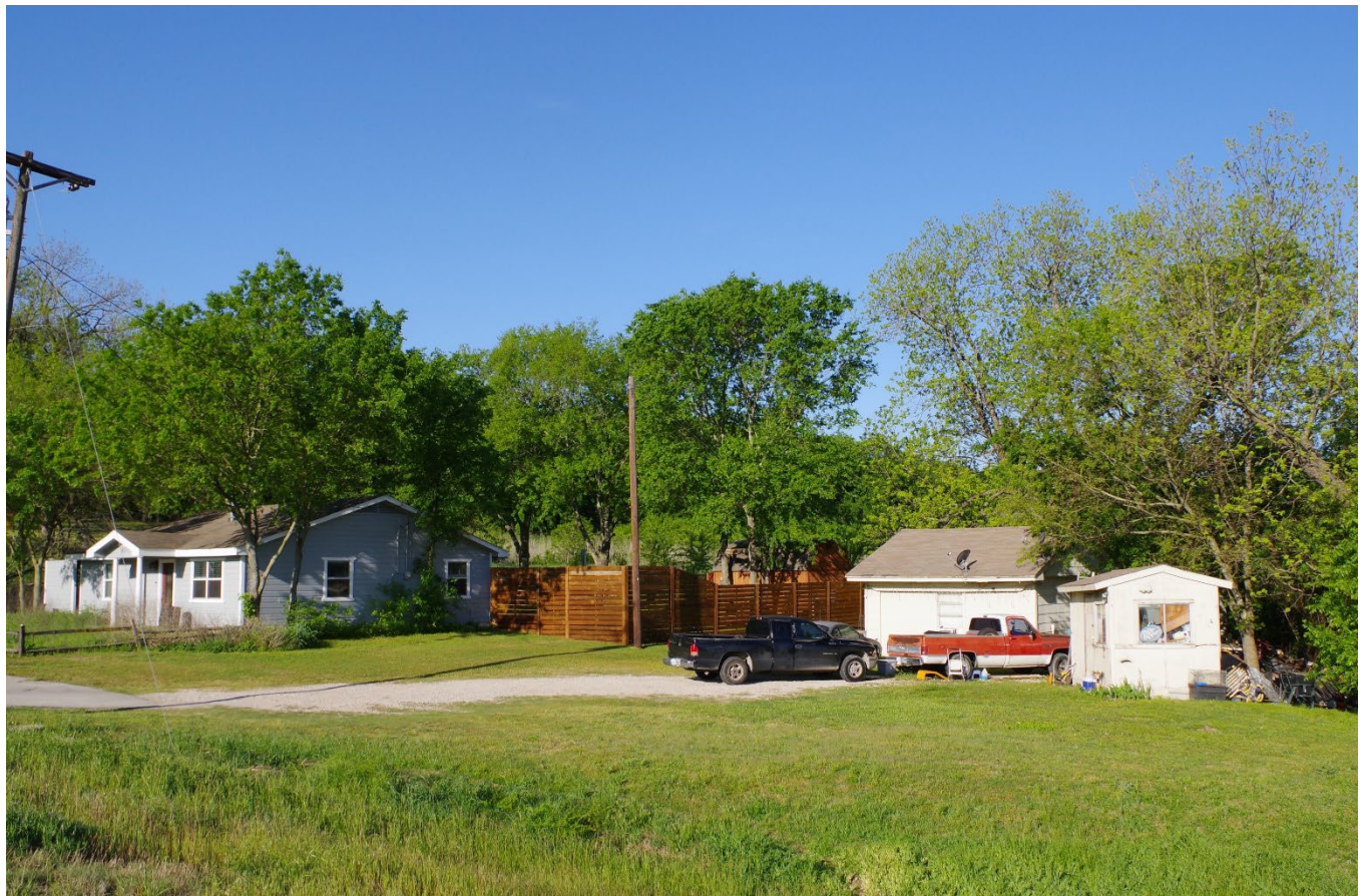
Overview of dwelling, former garage, and outbuilding/shed, camera facing southwest (May 2021)
