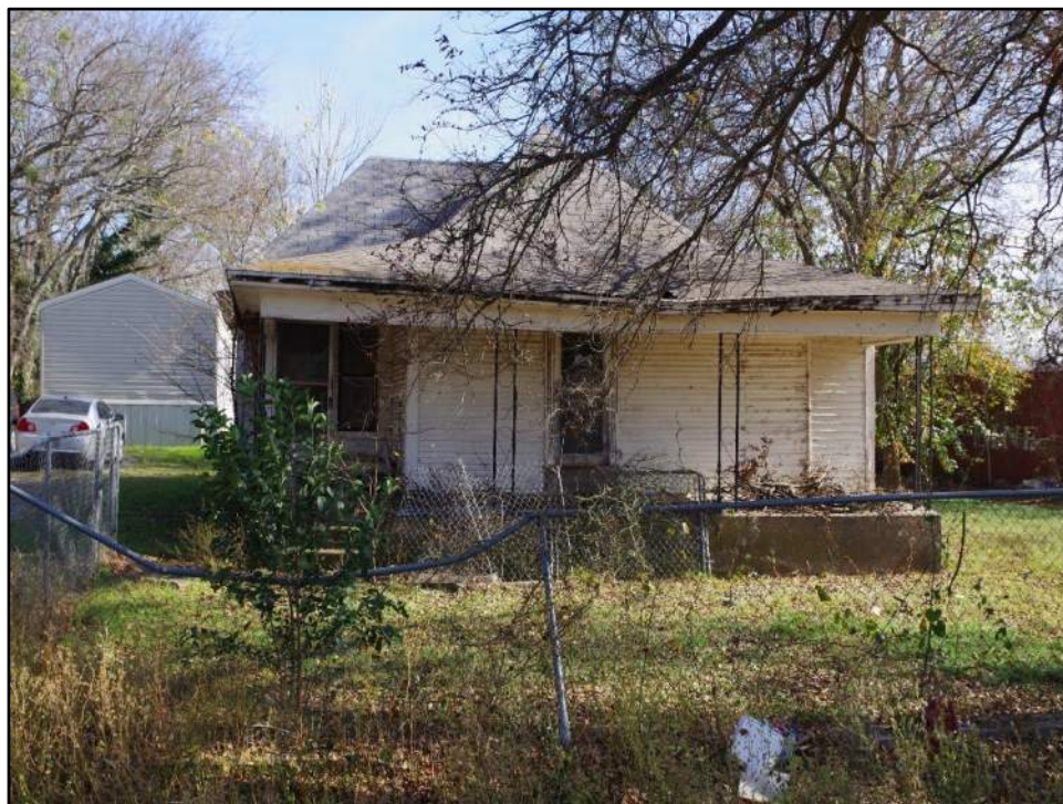
View of Resource 64, camera facing east.
