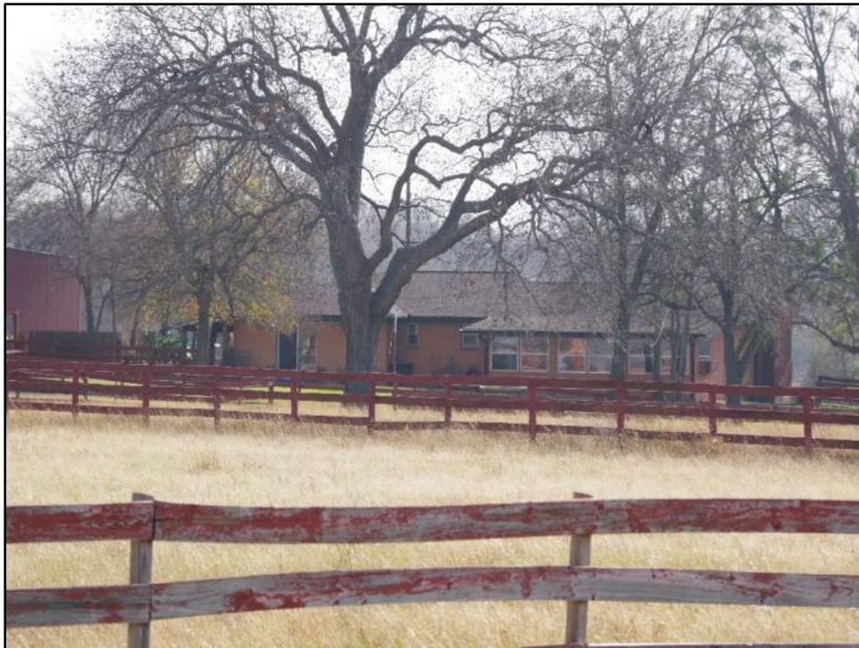
Photograph F-269: View of Resource 56a, camera facing east.
