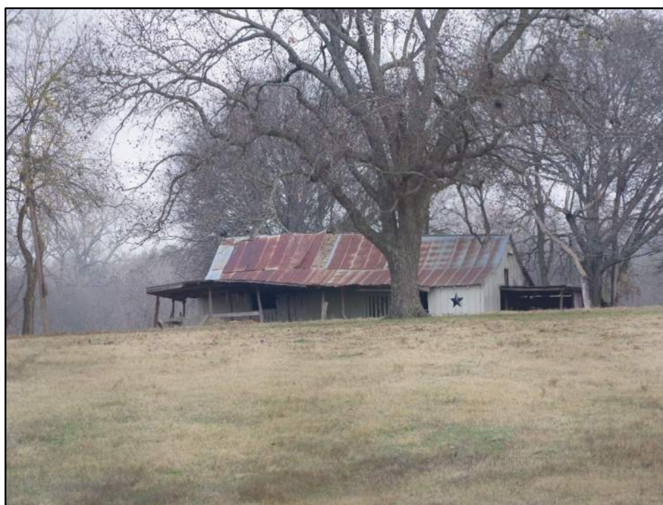
View of Resource 53b, camera facing north.
