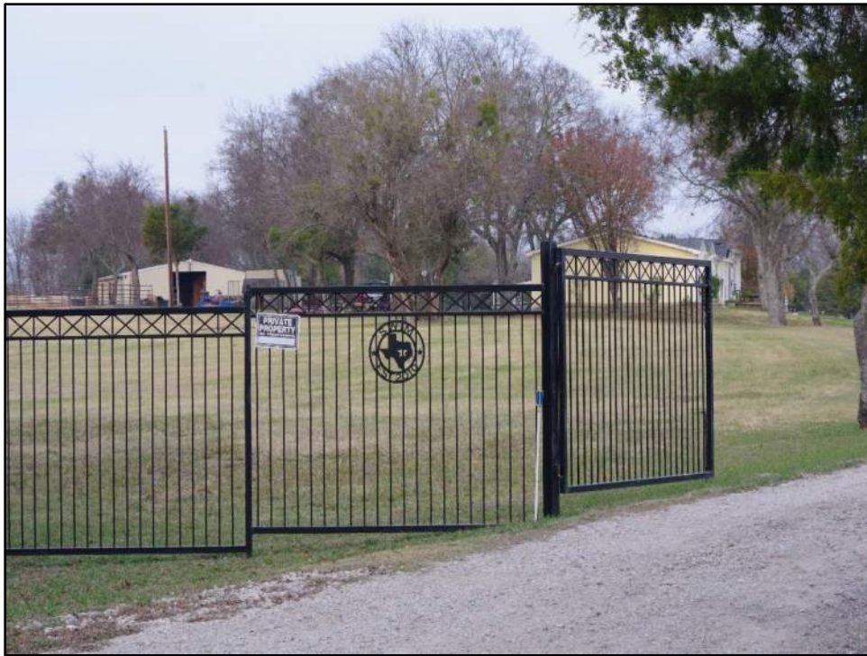
Photograph F-231: Overview of Resource 50, camera facing northeast.
