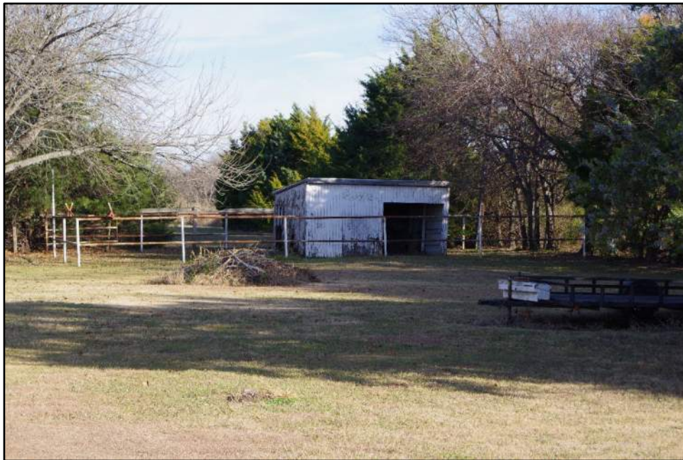
View of Resource 19c, camera facing northeast.
