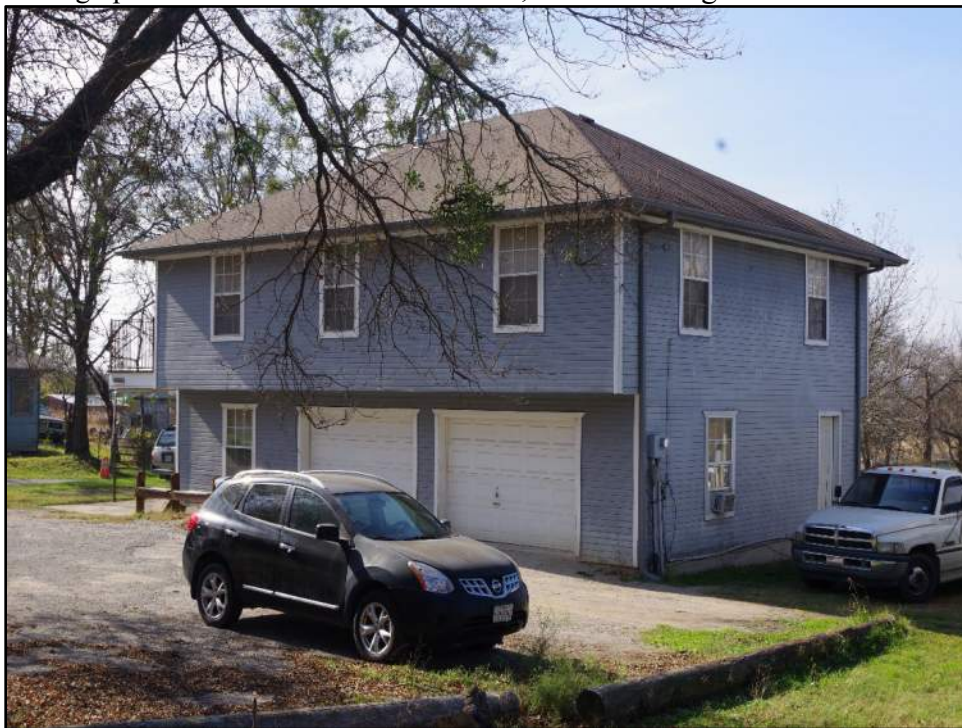
Photograph F-302: View of Resource 62b, camera facing southwest.
