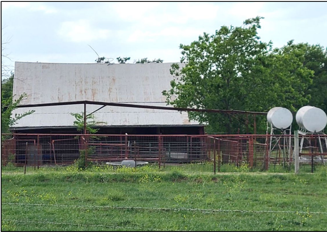
Photograph 9: View of 3187 FM 2933 barn, camera facing west (April 2023).
