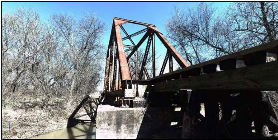
Photograph 15: Railroad Truss Bridge over East Fork Trinity River.
