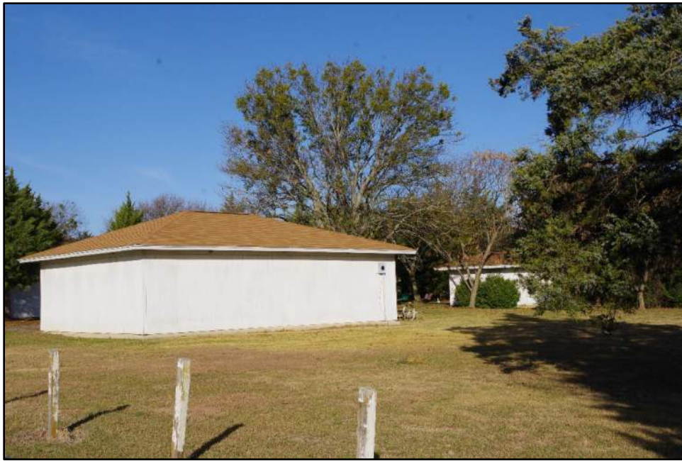
Photograph F-71: View of Resource 19b (background) and non-historic-age garage, camera facing northwest.
