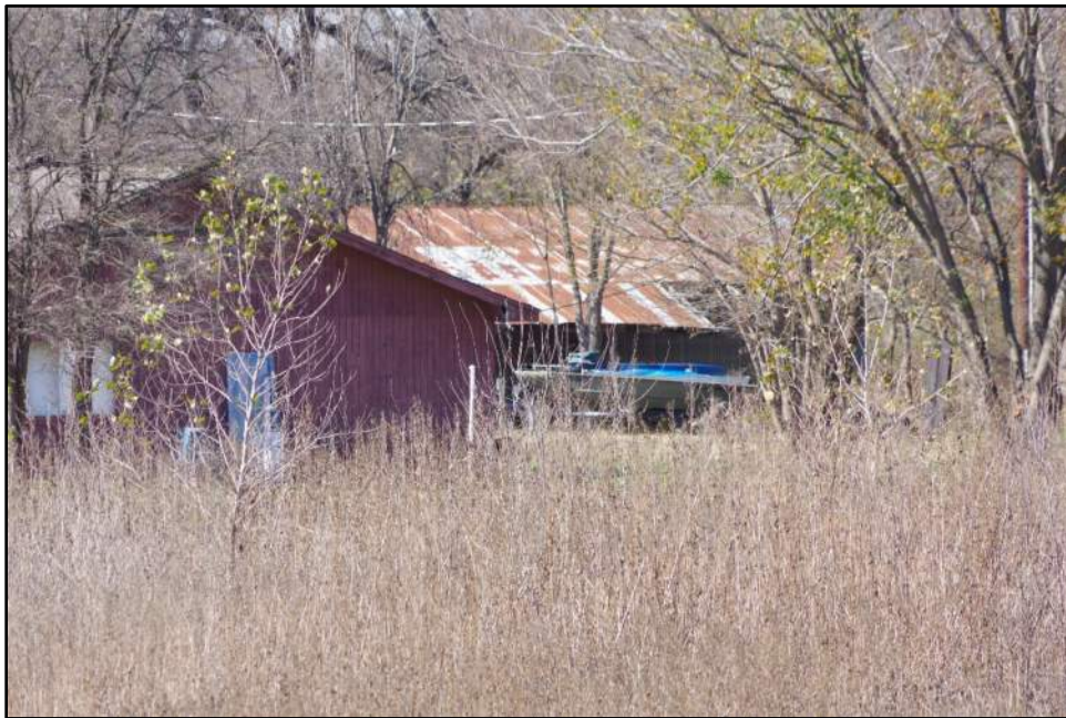
Photograph F-158: Obstructed view of Resource 32c, camera facing northwest.
