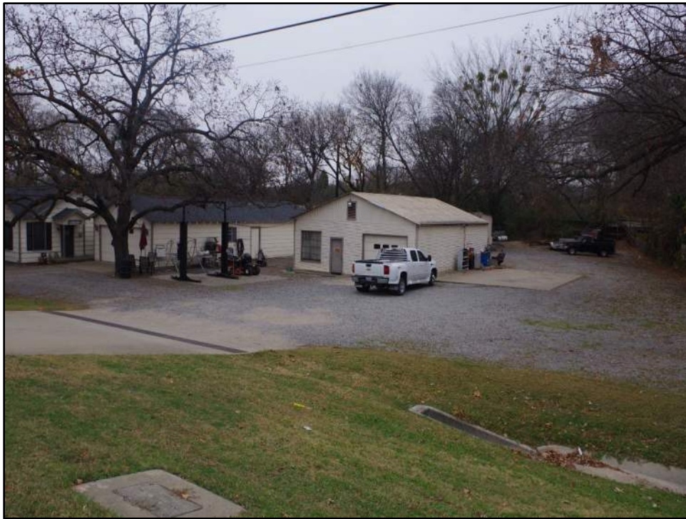
Photograph F-361: Overview of Resource 79, camera facing northwest.
