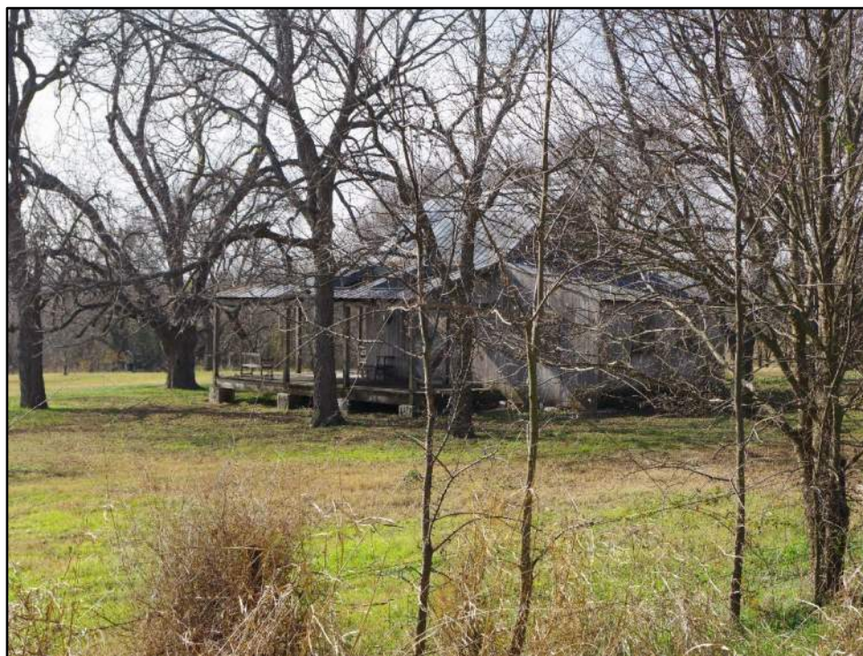
View of Resource 57a, camera facing northeast.
