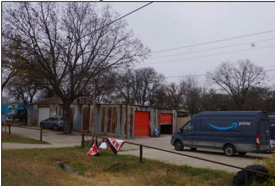
Photograph F-414: Overview of Resource 94, camera facing northwest.
