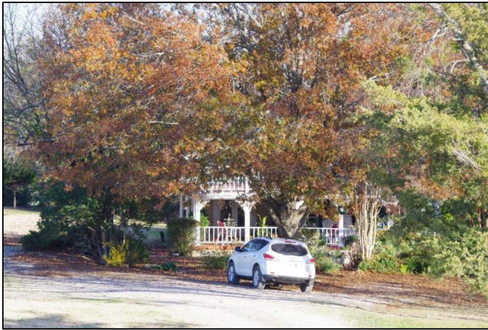
Photograph F-19: Obstructed view of Resource 06, camera facing east.
