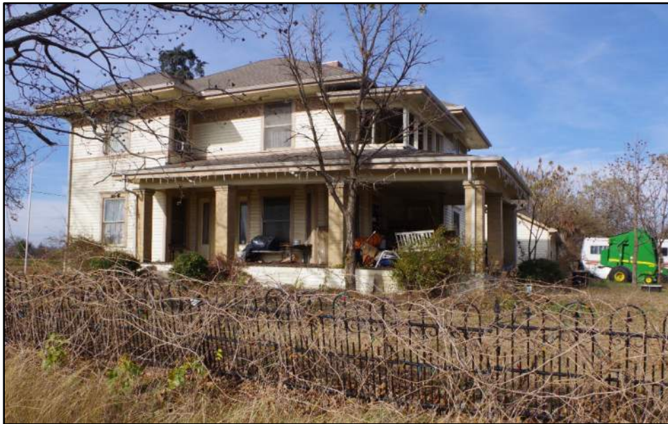
Photograph F-163: View of Resource 34a, camera facing north.
