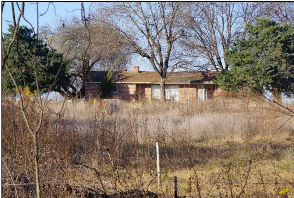
View of Resource 13a, camera facing north.
