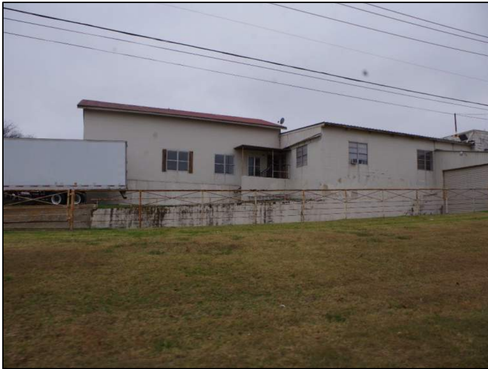
Photograph F-225: View of Resource 48, camera facing southwest.
