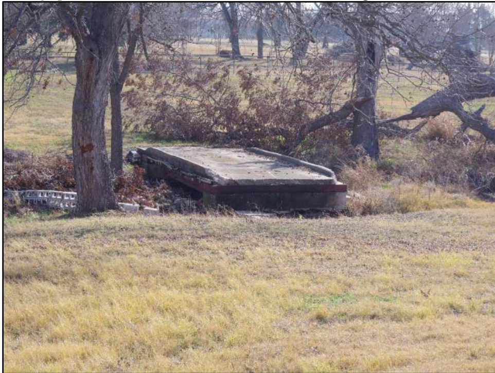
Photograph F-264: View of Resource 55b, camera facing east.
