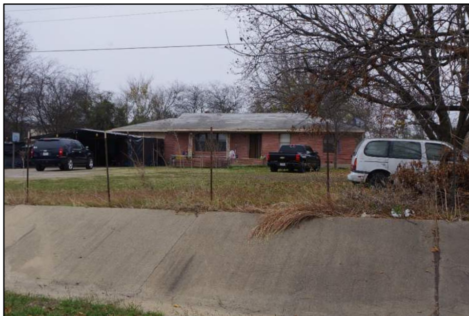
View of Resource 91a, camera facing north.
