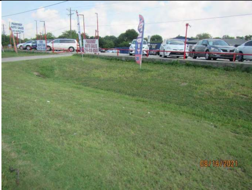
Photo 154. Photo of Ditch Drainage Feature Water Feature 345 in the eastern portion of the Environmental Footprint. Water Feature 345 was constructed in uplands to aid in the removal of stormwater from US 380. Note the upland vegetation throughout flow path, lack of a stream bed or banks, and adjacency to US 380. Photo is also representative of Water Feature 344, 349, 350, and 352 . Photo was taken to the north on August 16, 2021.
