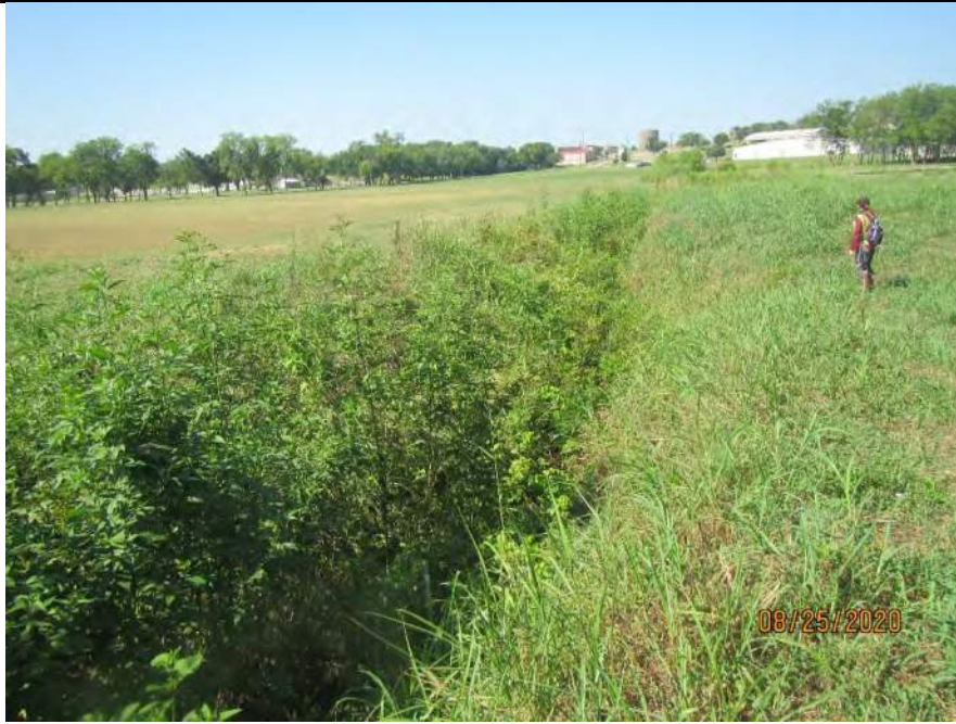
Photo 86. Photo of Ditch Drainage Feature Water Feature 183 in the central portion of the Environmental Footprint. Water Feature 183 was constructed within an agricultural field to assist in draining. Note the anthropogenic symmetry and upland vegetation covering the entire channel. Photo taken to the southwest on August 25, 2020.
