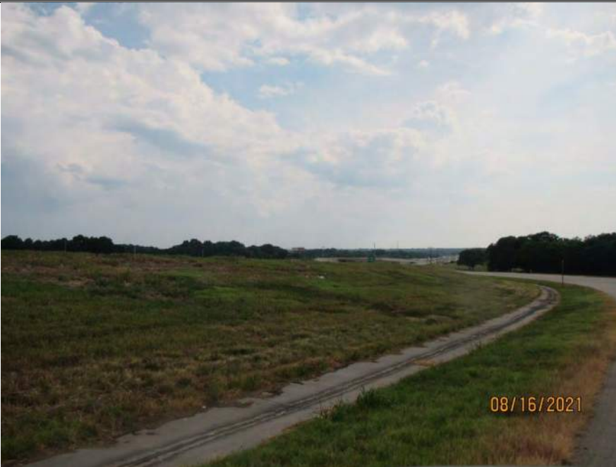
Photo 107. Photo of Ditch Drainage Feature Water Feature 214 in the central portion of the Environmental Footprint. Water Feature 214 is a concrete lined ditch and was constructed in uplands around the US 75 and SH 121 interchange to aid in the rapid removal of stormwater runoff from highways. Photo taken August 16, 2021.
