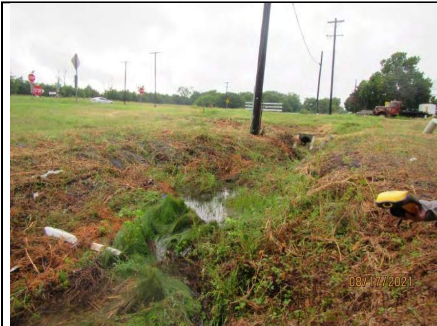
Photo 72. Photo of Ditch Drainage Feature Water Feature 159 in the central portion of the Environmental Footprint. Water Feature 159 was constructed in uplands to aid in the draining of stormwater from adjacent roads. Note the anthropogenic symmetry of the channel. Photo taken on August 17, 2021.
