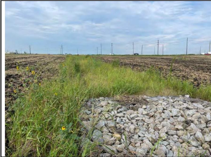
Photo 1. Photo of Ditch Drainage Feature Water Feature 1. Water Feature 1 was constructed within an agricultural field to assist in draining. Note the anthropogenic symmetry and upland vegetation covering the entire channel. Photo taken to the southwest on August 17, 2021.
