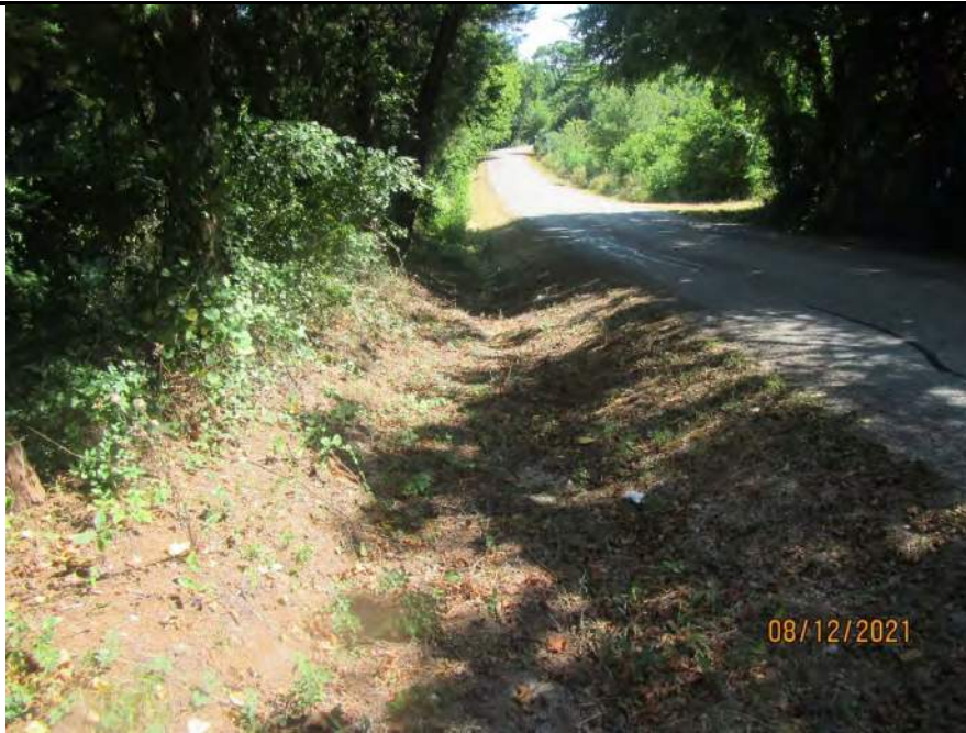
Photo 138. Photo of Ditch Drainage Feature Water Feature 308 in the eastern portion of the Environmental Footprint. Water Feature 308 was constructed in uplands to aid in the removal of stormwater runoff from the adjacent road. Note the upland vegetation in the hydrological flow path, as well as the lack of a stream bed or banks. Photo is also representative of Water Feature 303 and 306 and was taken August 12, 2021.
