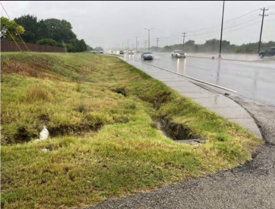
Photo 13. Photo of Ditch Drainage Feature Water Feature 27 in the western portion of the Environmental Footprint adjacent to US 380. Water Feature 27 was constructed in uplands and contained a section of scour. Photo taken to the west on August 17, 2021. Photo is representative of Ditch Drainage Features Water Feature 9, 28, 34, 36, 38, 39, 40, 41, 42, 43, 47, 48, 55, 56, 57, 60, 67, 68, 73, 74, 86, 90, 93, 95, 96, 324, and 326.
