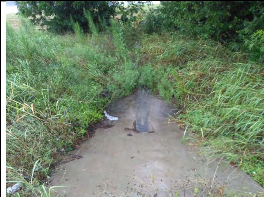
Photo 32. Photo of Swale Drainage Feature Water Feature 71 located in the western portion of the Environmental Footprint. Photo representative of Swale Drainage Feature Water Feature 348 . Water Feature 71 received its hydrology from the runoff of adjacent parking lots fed underground through a culvert. Note the lack of an OHWM, hydrophytic vegetation, hydric soils, hydrological indicators, stream bed, or banks within the area. Photo was taken to the south on August 18, 2021, after a heavy rainfall event.
