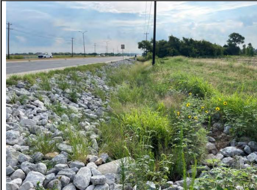
Photo 2. Photo of Ditch Drainage Feature Water Feature 2. Water Feature 2 was constructed in uplands to assist in the rapid removal of water from US 380. Photo was taken to the east on August 17, 2021.
