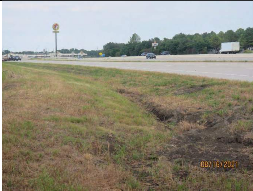
Photo 104. Representative photo of Ditch Drainage Features Water Features 208, 210, 211, 213, and 217 in the north central portion of the Environmental Footprint. These roadside ditches were constructed in uplands around the US 75 and SH 121 interchange to aid in the rapid removal of stormwater runoff from highways. Photo taken August 16, 2021.
