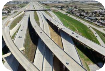
TxDOT DFW Connector $1.5B Dallas, TX
