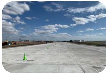
DFW Airport NE End Around Taxiway $47M Irving, TX
