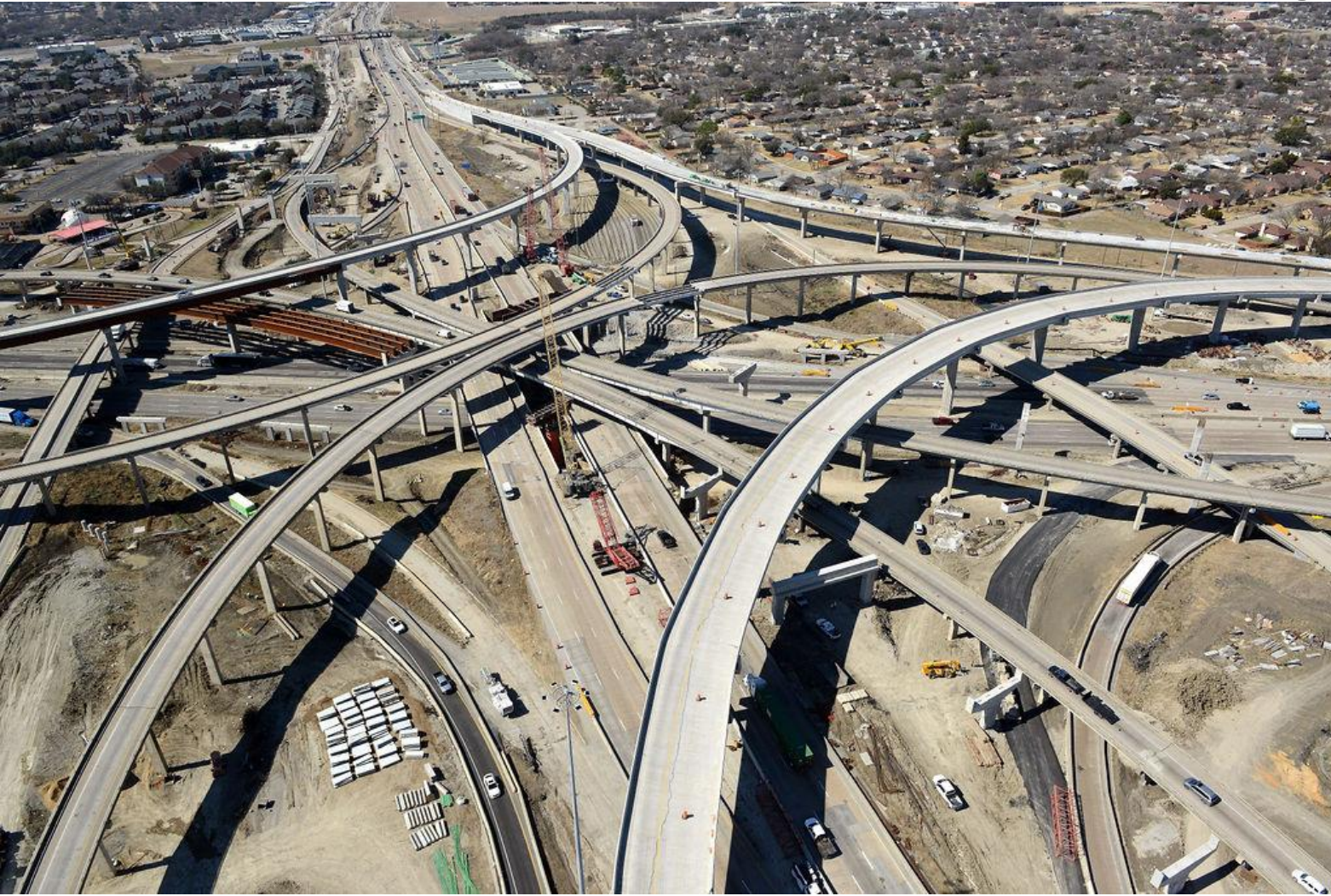
TxDOT Dallas LBJ East OVTI at I-635/I-30 Interchange
