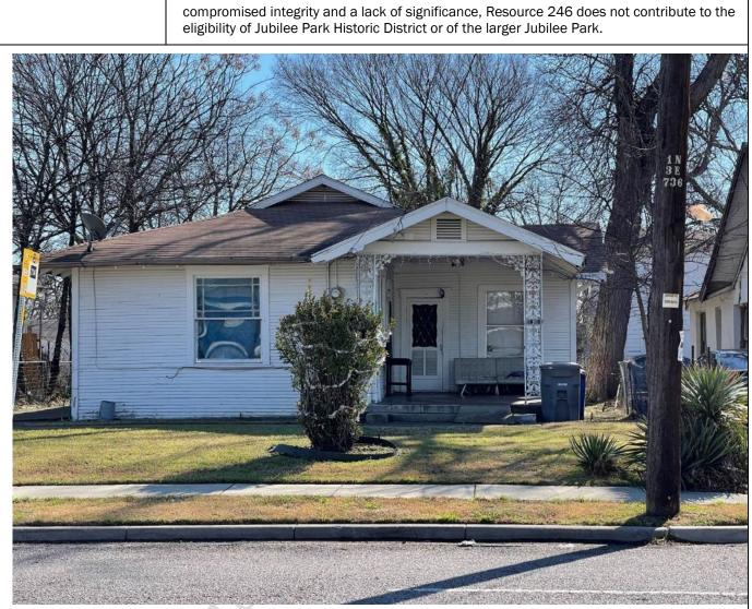
Resource 246 (HHM) [25b (HNTB)]: view of façade (northwest elevation) showing plastic replacement glazing and replacement porch supports
