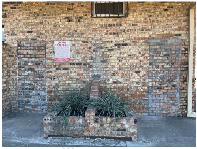
Resource 346 (HHM) [51 (HNTB)]: view of northeast elevation showing bricked-in door openings and planters
