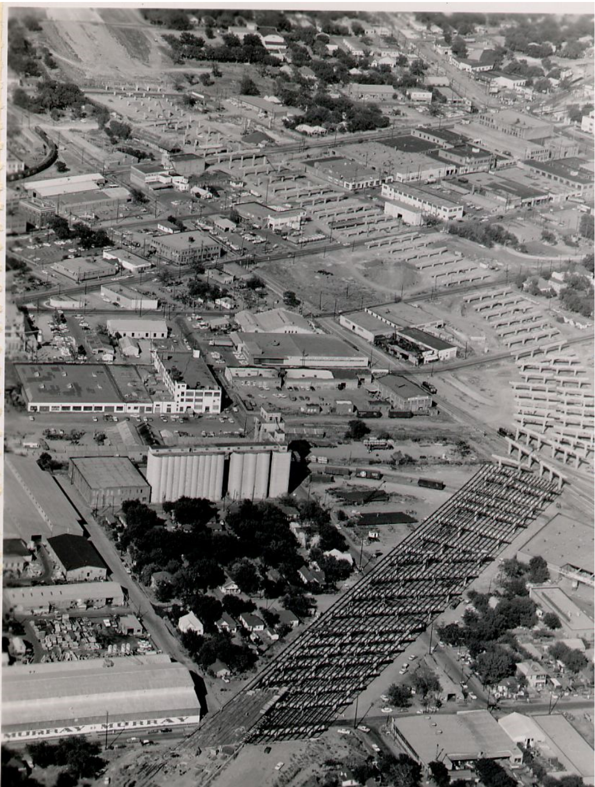
Figure 84. Construction of IH 30 in the 1960s past the Pearlstone Mill in Deep Ellum. Source: Texas Freeway, accessed February 23, 2023, i20 dallas undated elevated eastdallas.jpg (885x1084) (texasfreeway.com) .
