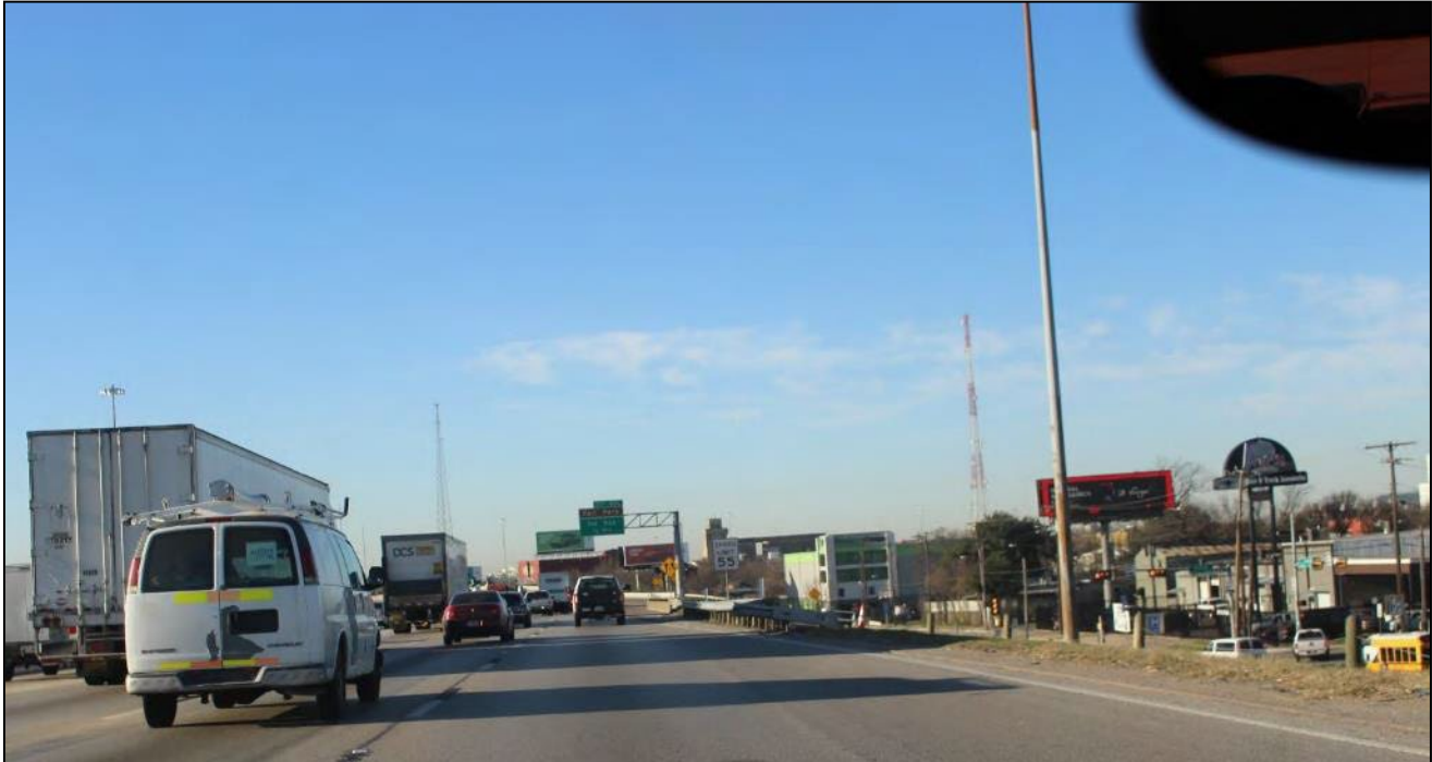
Photo 2: I-30 near exit 47 C – Camera facing southwest
