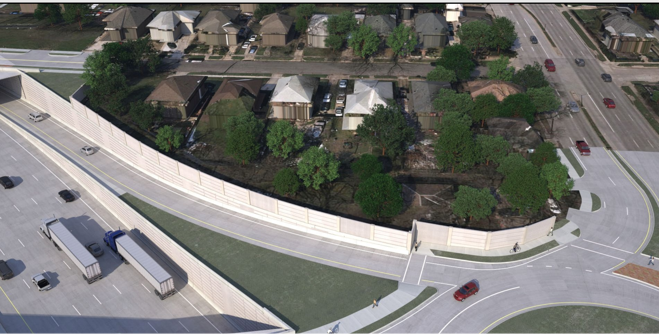
B) Birdseye View – Front of Noise Wall
