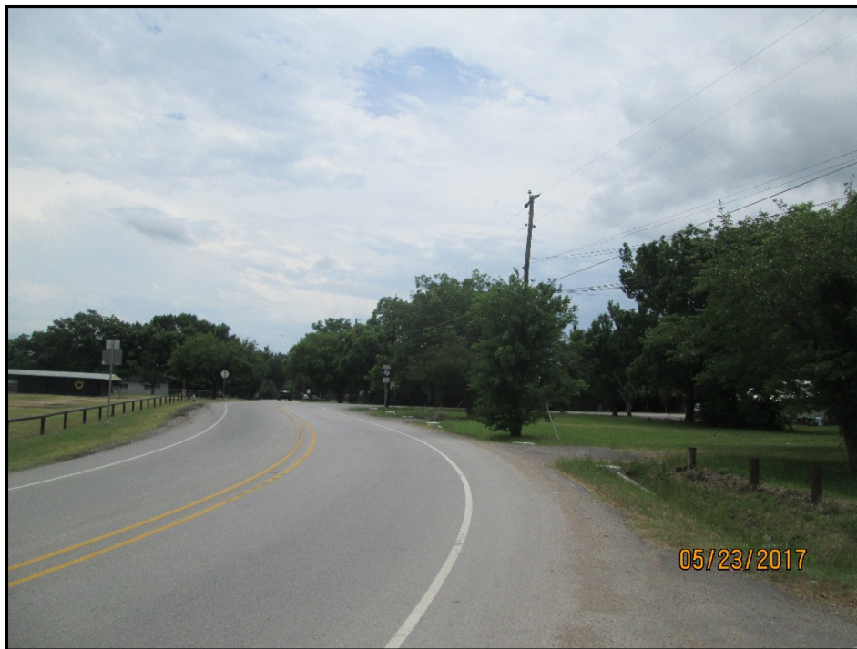
Photograph 2: View of the existing FM 148 roadway from the downtown Crandall area headed towards US 175.
