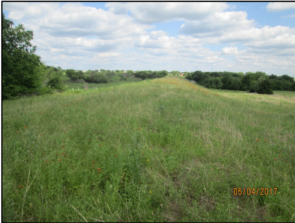
Photograph 4: View of a floodwater control impoundment associated with the Natural Resource Conservation Service (NRCS) easement adjacent to FM 148. View is to the southeast.
