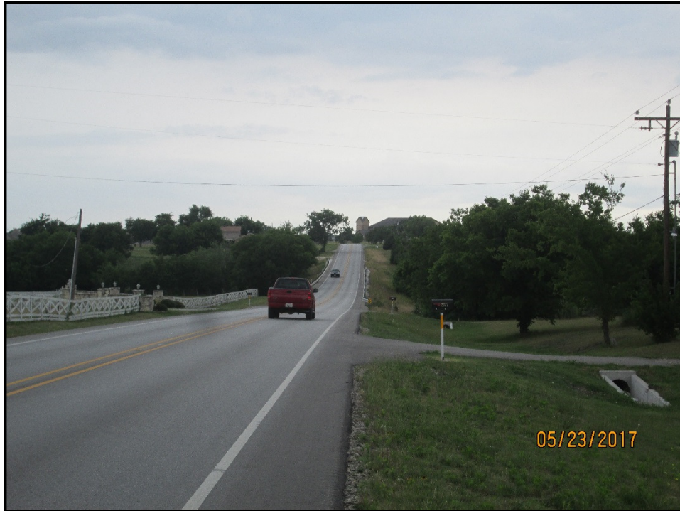
Photograph 3: View of the existing FM 148 roadway at the southern project terminus. View is to the northwest.
