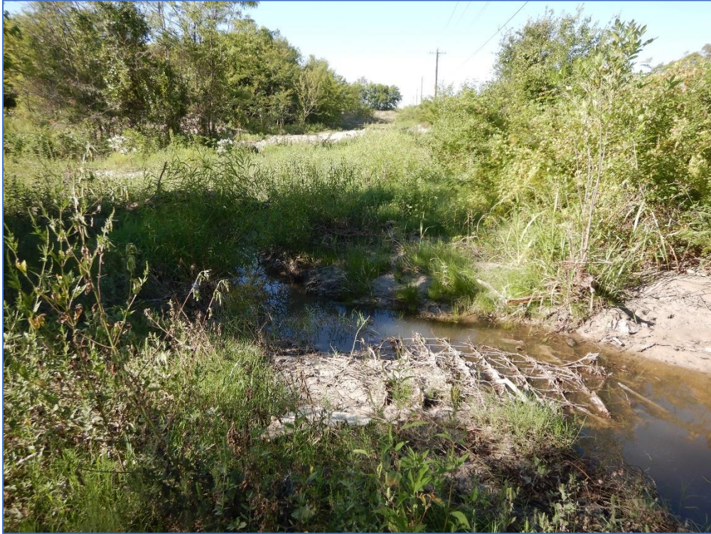
Photo 29. Shallow drainage on east side of FM 741 by Hometown Blvd; view southwest.
