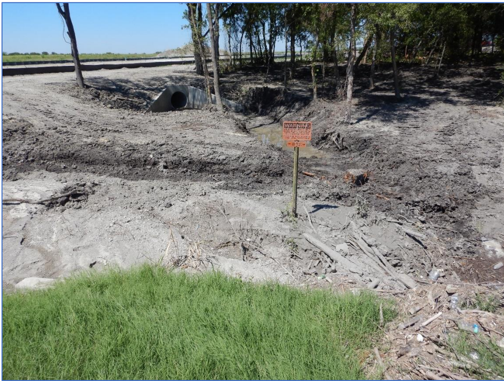
Photo 30. Reworked drainage on west side of FM 741 by Hometown Blvd; view northwest.
