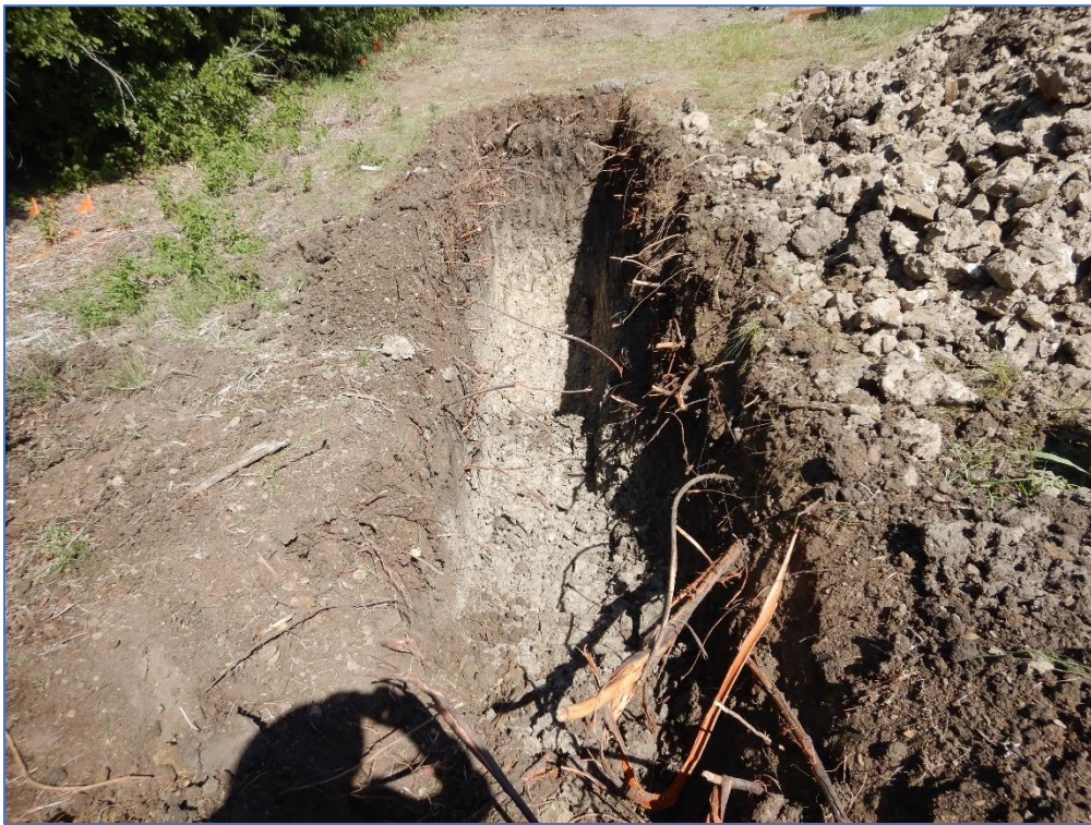
Photo 40. View of BT 2 from the south end; view north
