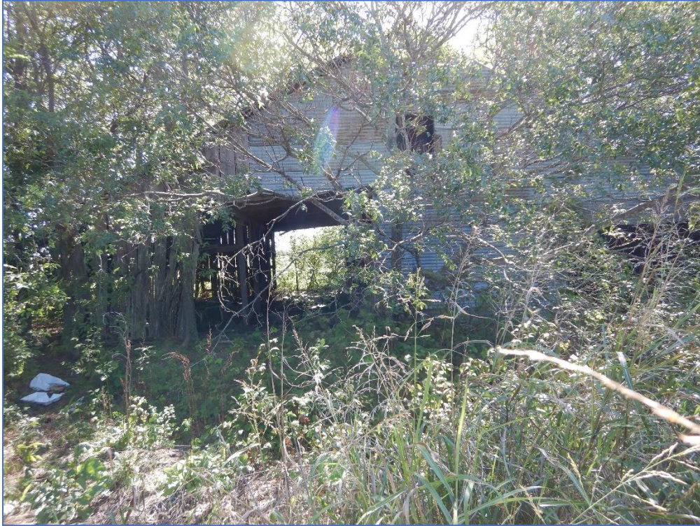
Photo 49. Front view of barn at site 41KF236; view southwest.
