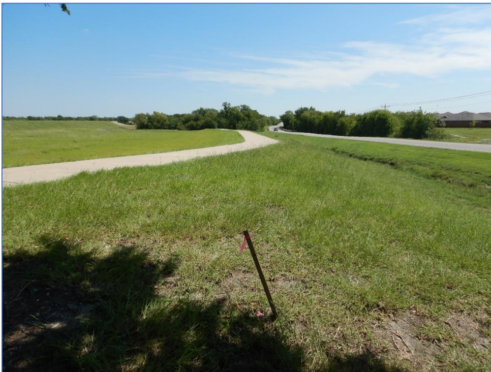
Photo 36. Disturbance from levees on north bank of drainage north of Griffin Lane; view southeast.
