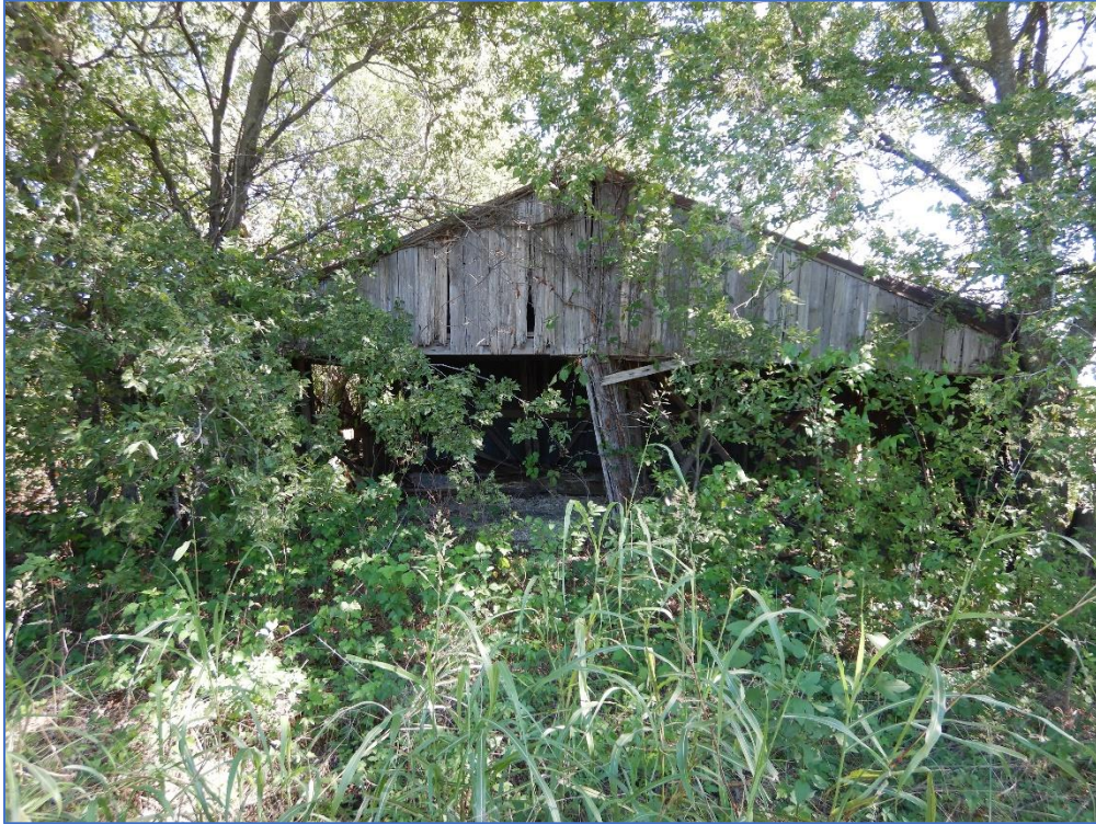
Photo 51. Front view of two car garage at site 41KF236; view northeast.
