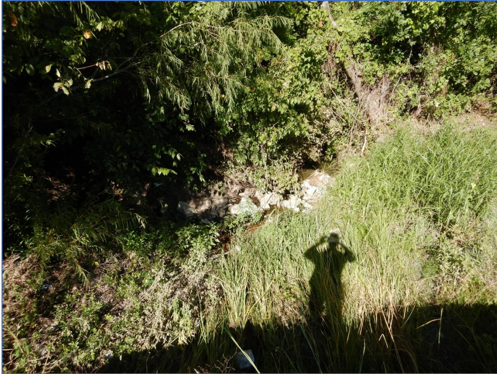
Photo 35. South bank of small drainage north of Griffin Lane; view northeast.
