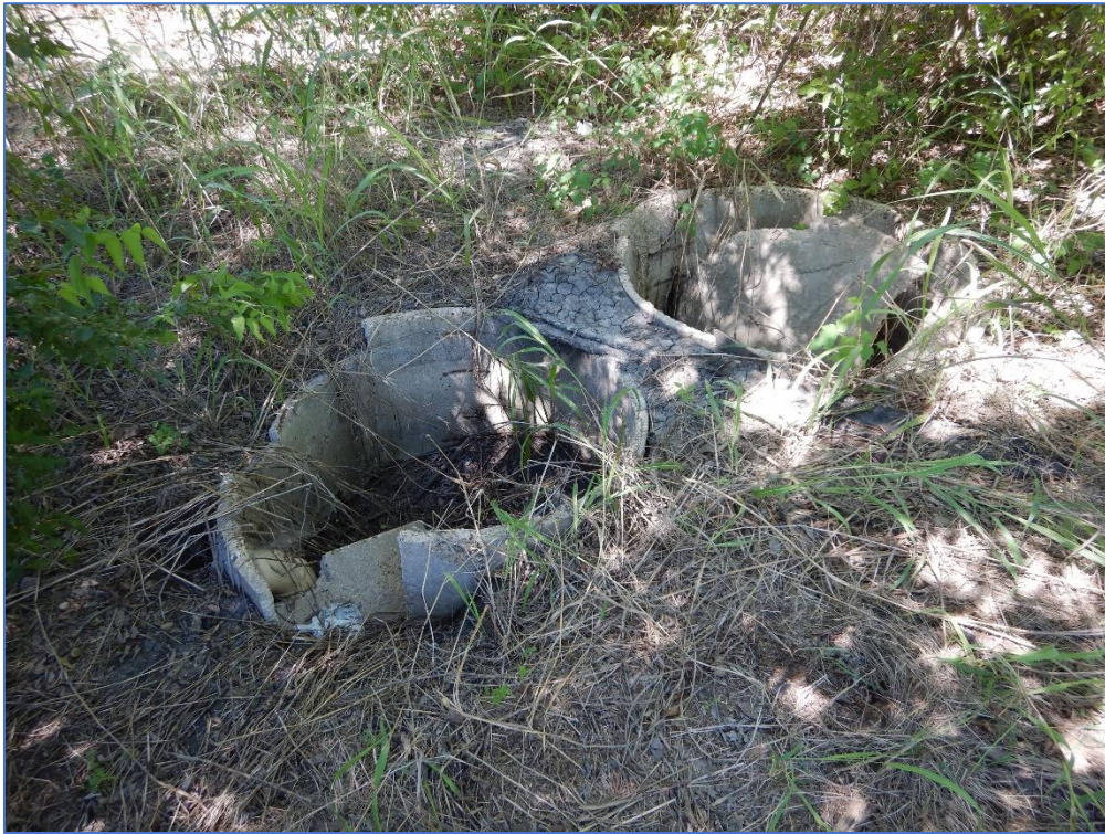
Photo 52. Concrete septic tanks at site 41KF236; view north.
