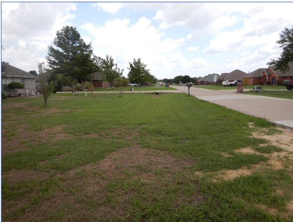
Photo 6. Residential and drainage ditch disturbance on County View Lane; view northwest.
