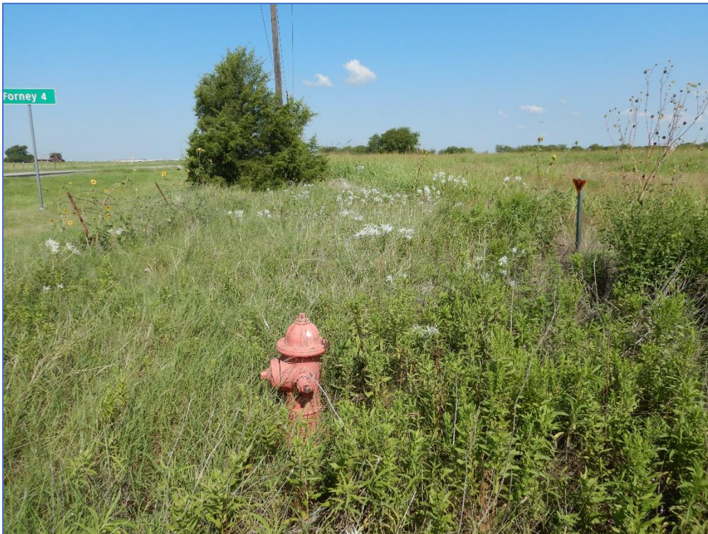
Photo 20. Water line disturbance in ROW by Precinct Circle; view northwest.
