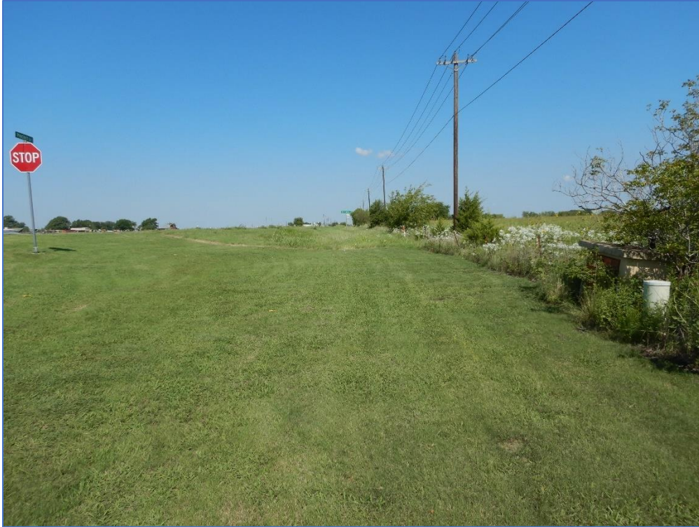
Photo 19. Disturbance from existing utilities within the ROW by Precinct Circle; view northwest.
