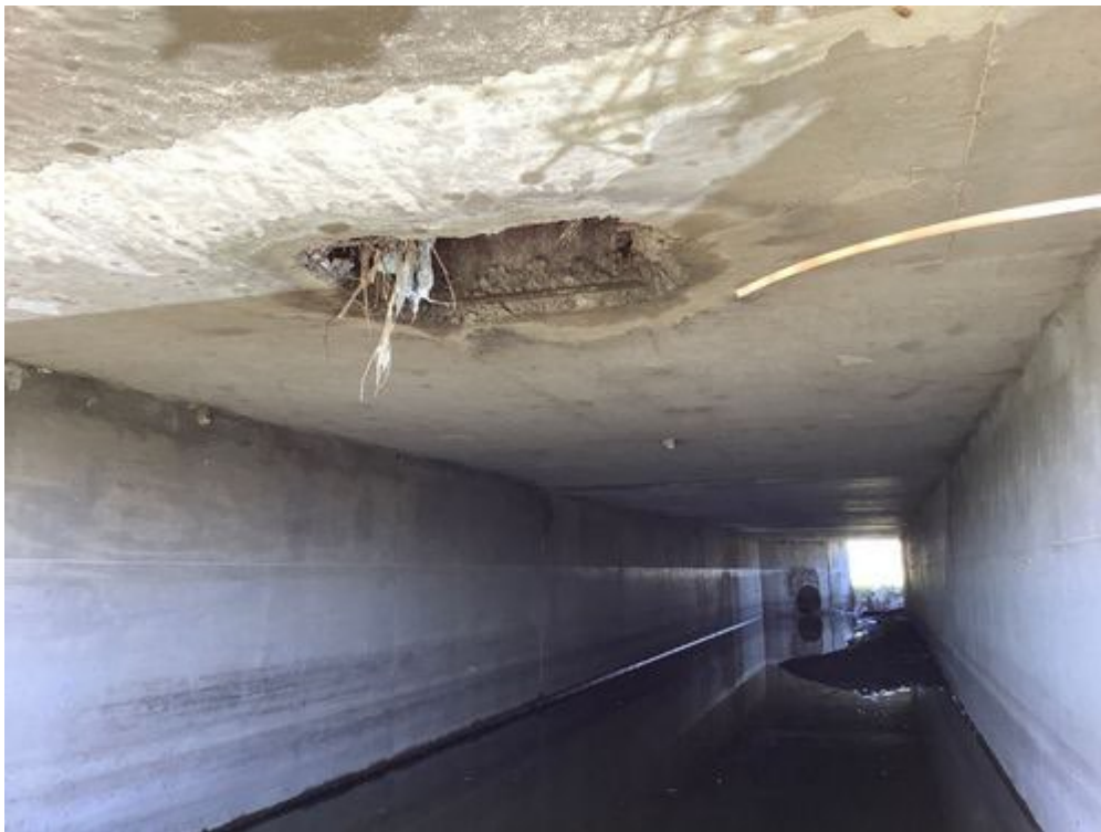
Photo 28: Crevice in a concrete box culvert that could potentially provide moderate roosting habitat for bat species.
