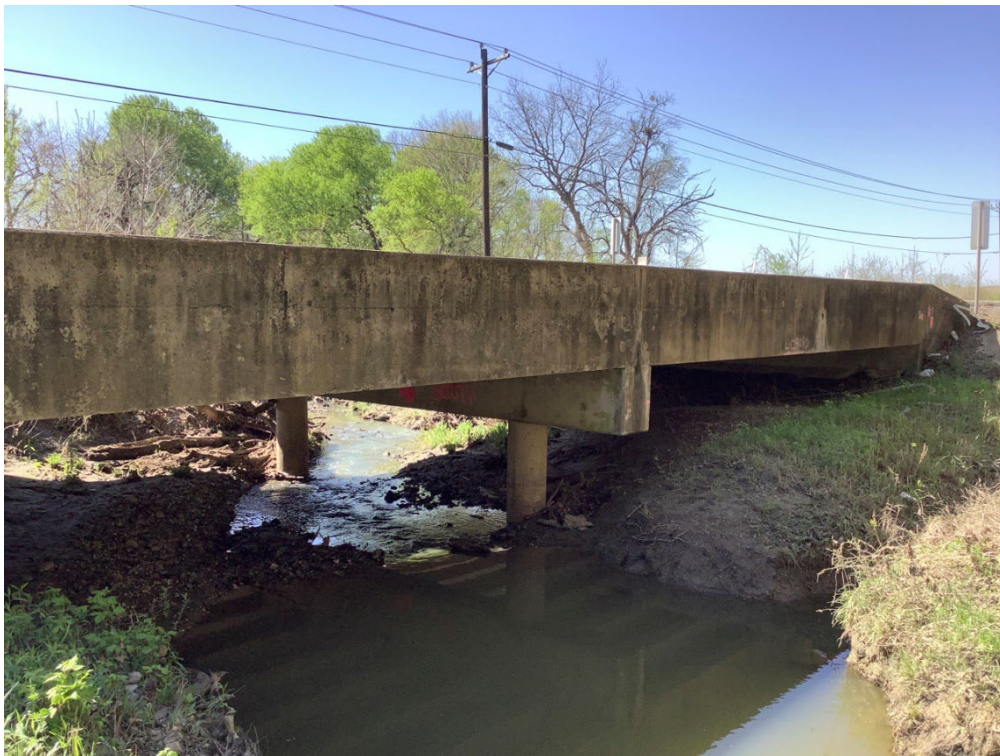
Photo 073: Water 3 (Unnamed tributary to Buffalo Creek) at the FM 741 bridge – Perennial stream.
