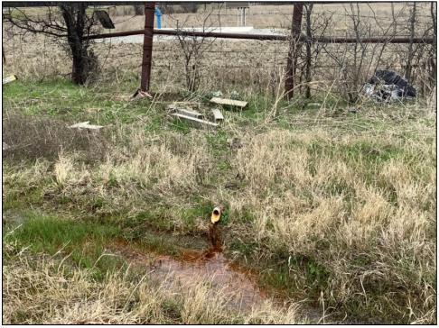
Photo 16: View of a drainage pipe observed during the site survey. The pipe is discharging discolored water with an oily sheen. The source of the discharge is unknown. This location is considered a low risk for the project.
