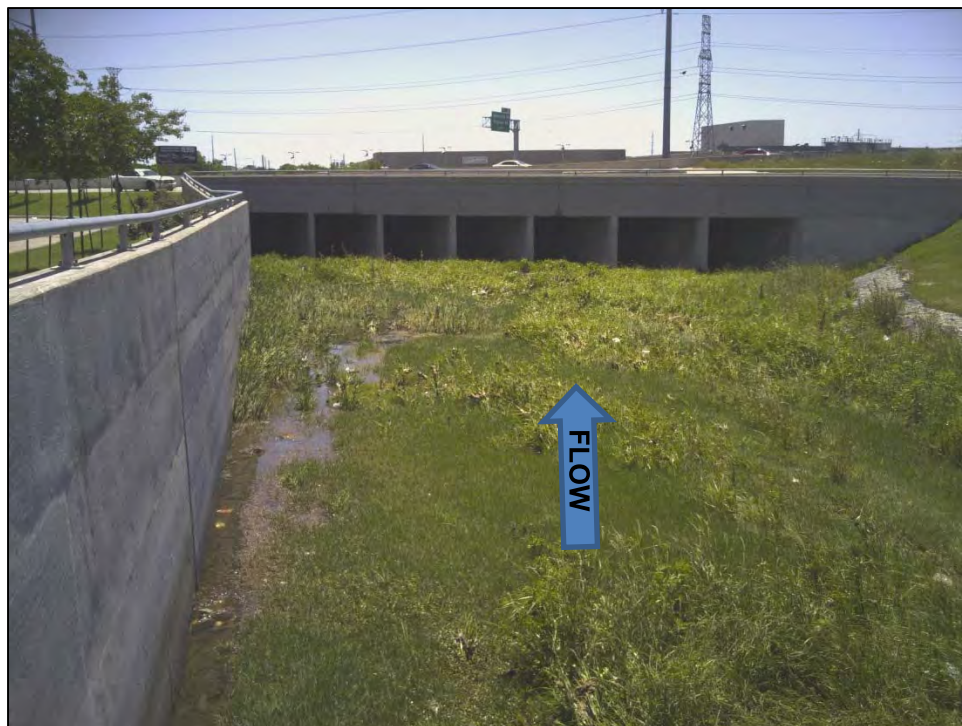
Photograph 21: Representative view of Long Branch crossing #1 downstream of Northwest Highway progressing to box culvert under IH 635 service road. This segment is lined by articulated concrete blocks. View is to the south.
