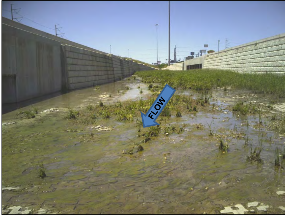
Photograph 22: Representative view of Long Branch crossing #1 downstream of IH 635 service road progressing to box culvert under IH 635. This segment is lined by articulated concrete blocks. View is to the northwest.
