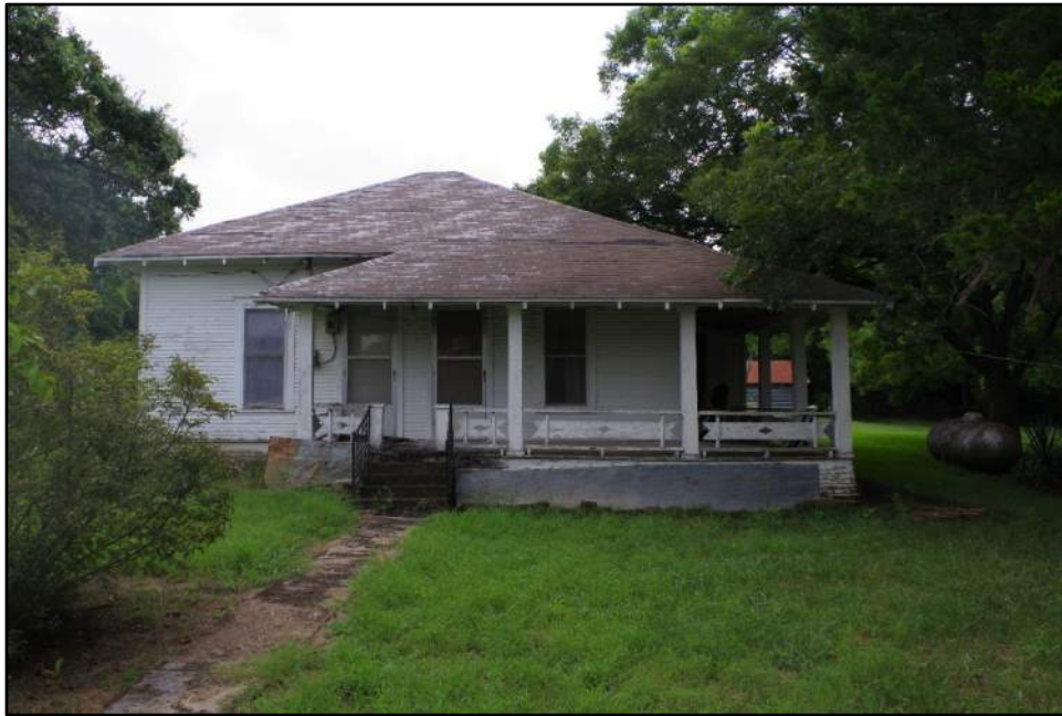
View of Resource 37a, camera facing north.
