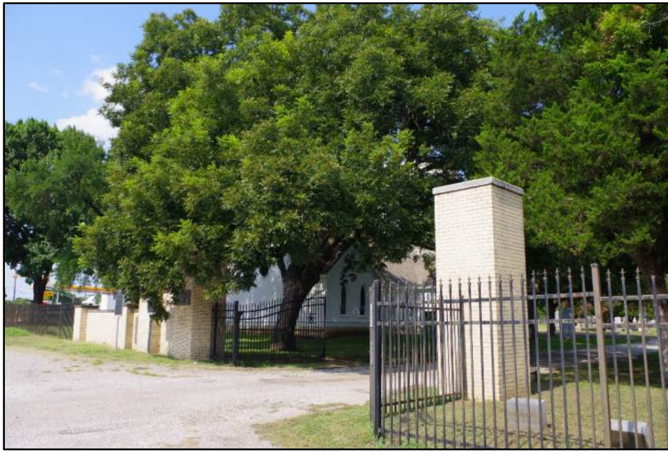
Photograph F-57: View of entrance gates to Resource 18 (Pecan Grove Cemetery), camera facing northeast.
