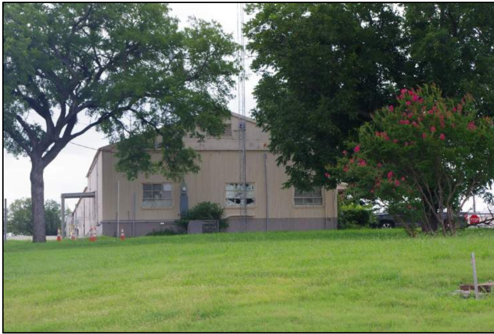
Photograph F-81: View of Resource 22a, camera facing east.
