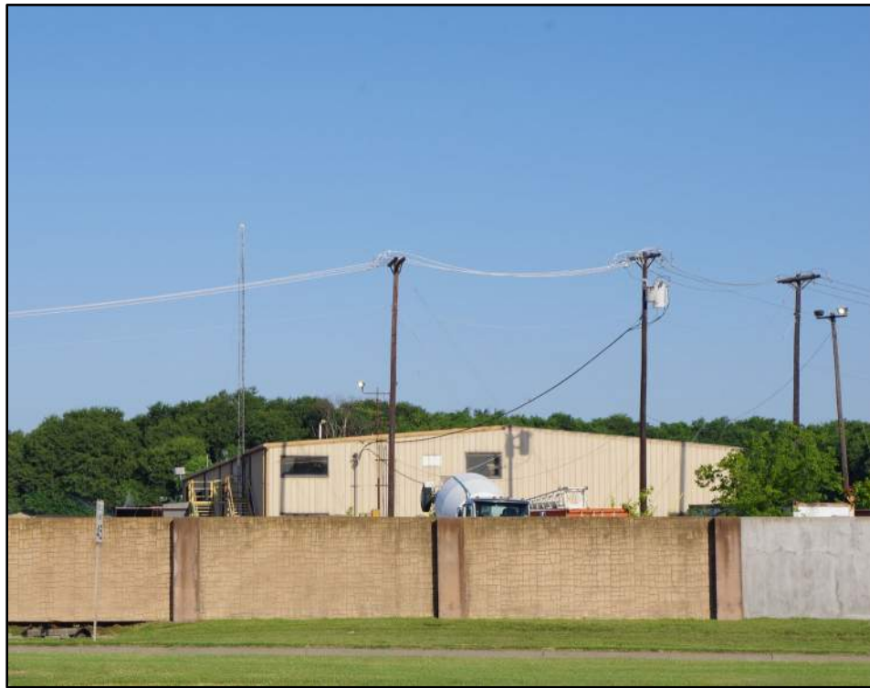
Photograph F-6: View of non-historic-age building associated with Resource 01, camera facing west.
