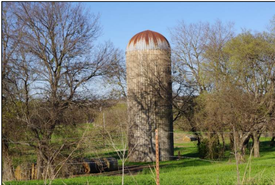
View of Resource 07b, camera facing north.
