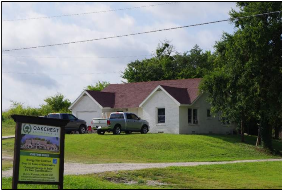
Photograph F-179: Obstructed view of Resource 47, camera facing southeast.
