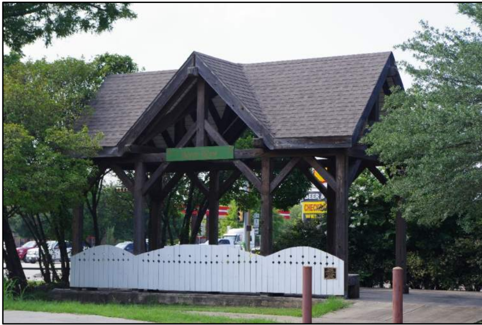
Photograph F-67: View of non-historic-age pavilion associated with Resource 18 (Pecan Grove Cemetery), camera facing northwest.
