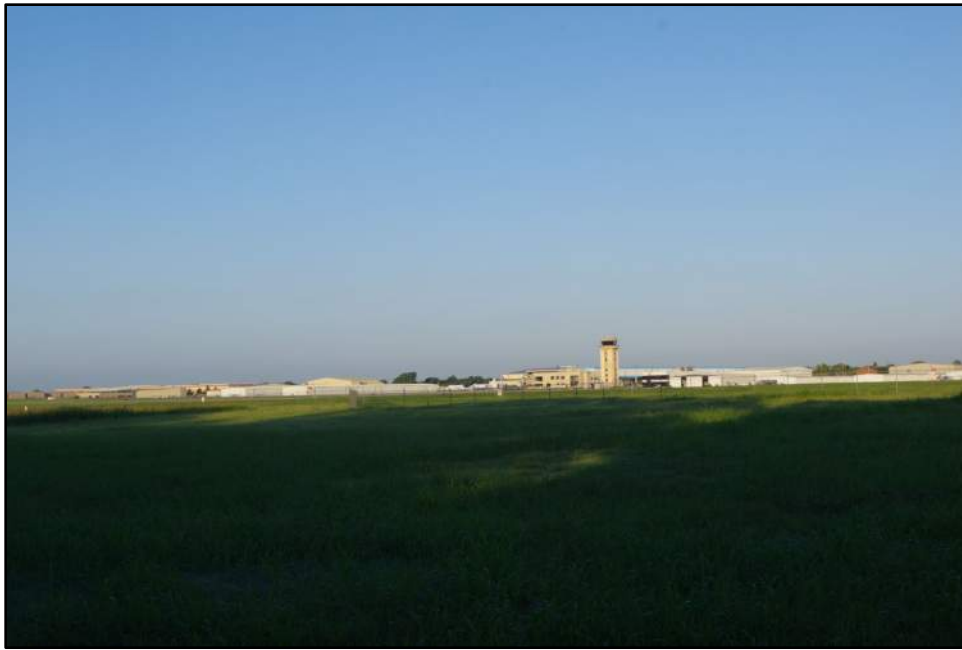
Photograph F-187: Rural Historic Landscape Evaluation Photo Point 03, view from FM 722 (Enloe Road) toward McKinney National Airport, camera facing southwest.
