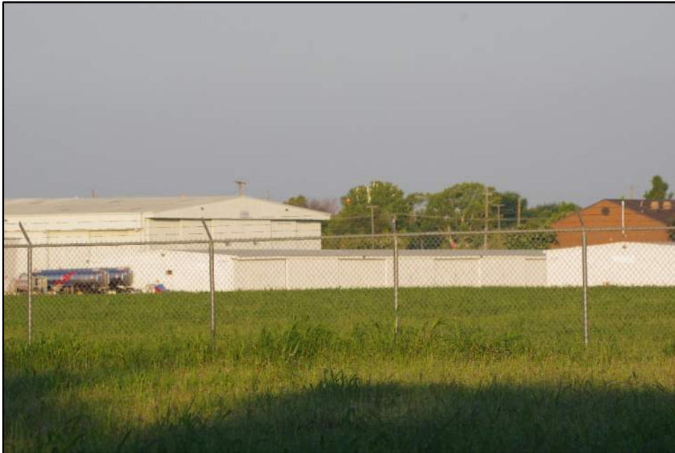
Obstructed view of Resource 09a, camera facing west.
