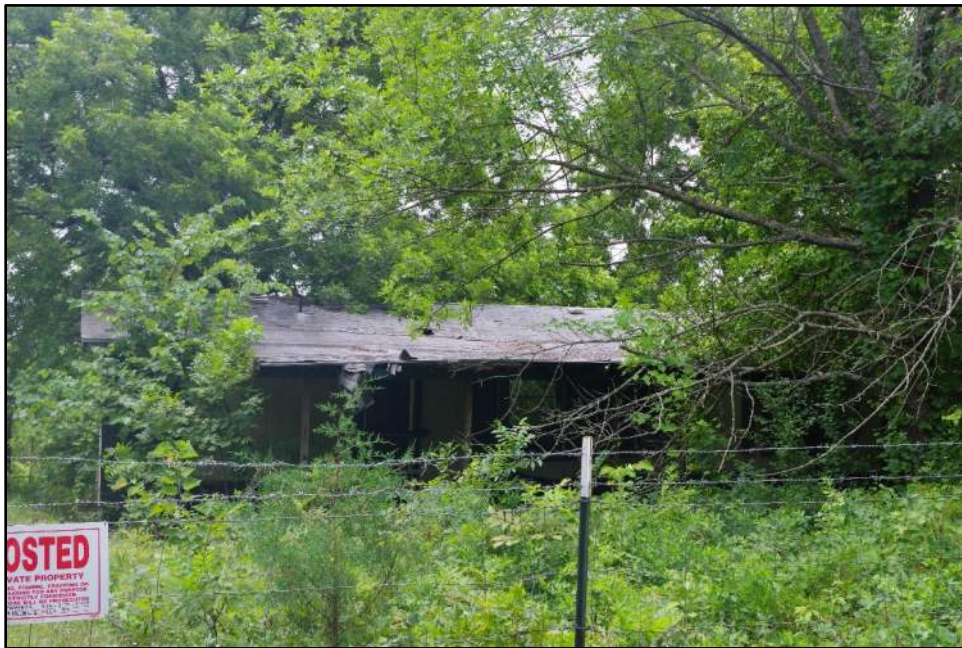
Photograph F-104: View of Resource 31b, camera facing southwest.
