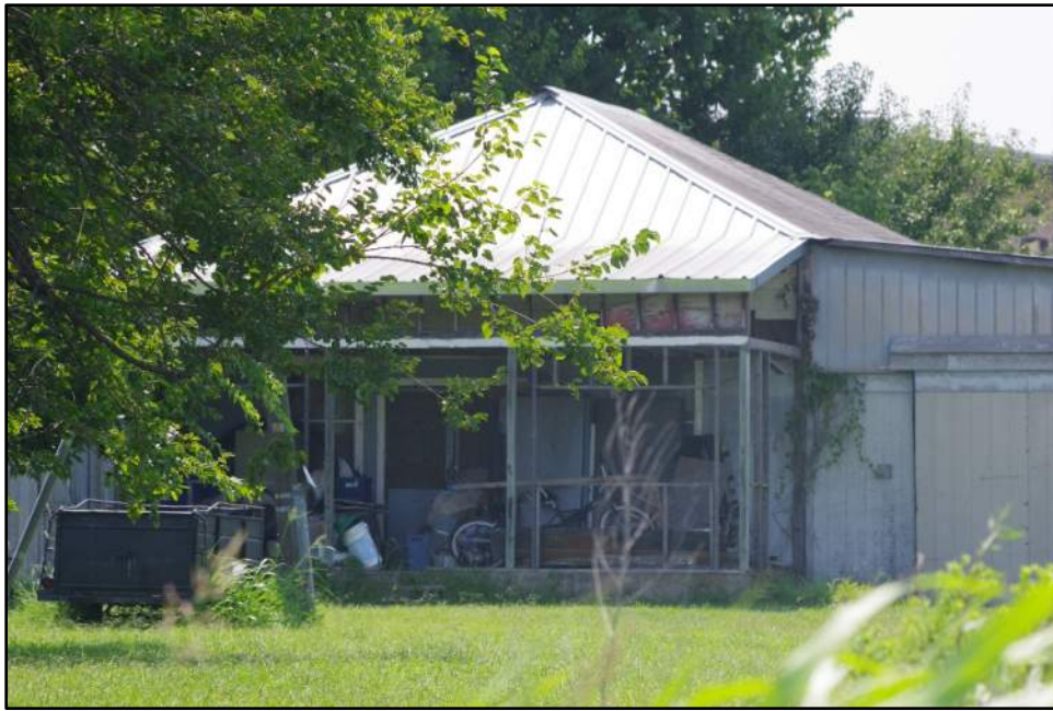
Photograph F-37: View of Resource 11b, camera facing southwest.
