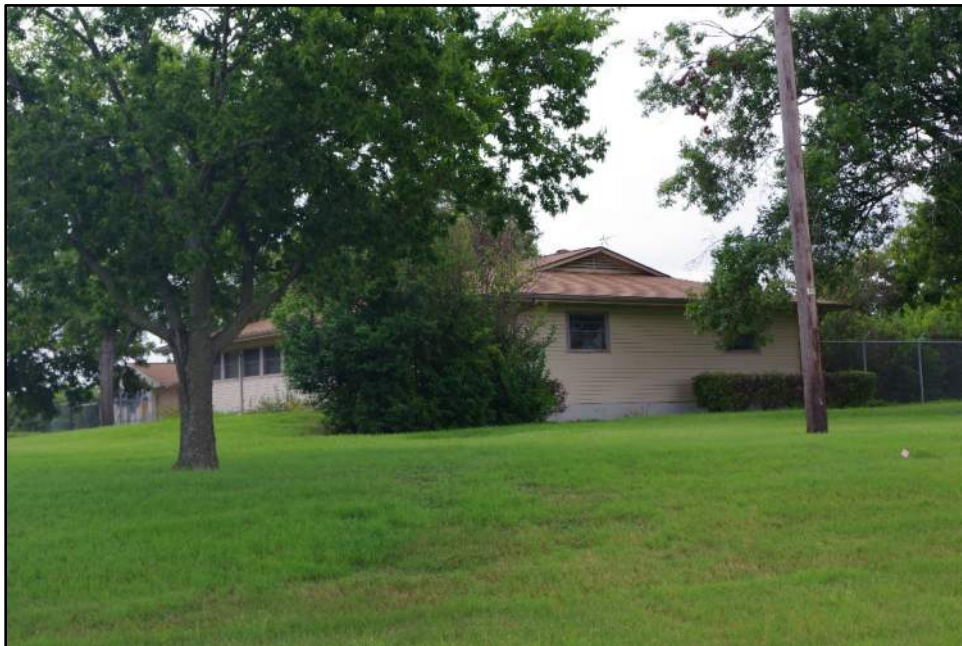
Photograph F-82: View of Resource 22b, camera facing southeast.
