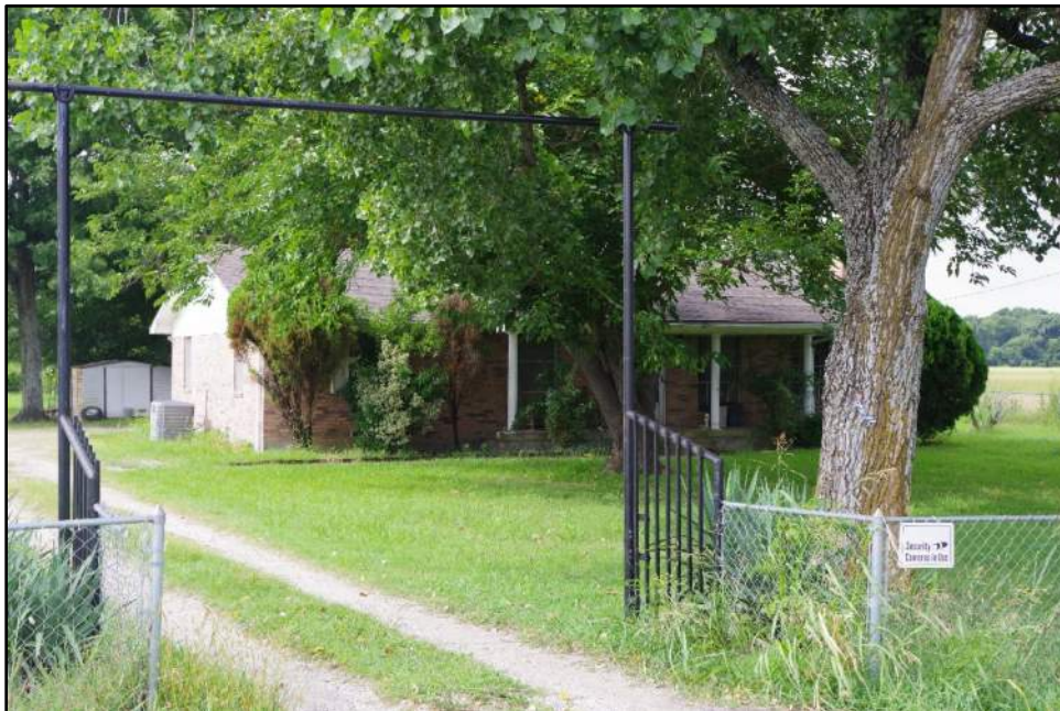
Photograph F-144: View of Resource 39, camera facing southwest.
