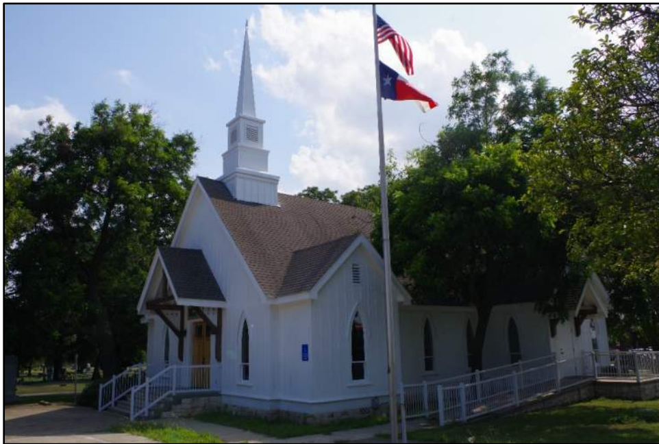
Photograph F-66: View of non-historic-age chapel associated with Resource 18 (Pecan Grove Cemetery), camera facing southwest.
