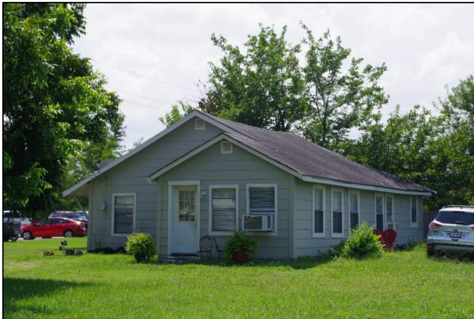
View of Resource 11a, camera facing southwest.
