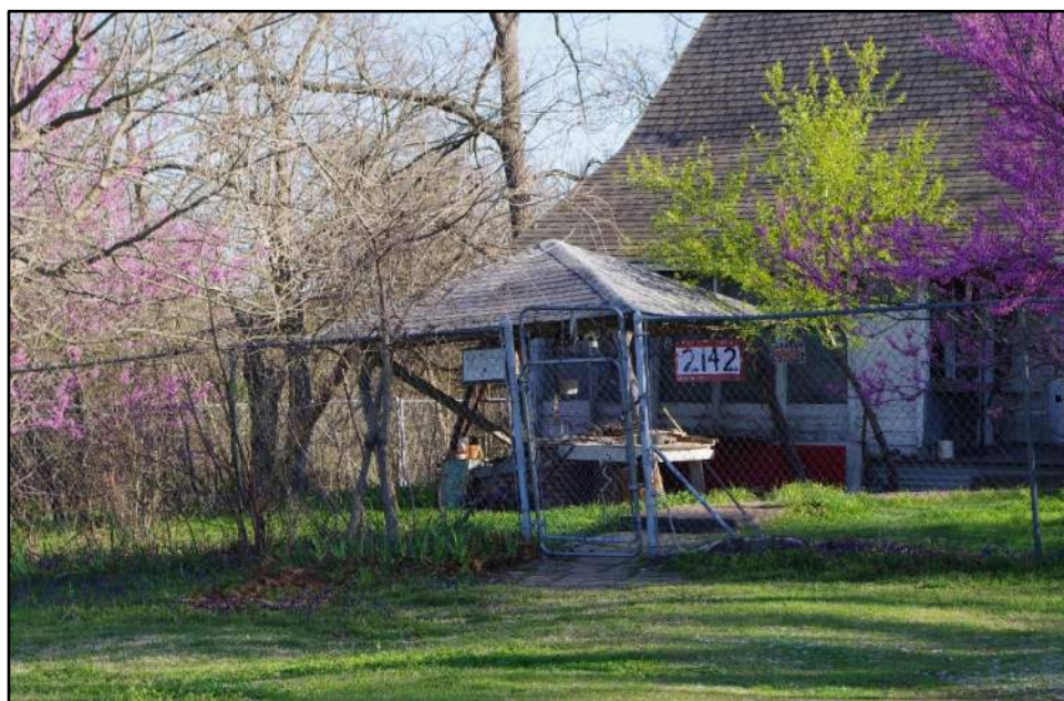
View of Resource 44f, camera facing southwest.
