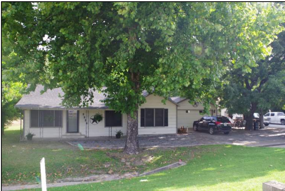
Photograph F-174: Overview of Resource 46, camera facing northeast.
