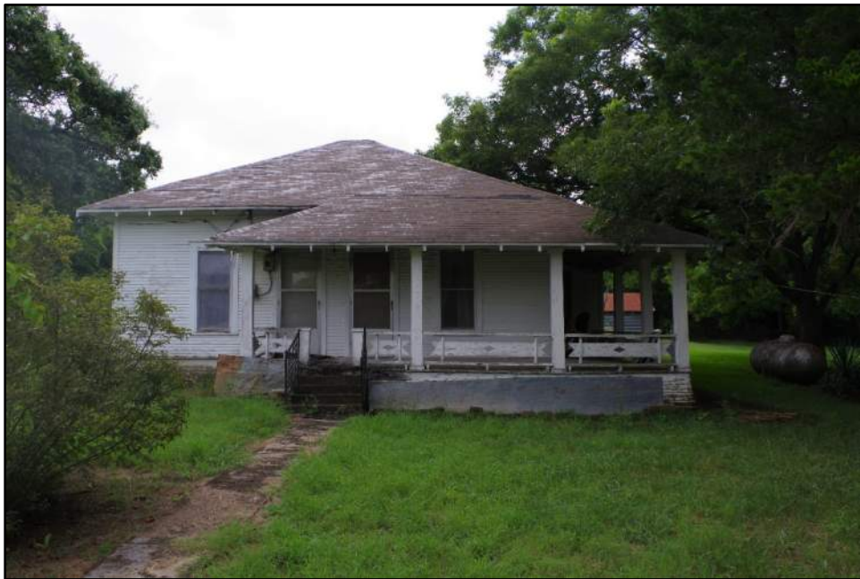
Photograph F-124: View of Resource 37a, camera facing north.
