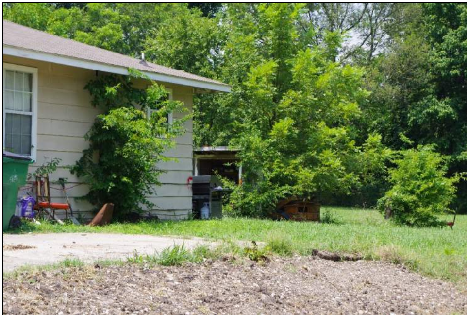
Photograph F-10: View of non-historic-age shed associated with Property 02, camera facing northwest.
