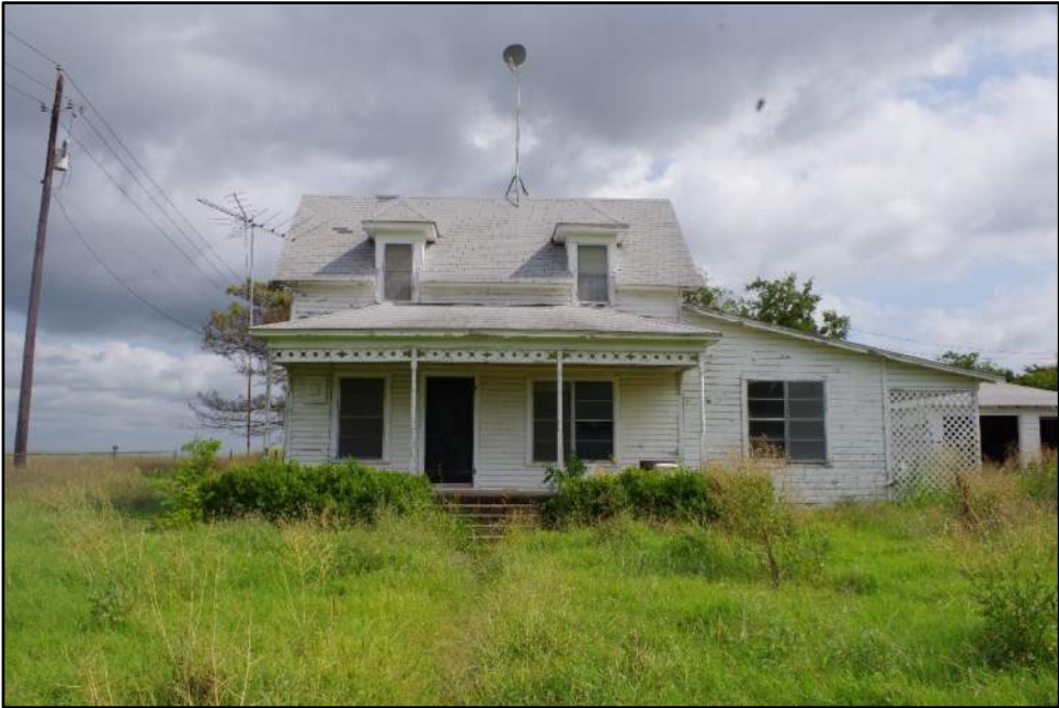
View of Resource 38a, camera facing north.
