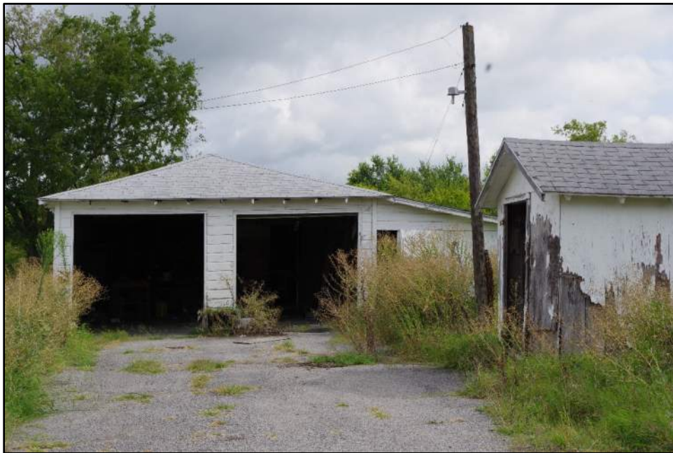
Photograph F-136: View of Resource 38b, camera facing north.
