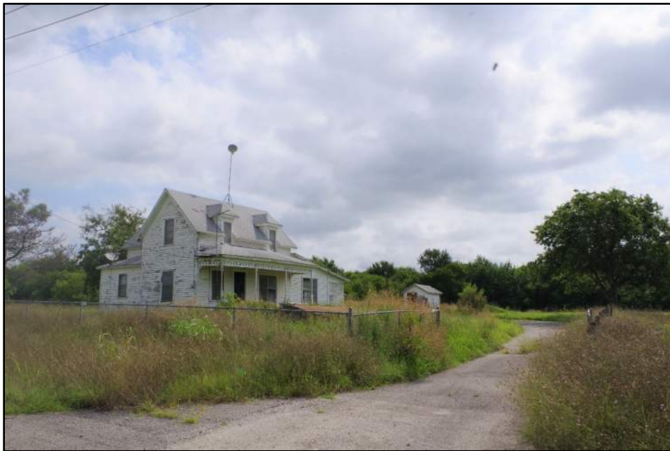
Photograph F-132: Overview of Resource 38, camera facing northeast.
