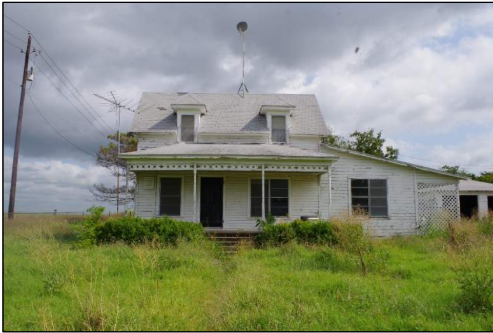
Photograph F-133: View of Resource 38a, camera facing north.
