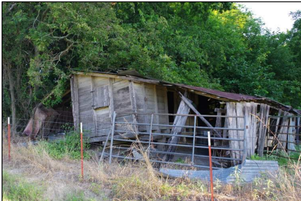
Photograph F-164: View of Resource 44d, camera facing northwest.
