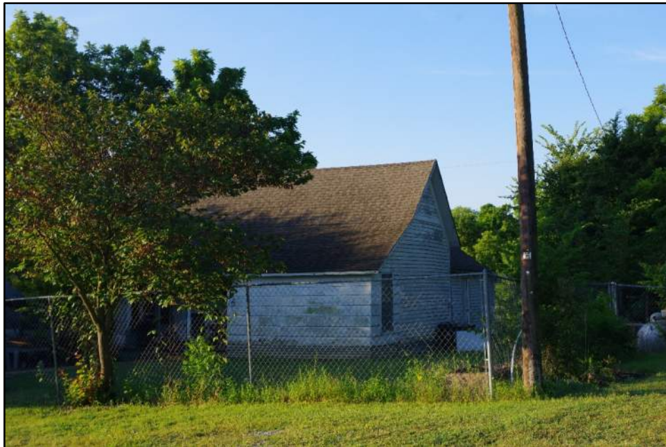
Photograph F-159: Obstructed view of Resource 44a, camera facing southeast.
