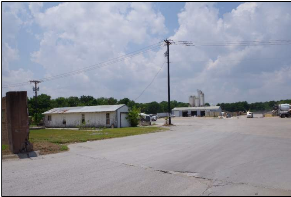
Photograph F-3: Overview of historic-age warehouses, camera facing northwest.
