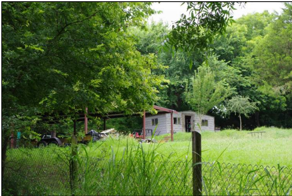
Photograph F-112: View of non-historic-age outbuildings associated with Resource 33, camera facing southwest.
