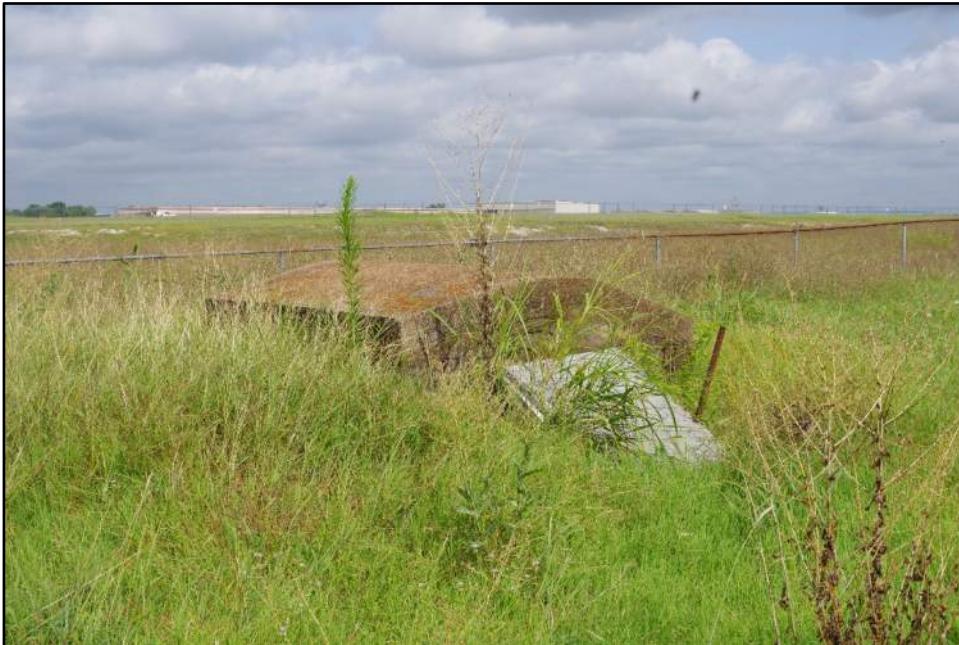
View of Resource 38e, camera facing west.
