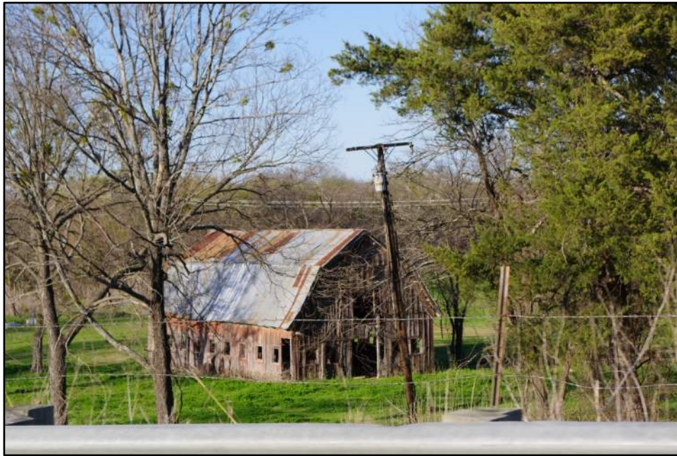
View of Resource 07a, camera facing northeast.
