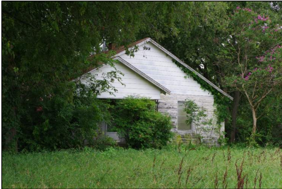
View of Resource 41a, camera facing south.
