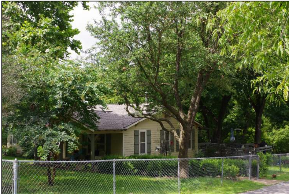
View of Resource 35a, camera facing southwest.
