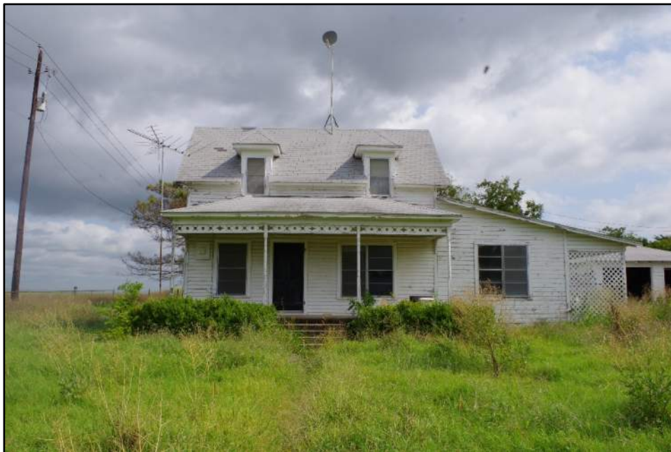
View of Resource 38a, camera facing north.
