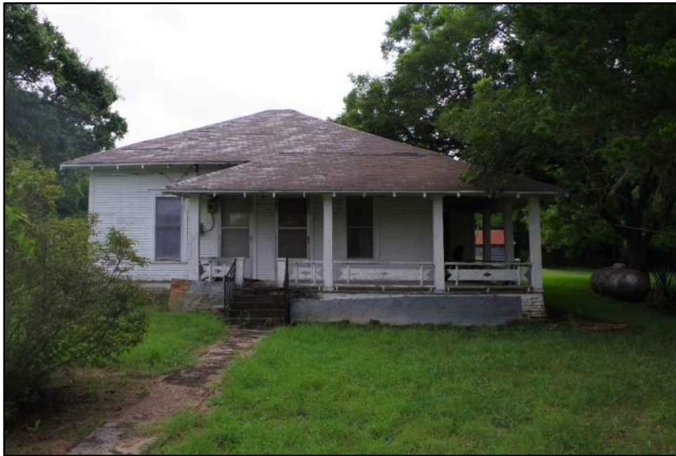
View of Resource 37a, camera facing north.
