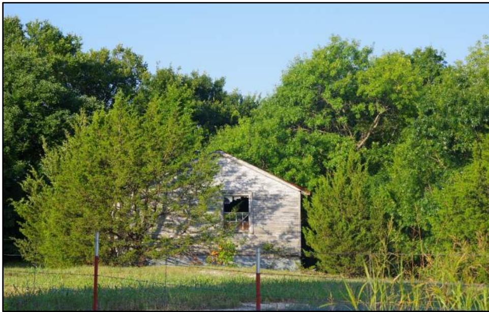
Photograph F-168: View of Resource 44g, camera facing southwest.
