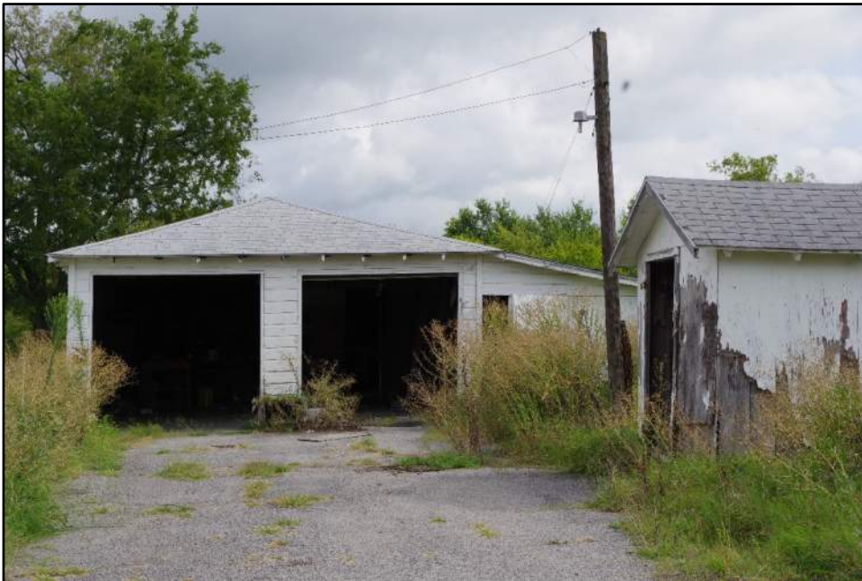
View of Resource 38b, camera facing north.
