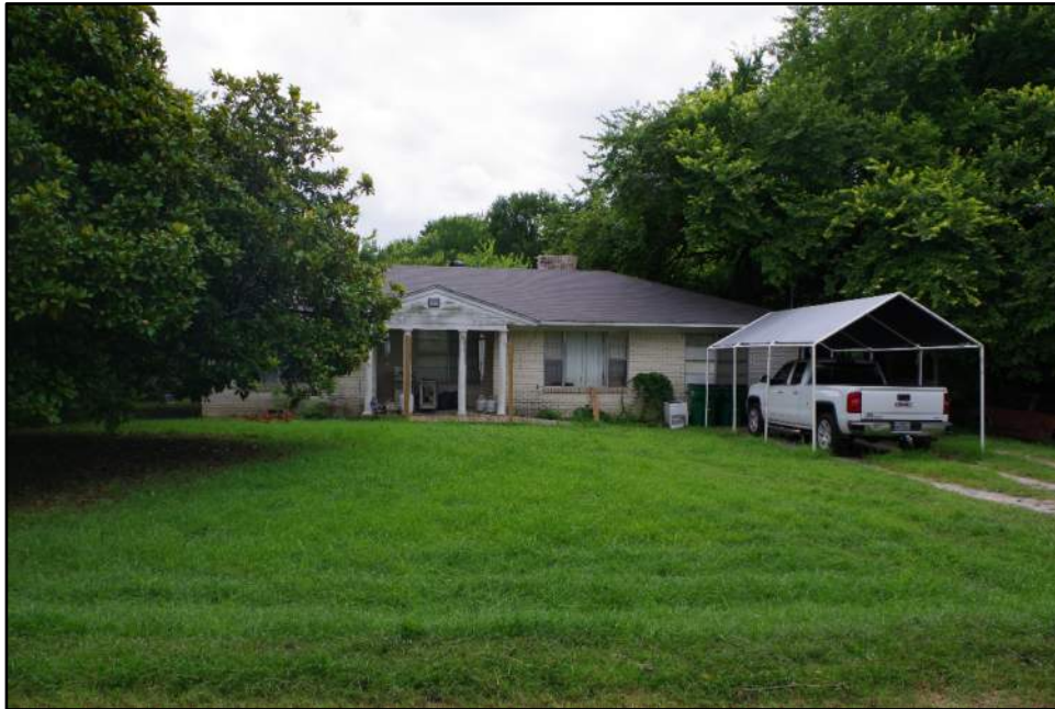
View of Resource 31a, camera facing south.
