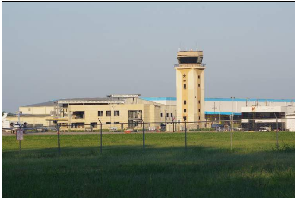
Photograph F-31: View of non-historic-age air control tower and terminal (McKinney National Airport) associated with Property 09, camera facing southwest.
