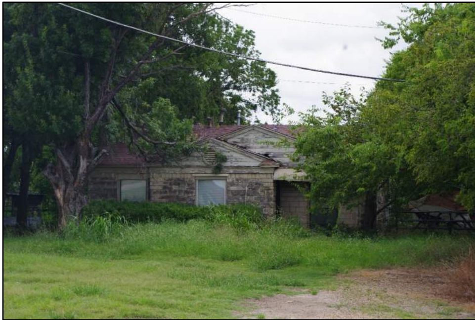
View of Resource 25, camera facing east.
