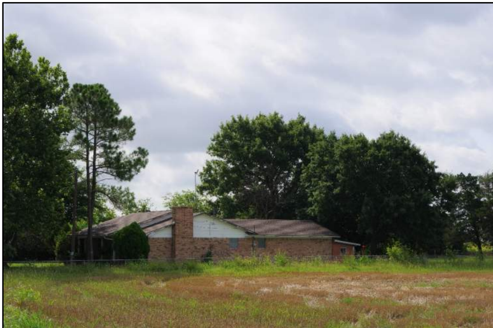
Photograph F-142: Overview of Property 39, camera facing southeast.
