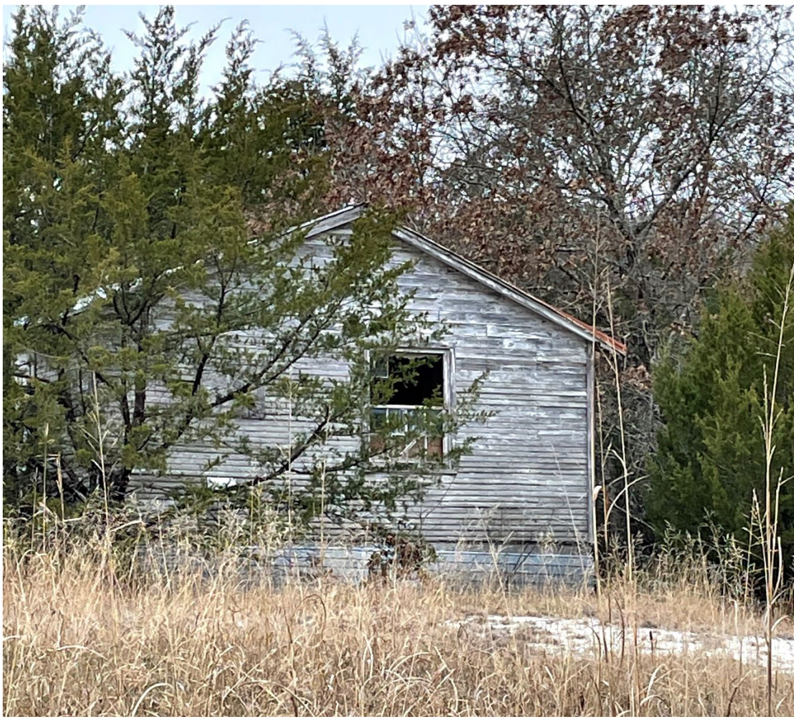
Resource 01f, historic age building in area of former Enloe School in APE on CR 722 looking south.
