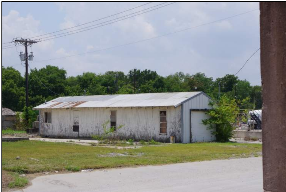
View of Resource 01a, camera facing southwest.
