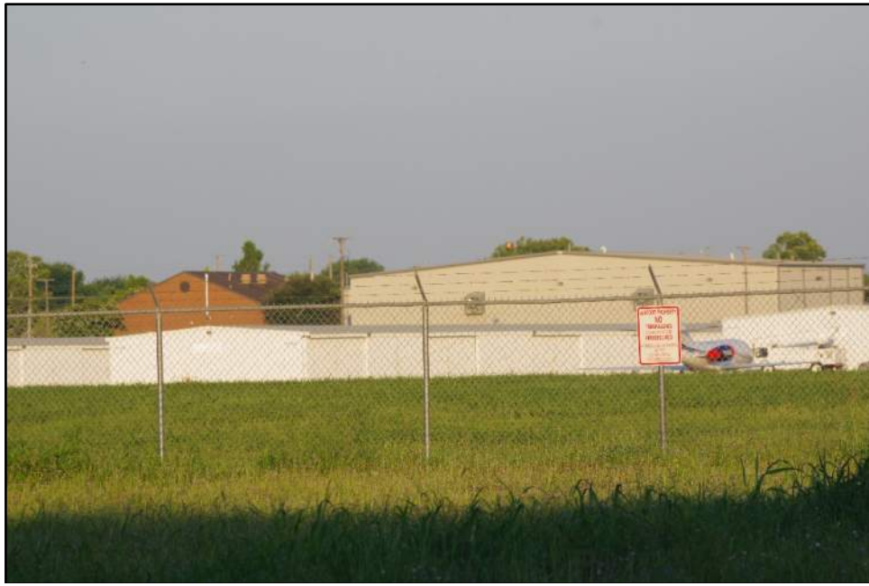
Photograph F-29: Obstructed view of Resource 09b, camera facing west.
