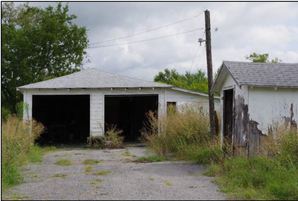
View of Resource 38b, camera facing north.
