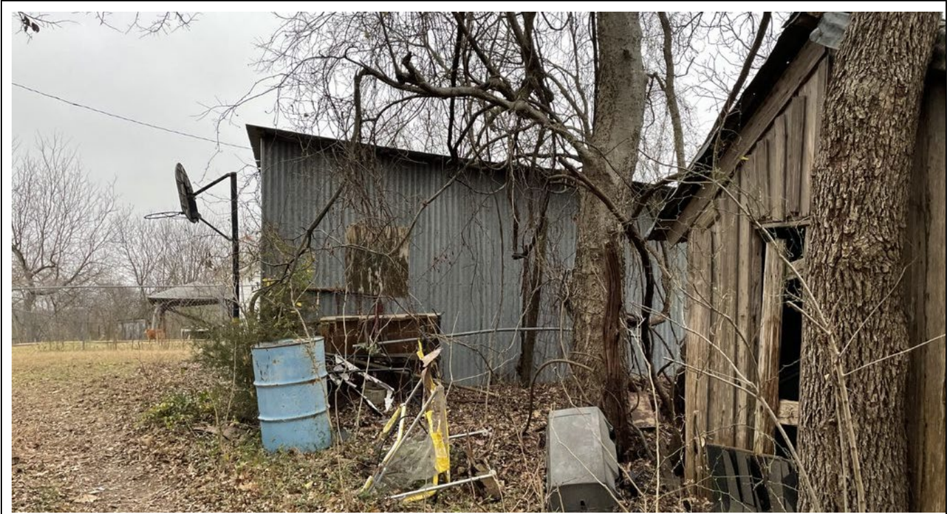
Resource 01b, storage building associated with Enloe Farm, looking east-southeast.
