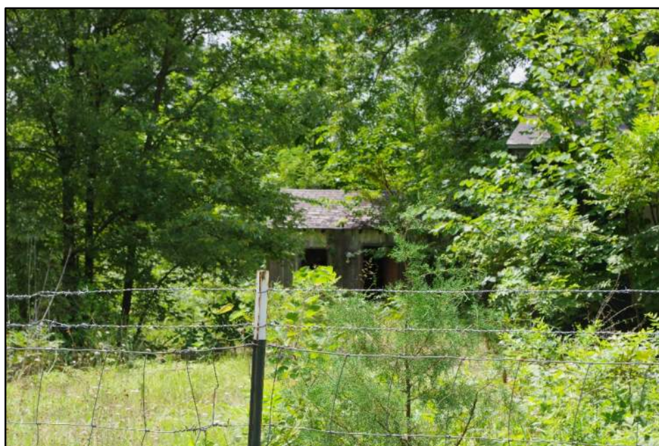
View of Resource 31c, camera facing south.
