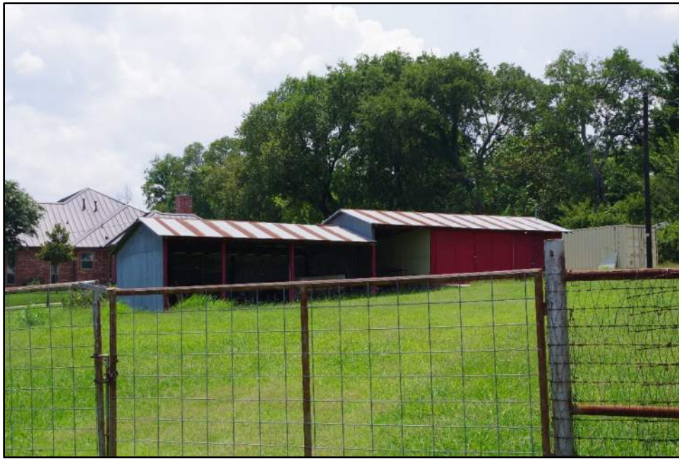
Photograph F-17: View of Resource 05, camera facing southwest.
