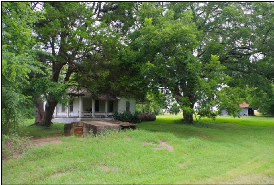
Photograph F-122: Overview of Resource 37, camera facing northwest.
