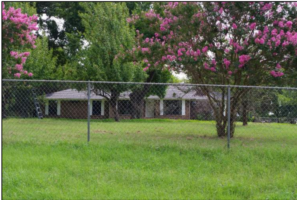
View of Resource 34, camera facing east.
