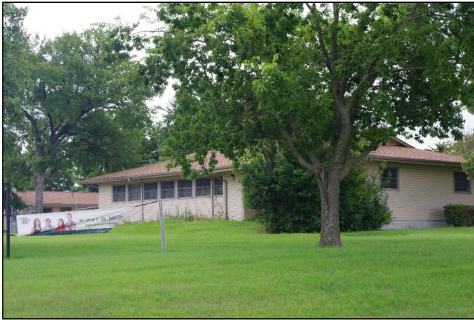
Photograph F-83: View of Resource 22b, camera facing southeast.
