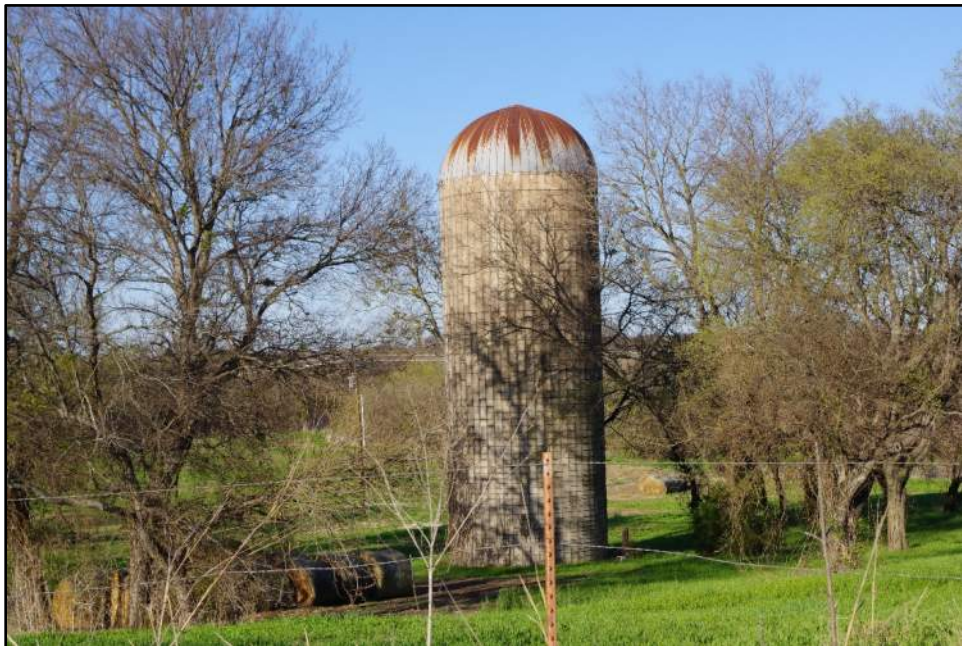
Photograph F-24: View of Resource 07b, camera facing north.
