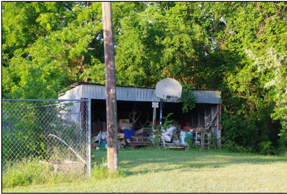
Photograph F-161: View of Resource 44b, camera facing southwest.
