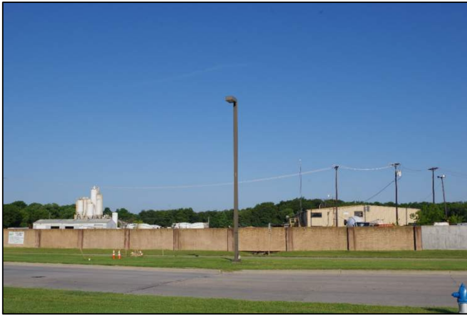
Photograph F-1: Overview of Resource 01, camera facing west.
