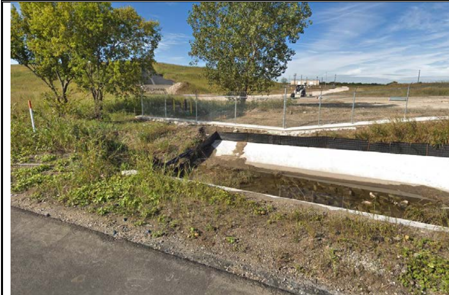
Photo 8. Representative photo of ephemeral stream Water Feature 20 (Google Street View October 2018). This stream functions like a ditch (only flowing as water sheds off the roadway); however, this feature appears to be a realignment of a natural ephemeral stream channel.
