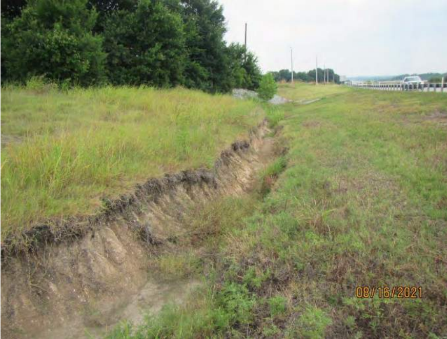
Photo 109. Photo of Ditch Drainage Feature- Water Feature 216 in the central portion of the Environmental Footprint. Water Feature 216 was constructed in uplands to aid in the removal of stormwater runoff from US 75. Note the presence of erosion here. Photo was taken to the west on August 16, 2021.
