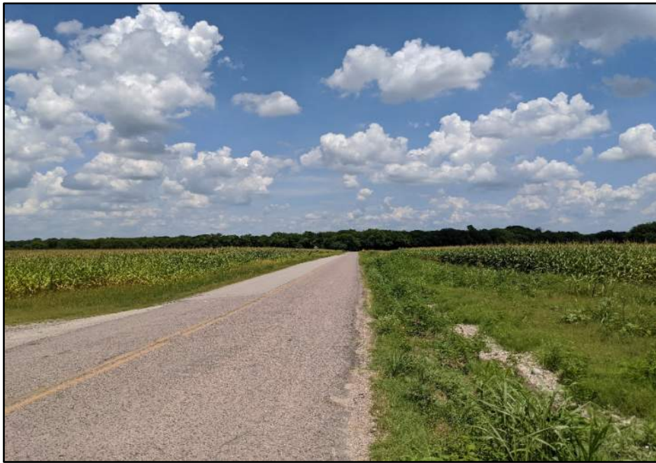
Photograph 5: Representative view of the Urban Low Intensity vegetation type observed within the project area. The Row Crops vegetation type occurs on either side of the road.
