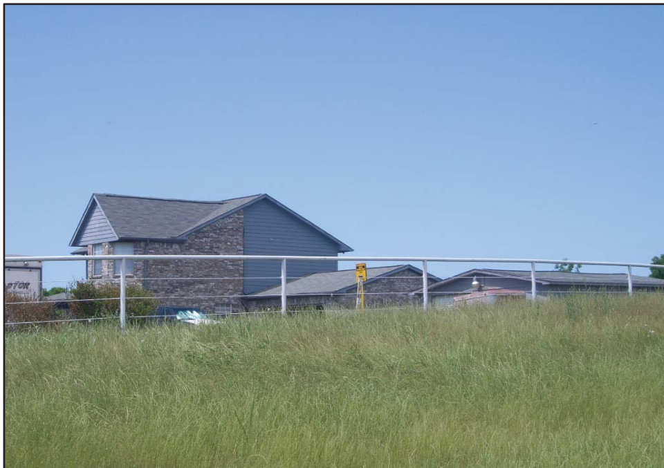
Photo 46: View looking southwest toward a natural gas pipeline marker along Fishtrap Road just west of US 377. Date of Photo: 5/6/20.
