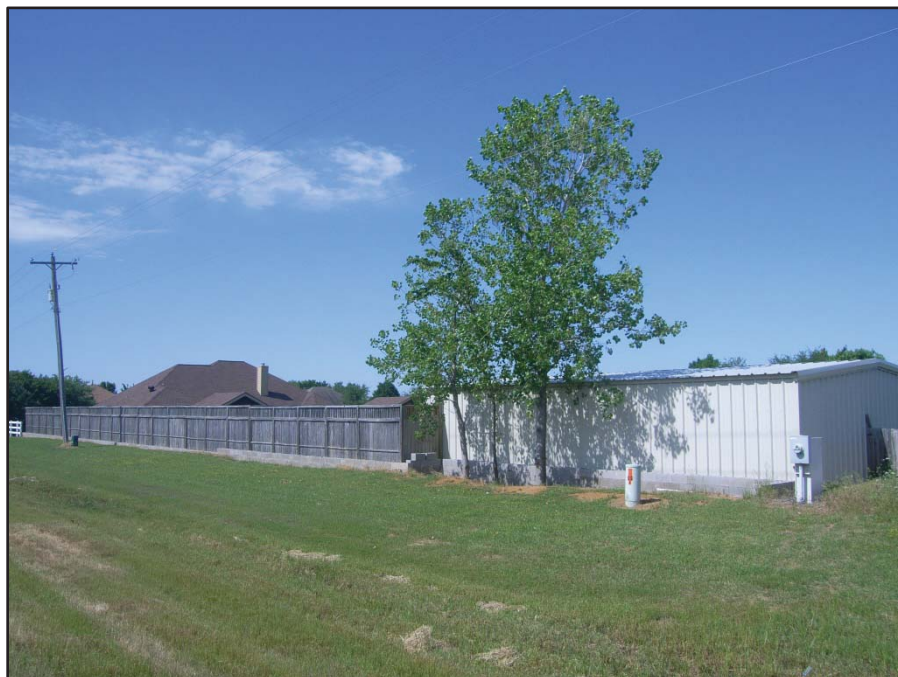
Photo 28: View looking southwest from US 377 toward a metal shed, and two other storage buildings, potential displacements (Disp. 11) at 855 Sherry Ln S, Krugerville, TX 76227. Date of Photo: 5/6/20
