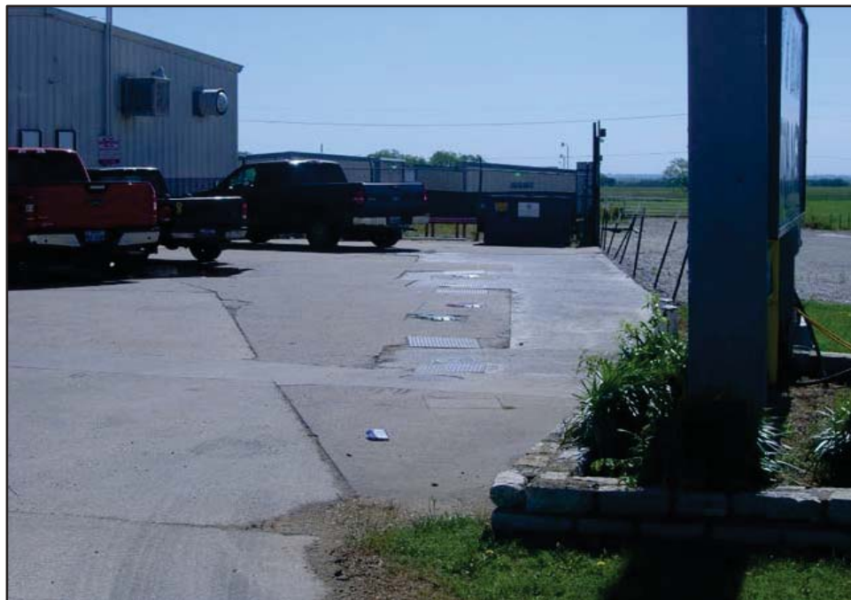
Photo 36: View looking southeast towards the tank hold of the Sunny Mart LPST and PST site at 1293 S. US 377, Ste. 100, Pilot Point, TX 76258 (HazMat Site 11). Date of Photo: 4/29/20.
