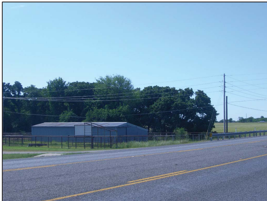
Photo 21: View looking southeast from US 377 toward a metal barn that is a potential displacement (Disp. 3) at 1311 S US 377, Pilot Point, TX 76258. Date of Photo: 5/6/20
