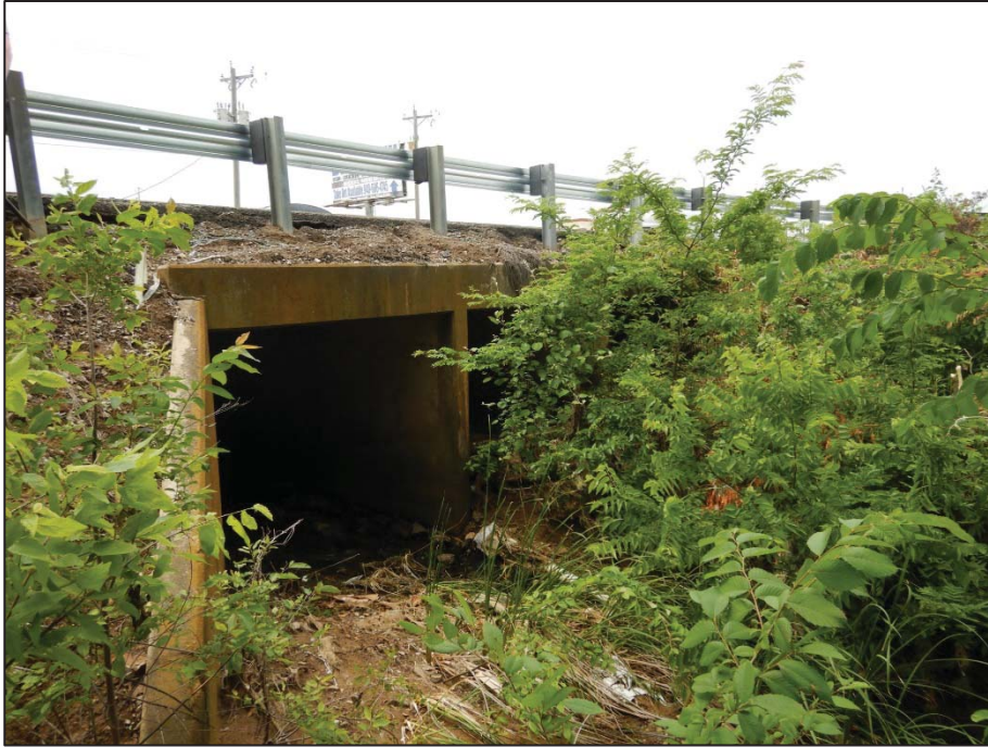
Photo 91: View looking west toward Crossing 13 – Running Branch (US 377 northbound side).
