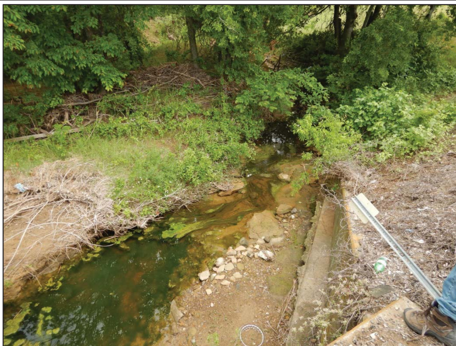
Photo 96: View looking southeast toward Crossing 14 – tributary to Pecan Creek (US 377 northbound side).
