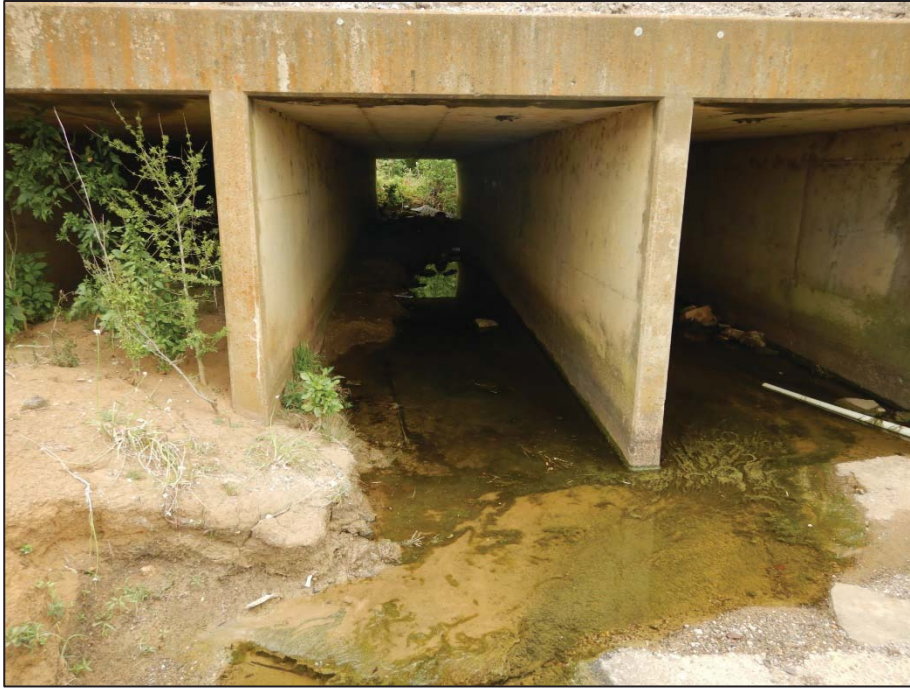
Photo 89: View looking east toward Crossing 13 – Running Branch (US 377 southbound side).
