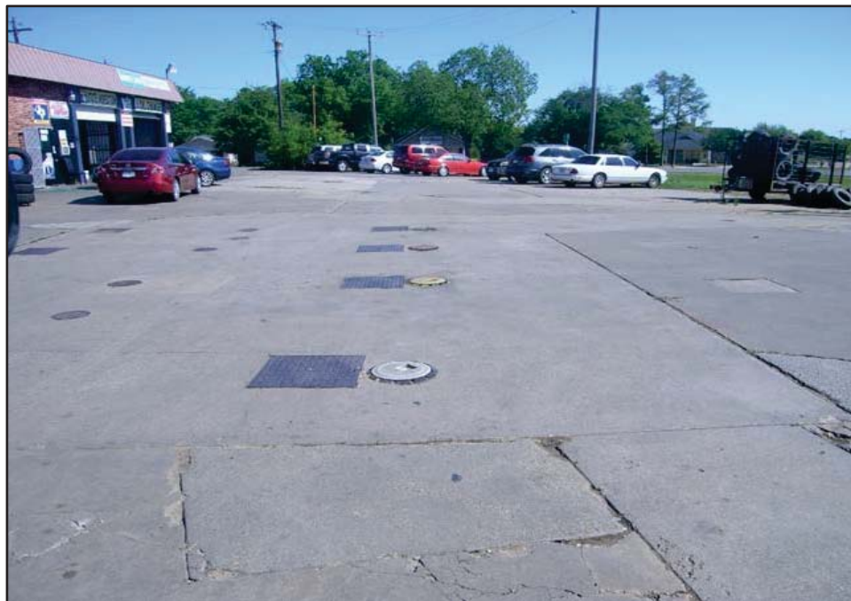
Photo 42: View looking north towards the tank hold of the Chaparral Plaza LPST and PST site at 704 S. US 377, Aubrey, TX 76227 (HazMat Site 28). Date of Photo: 4/29/20.
