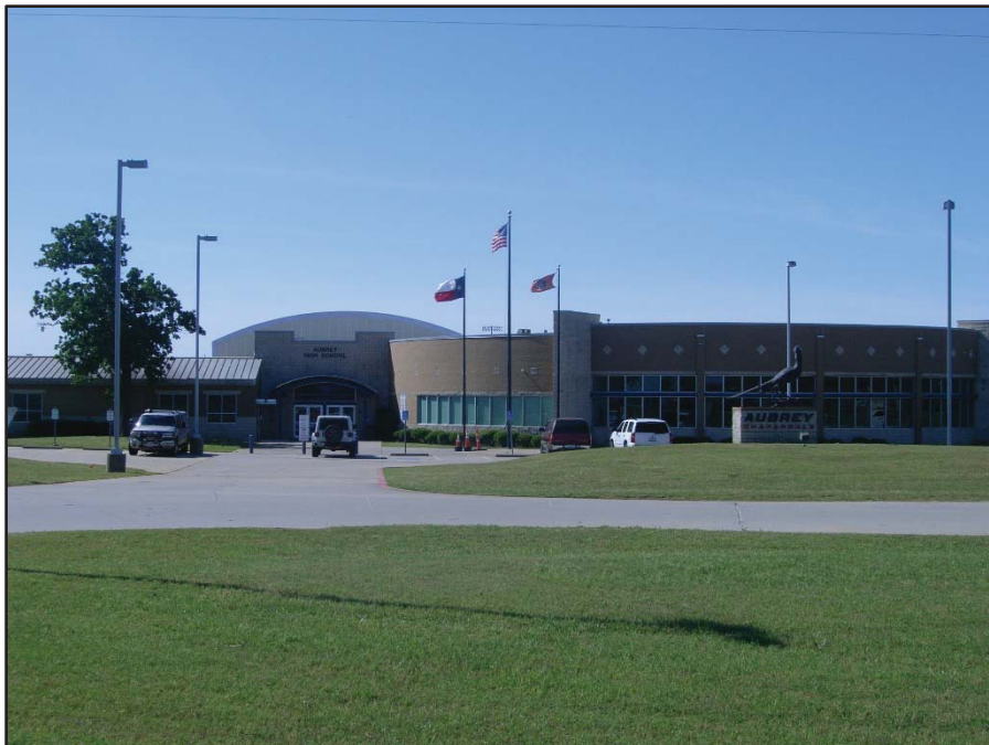
Photo 10: View looking south from Spring Hill Rd towards Aubrey High School (ID 54) at 510 Spring Hill Rd, Aubrey, TX 76227. Date of Photo: 4/29/20.
