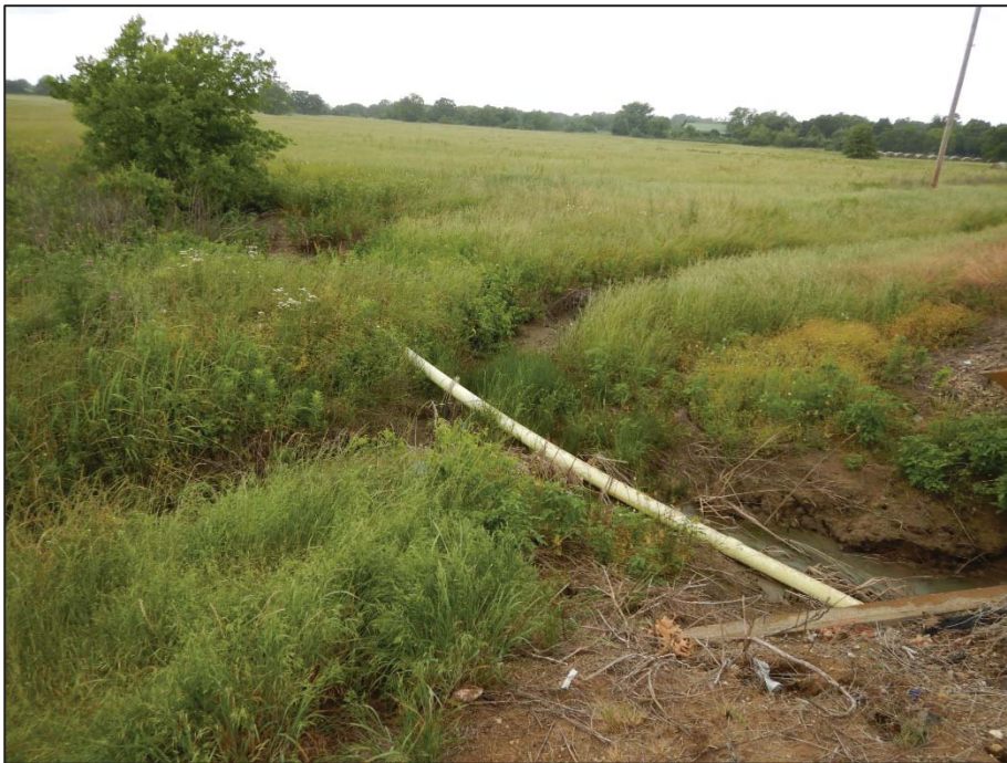
Photo 100: View looking west toward Crossing 16 – tributary to Cantrell Slough (US 377 southbound side).
