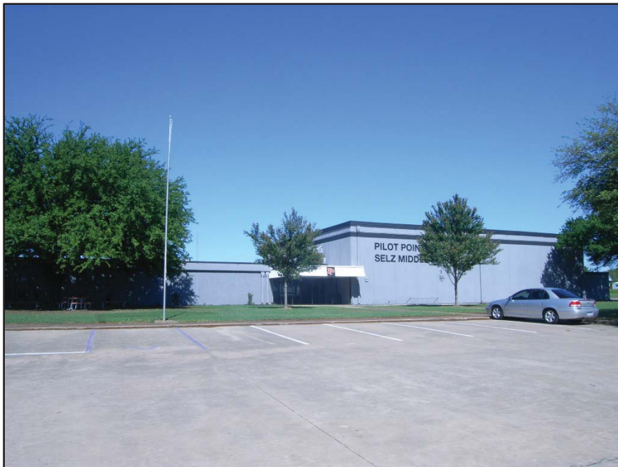
Photo 2: View looking west from S Harrison St towards Pilot Point Middle School (ID 29) at 828 S Harrison St, Pilot Point, TX 76258. Date of Photo: 4/29/20.
