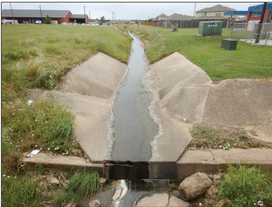
Photo 90: View looking west toward Crossing 13 – Running Branch (US 377 southbound side).
