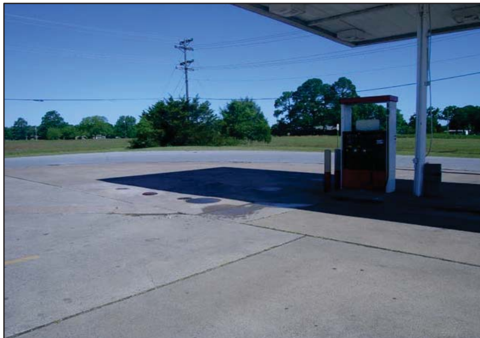
Photo 38: View looking northwest towards the tank hold of the Edgar's Shell LPST and PST site at 100 N. US 377, Krugerville, TX 76227 (HazMat Site 16). Date of Photo: 4/29/20.
