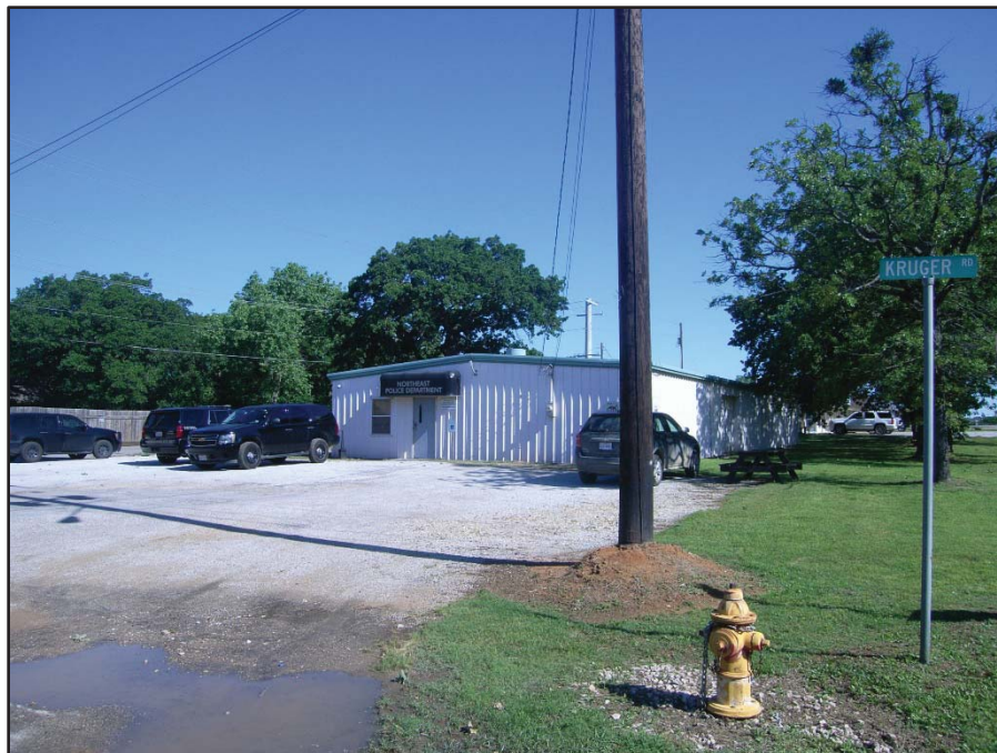
Photo 15: View looking northwest along Kruger Rd toward the Northeast Police Department (ID 65) at 100 Kruger Rd, Krugerville, TX 76227. Date of Photo: 4/29/20
