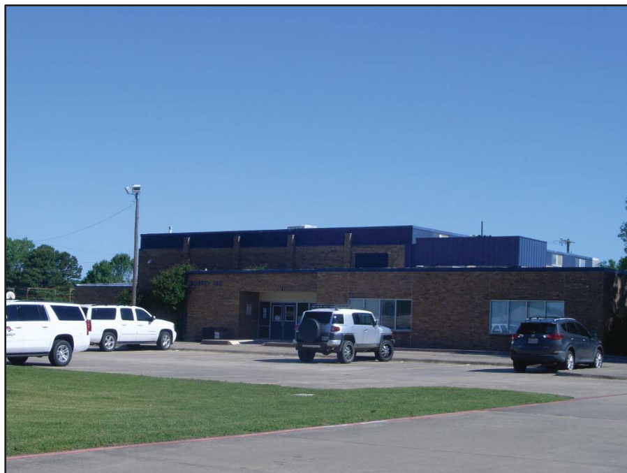
Photo 8: View looking west from a parking lot off US 377 towards the Early Bird Learning Center (ID 41) at 415 Tisdell Ln, Aubrey, TX 76227. Date of Photo: 4/29/20.
