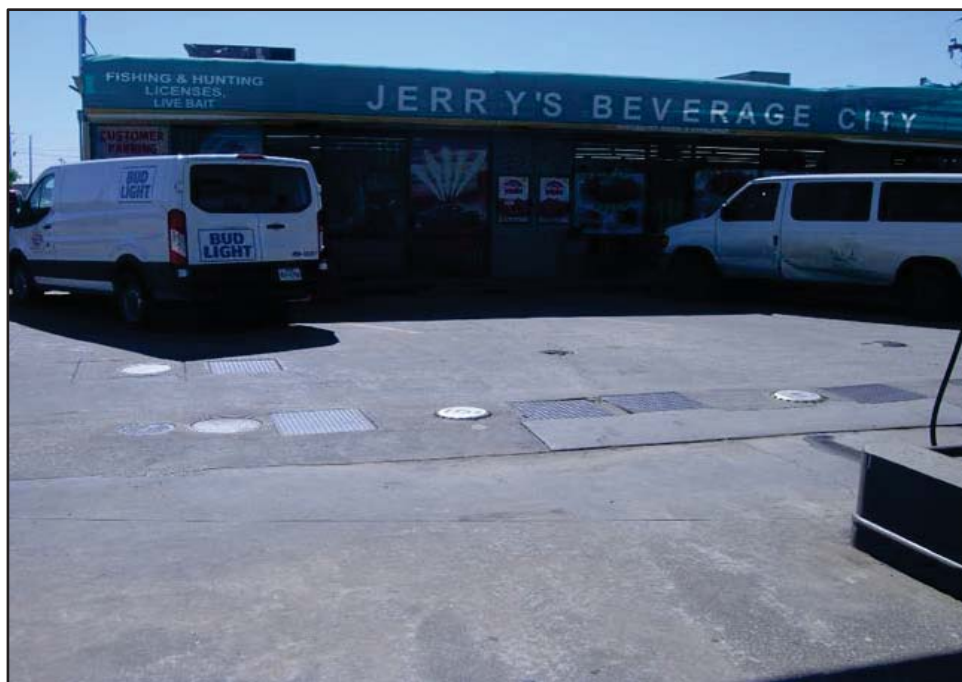
Photo 37: View looking east towards the tank hold of the Jerry's Beverage City LPST and PST site at 1225 N. US 377, Pilot Point, TX 76258 (HazMat Site 12). Date of Photo: 4/29/20.
