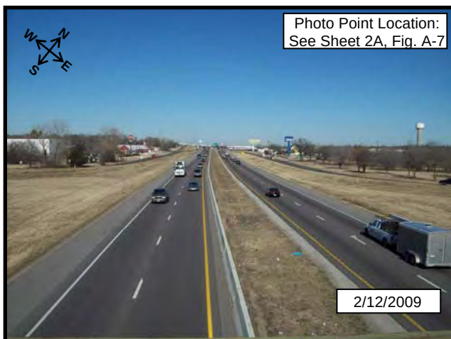
Photograph 3. Representative roadway configuration of existing IH 35E mainlanes, taken at Post Oak Drive.
