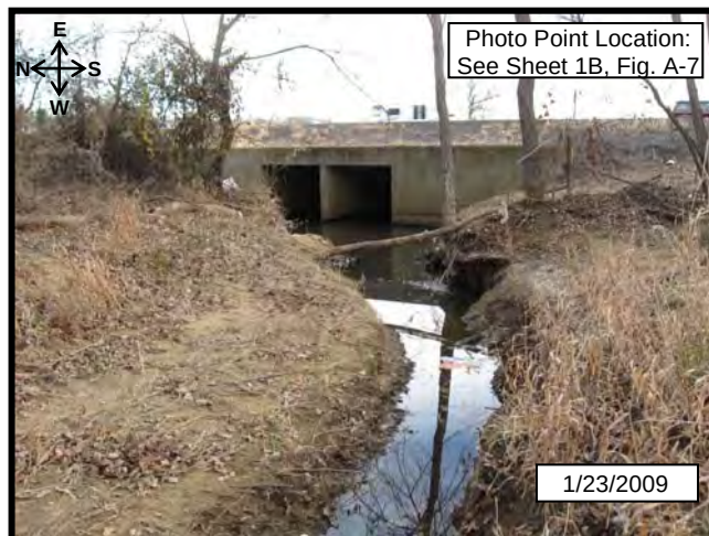
Photograph 8. View of same channel in Photograph 7, looking toward IH 35E showing cross drainage via box culverts, which is typical throughout project area.
