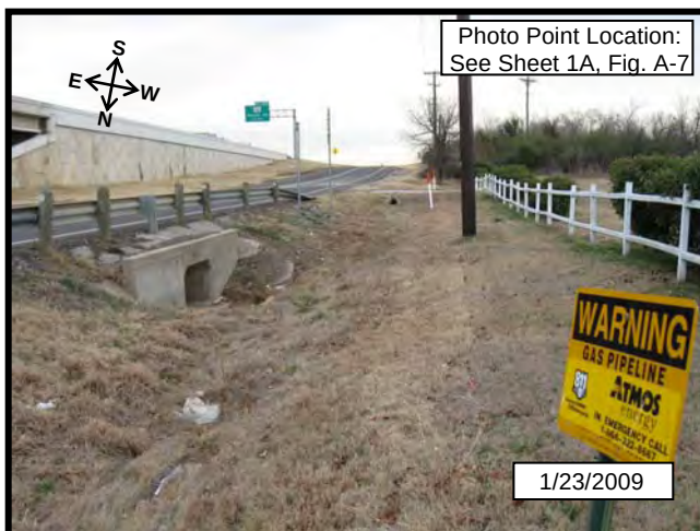
Photograph 9. Drainage culvert on west side of IH 35E that receives storm water from bar ditch runoff but has no defined channel that extends westward (Site W-1).
