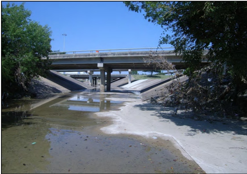
Photograph 18: Representative photograph of a concrete lined channel flowing under bridged section of US 80. View is to the north-northeast. (9/14/2017)
