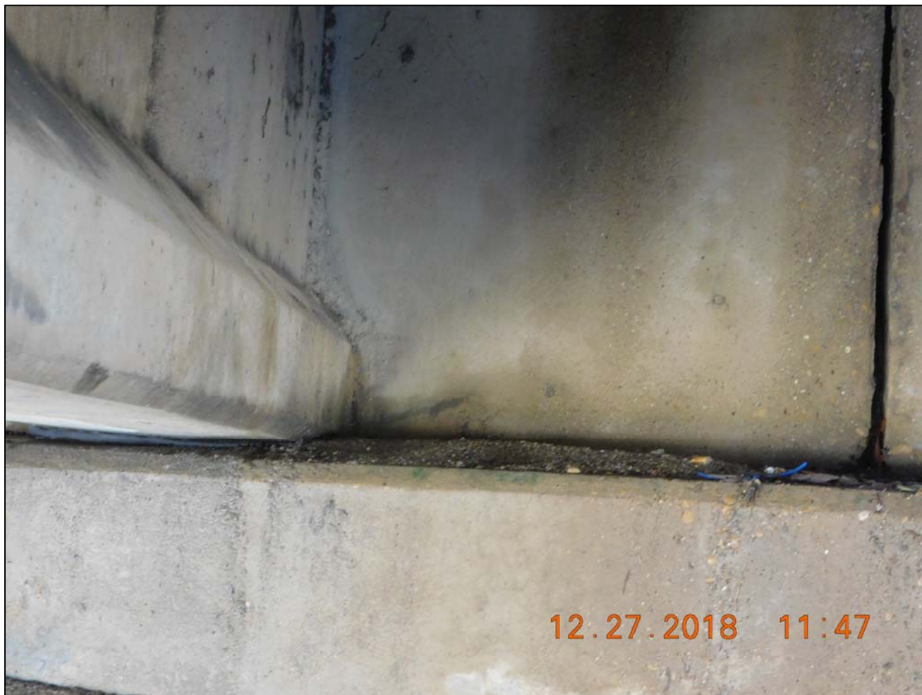
Photos 3: View of bulging neoprene bearing pad.
