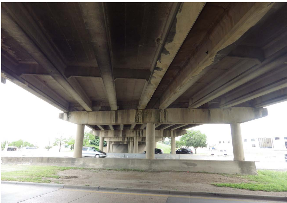
Underside of bridges showing how existing piers limit required widening of US 80.
