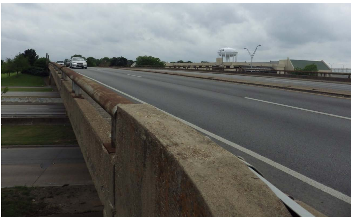
View showing insufficient bridge width.
