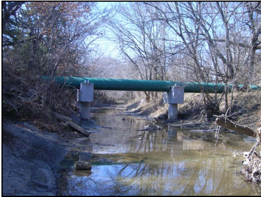
Photo 13: View looking west-northwest and upstream along Wilson Creek from the west side of FM 2478 near Sta. 410+00. The blue pipe is off proposed ROW and consists of a 24-inch sanitary sewer line.
