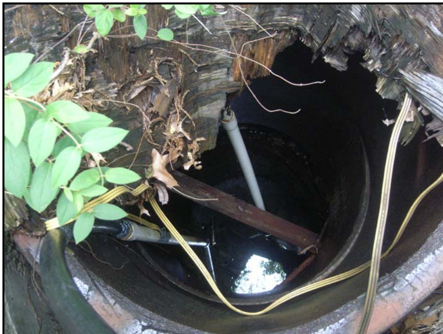
Photo 24: View looking into the water well on the east side of FM 2478 near Sta. 396+50. The total depth of the well from the top of the structure is approximately 13 feet and the water table in the well is approximately 7-1/2 feet below the top of the structure. The well is used for irrigation.
