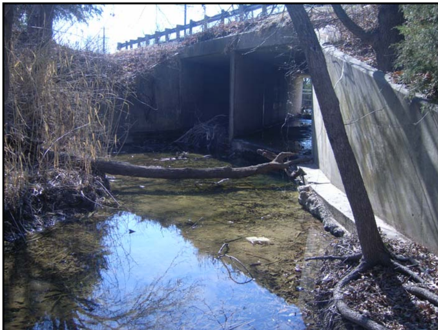
Photo 10: View looking southwest and upstream along Rutherford Branch toward the Horn Branch bridge from east of FM 2478 near Sta. 388+00. This bridge class culvert would be demolished and replaced as a part of the proposed project.
