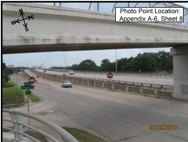
Photograph 29. IH 45 and Lenway, taken from the pedestrian bridge ramp on the southbound frontage road, looking northeast
