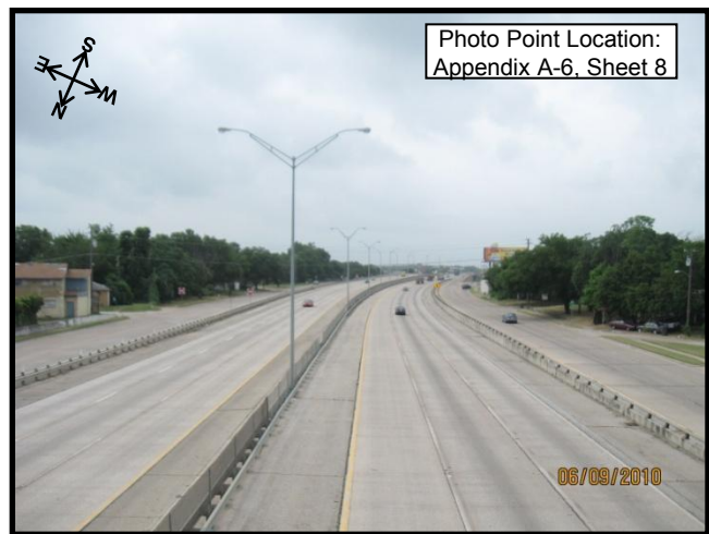
Photograph 32. IH 45 and Lenway, taken from the pedestrian bridge, looking south on IH 45
