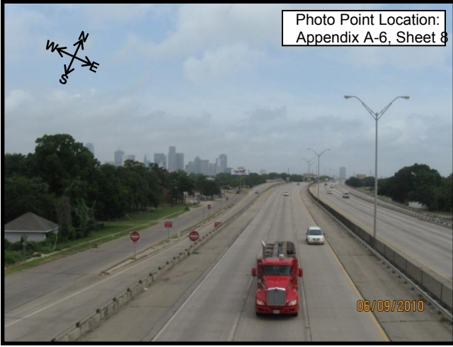
Photograph 31. IH 45 and Lenway, taken from the pedestrian bridge, looking north on IH 45
