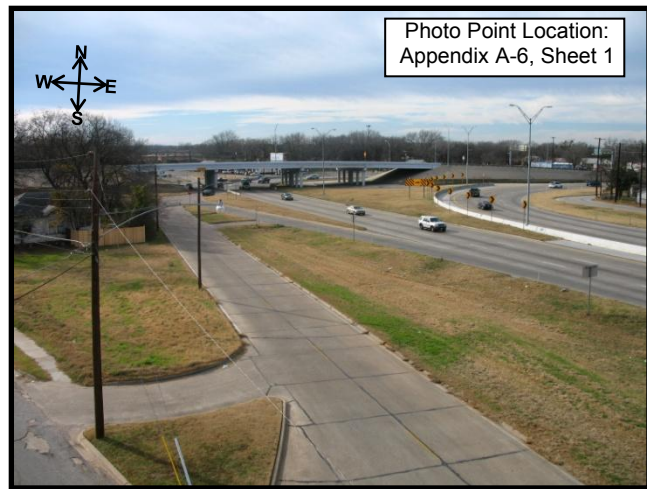
Photograph 20. 310-175, SE Corner – looking north.
