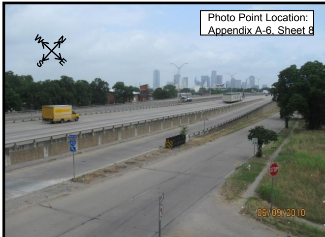
Photograph 35. IH 45 and Lenway, from the pedestrian bridge ramp on the northbound frontage road, looking northwest
