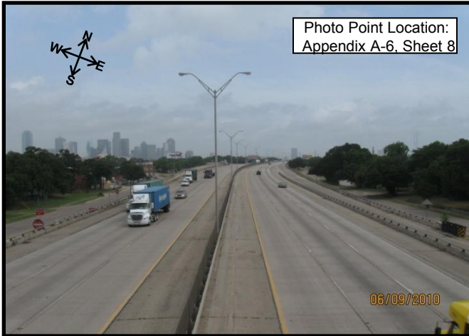
Photograph 33. IH 45 and Lenway, from the pedestrian bridge, looking north on IH 45
