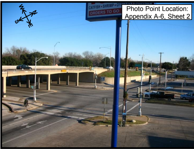
Photograph 19. 175 and Hatcher Street, NW Corner
