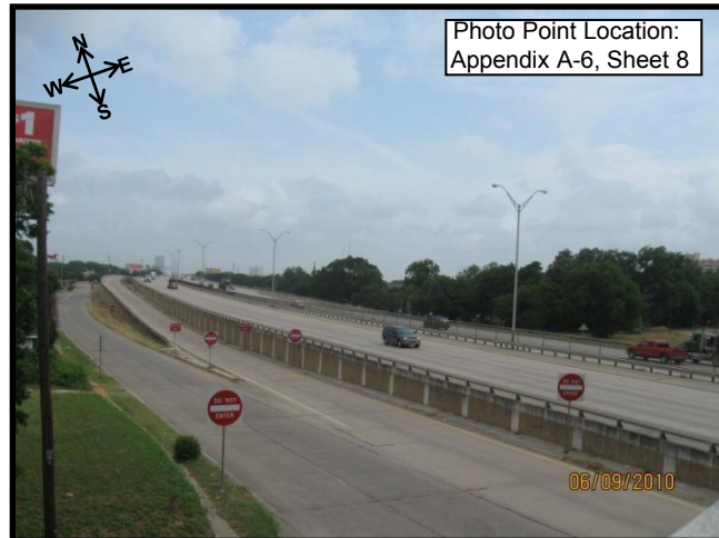
Photograph 30. IH 45 and Lenway, taken from the pedestrian bridge ramp on the southbound frontage road, looking northeast
