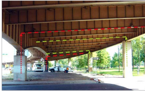
Photos show main girders with unsymmetric column supports.
