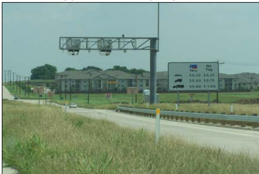
FIGURE 4-2: RAMP TOLL GANTRY
