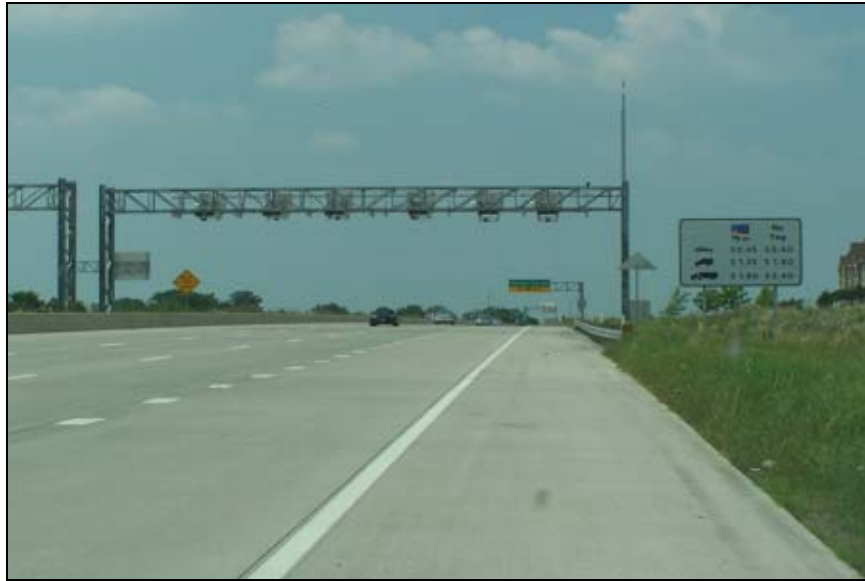
FIGURE 4-1: MAINLANE TOLL GANTRY
